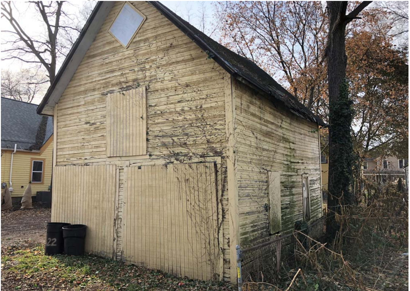
Photo showing building after vegetation has been removed.
