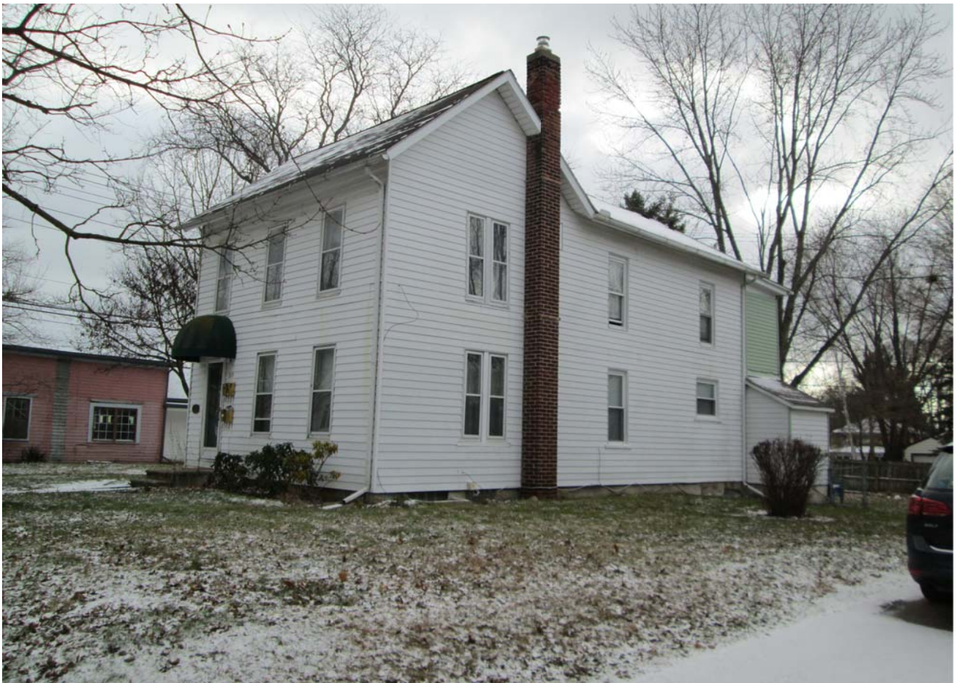
Facing southeast to facade and west elevation
