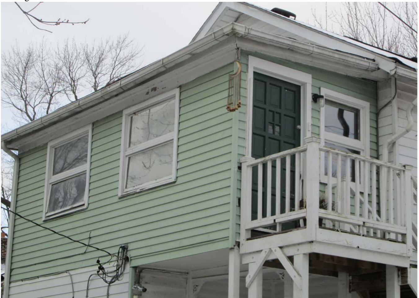
Detail of windows to be replaced.
