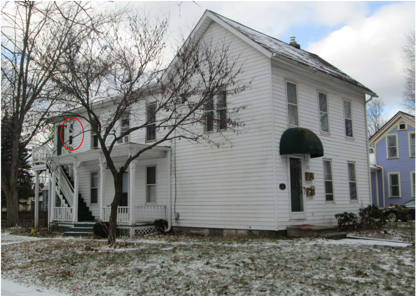
Facing southwest to facade and east elevation
