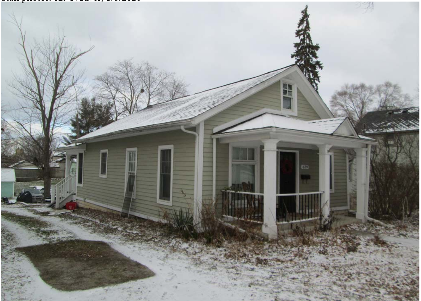
Facing northwest to facade and south elevation.
