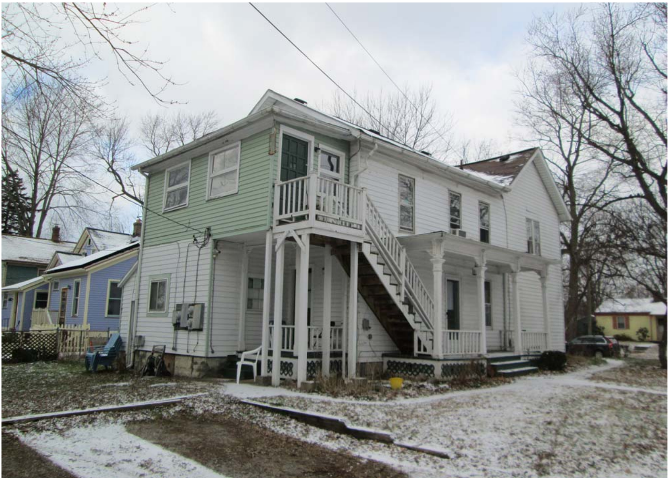
Facing northwest to east and south elevations
