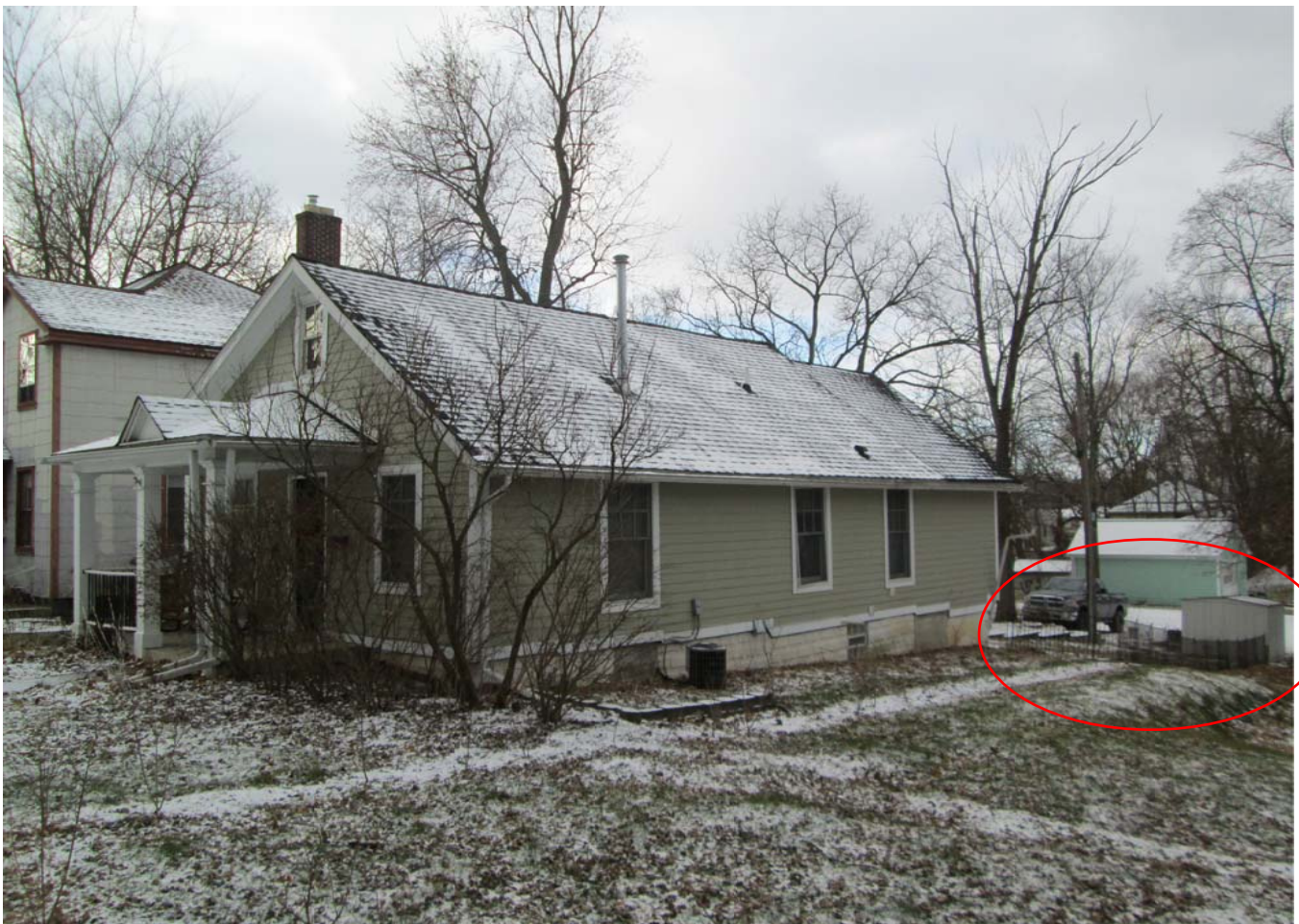
Facing southwest to facade and north elevation- fence and shed at right.
