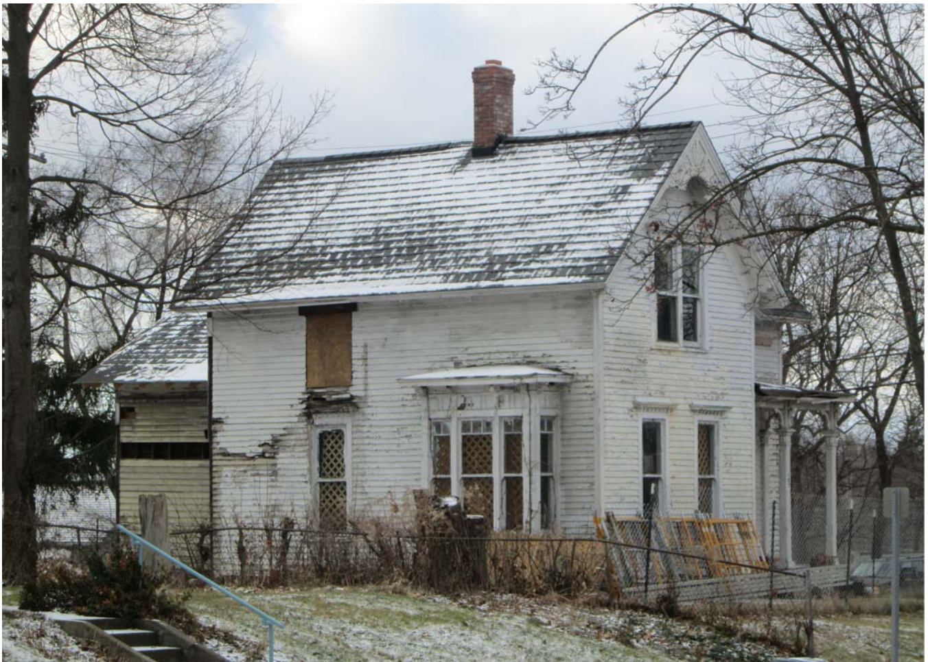
Facing southwest to facade and east elevation.
