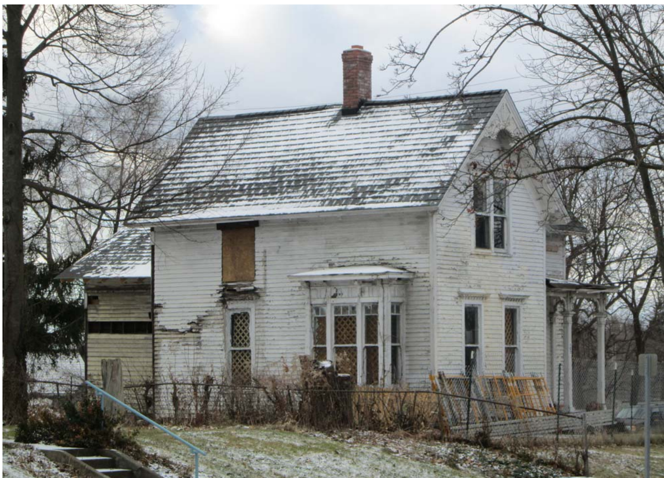
Facing southwest to facade and east elevation.
