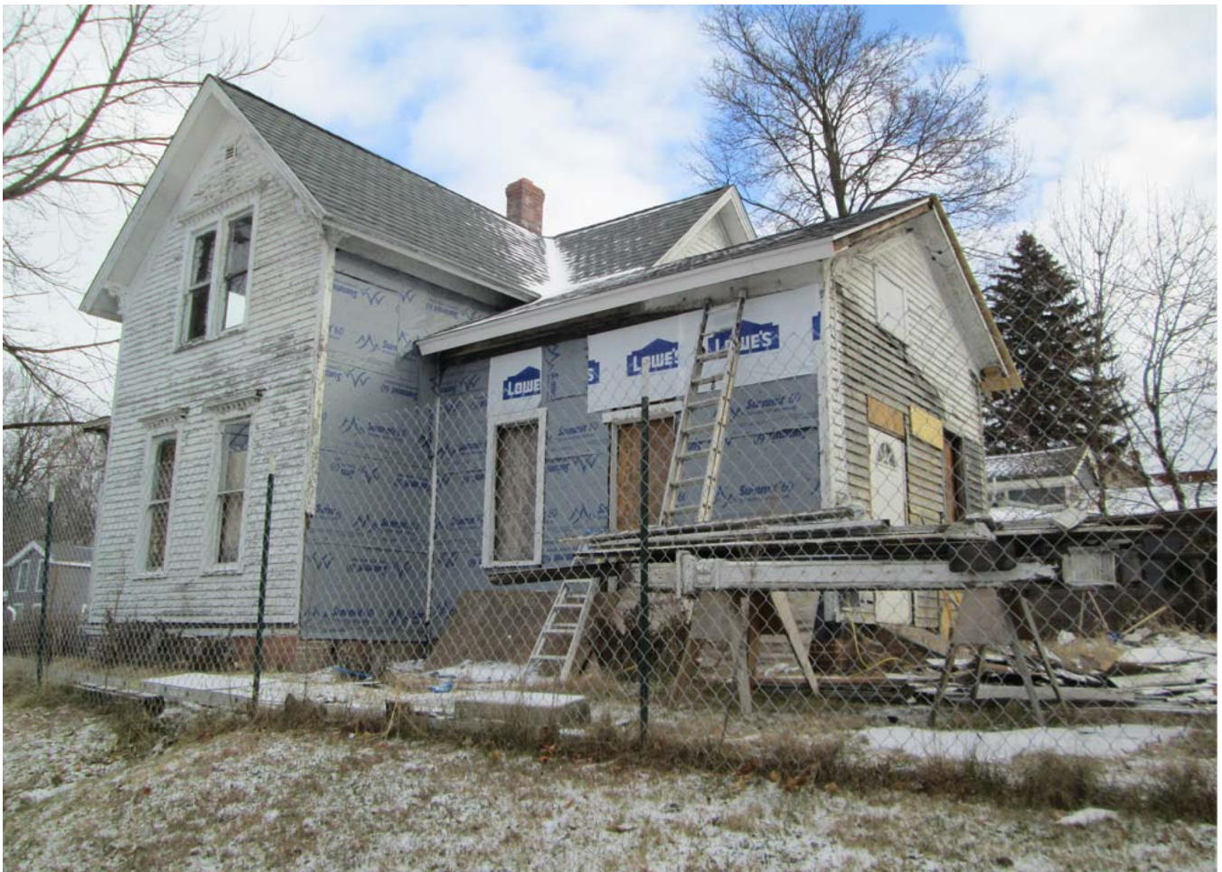
Facing northeast to west and south elevations.
