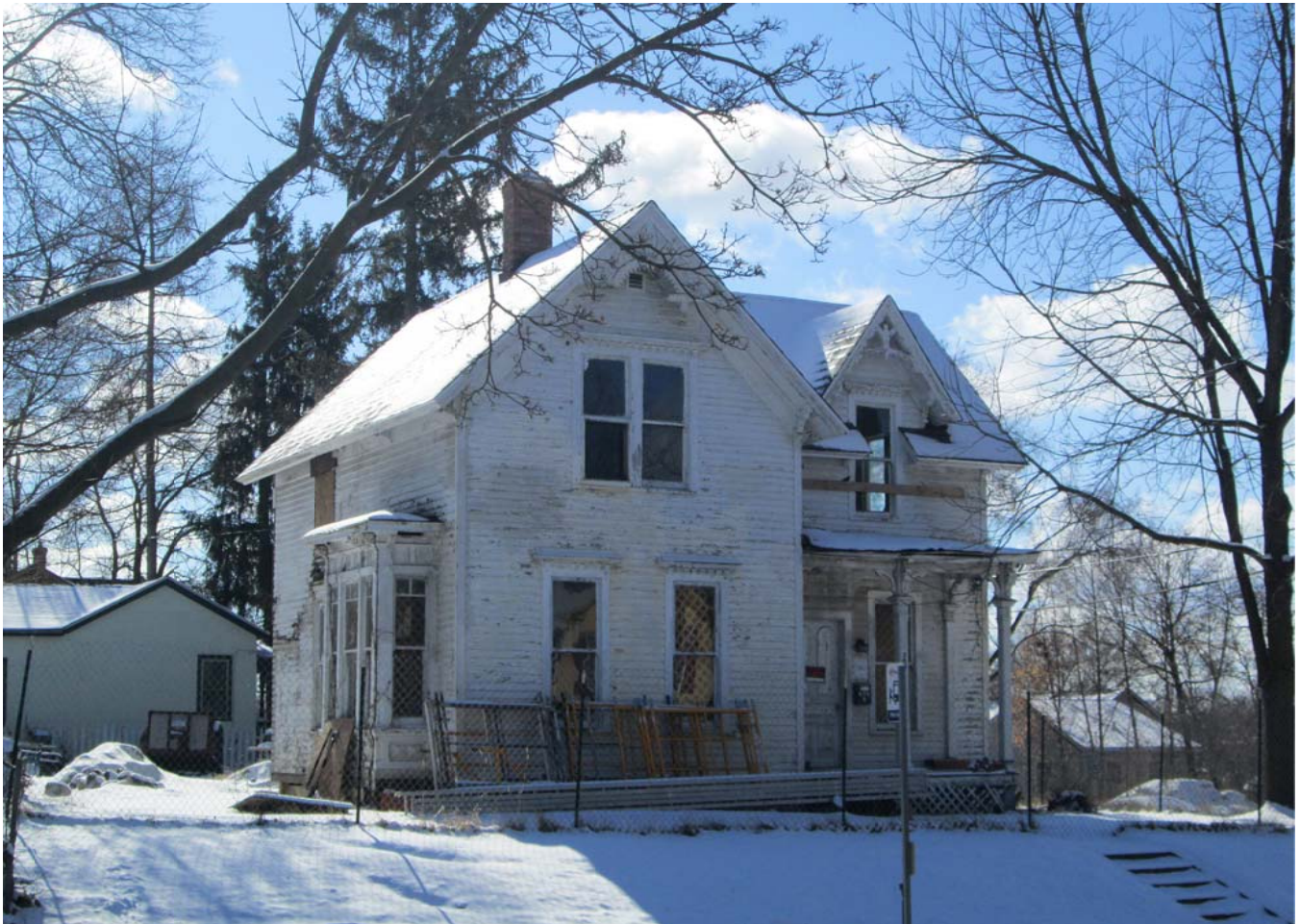
Facing southwest to facade and east elevation
