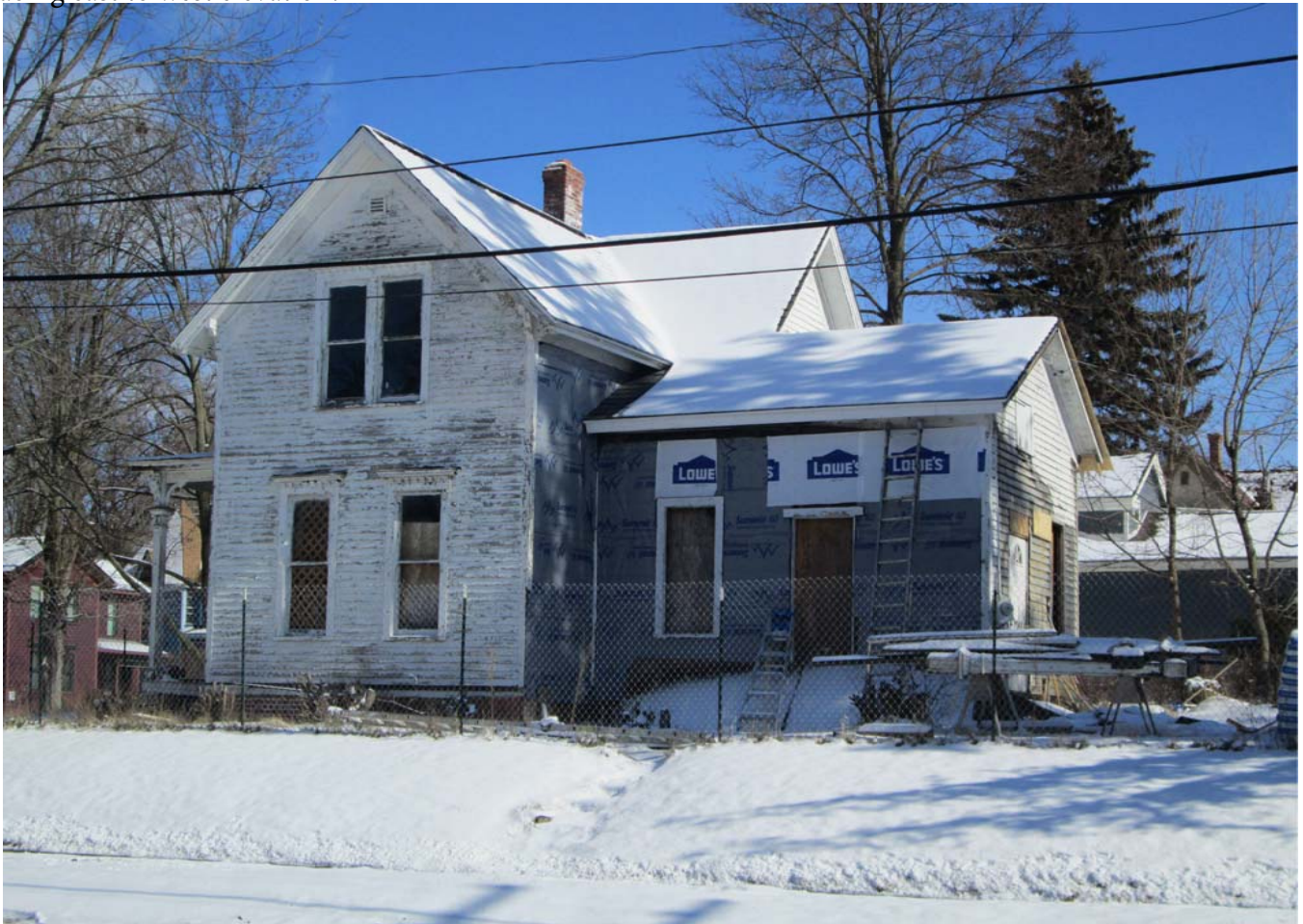
Facing northeast to west and south elevations.
