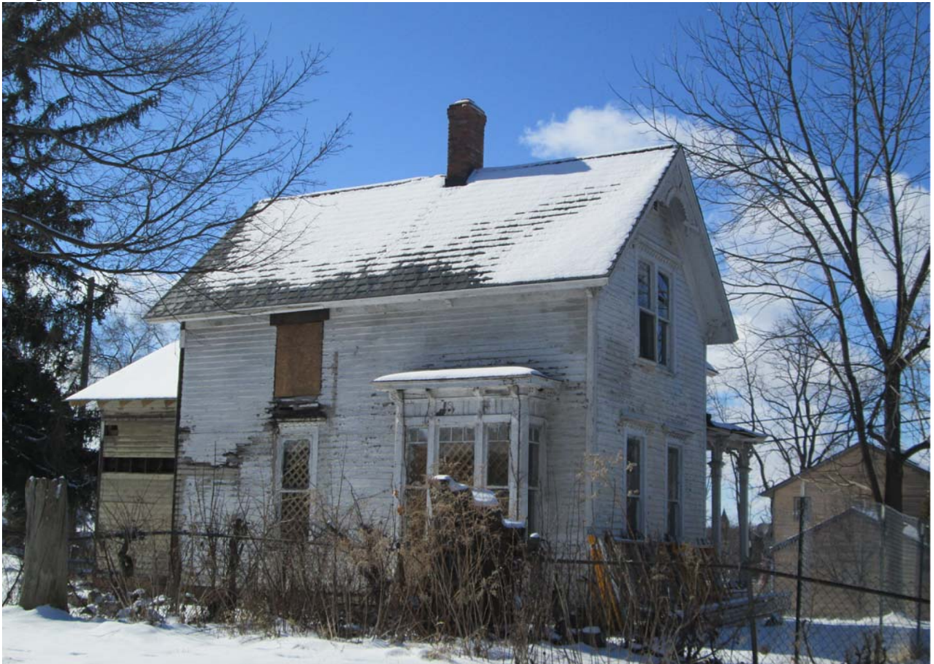
Facing southwest to facade and west elevation
