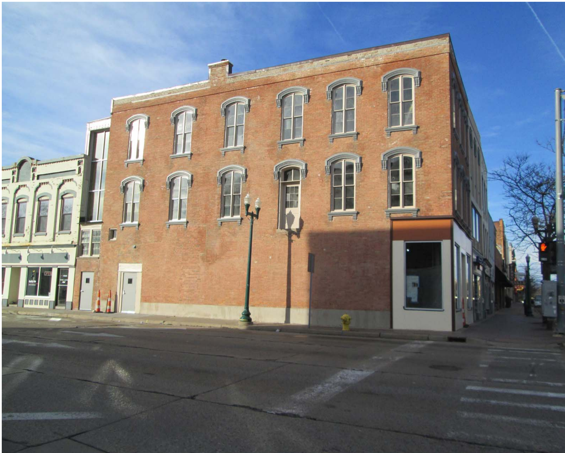
Facing east-southeast to east elevation
