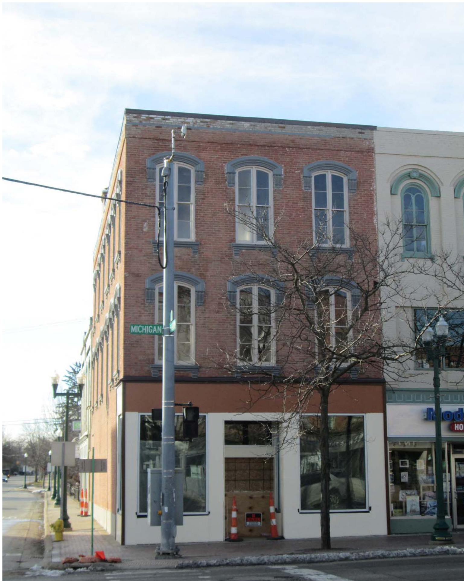
Facing south-southwest to facade
