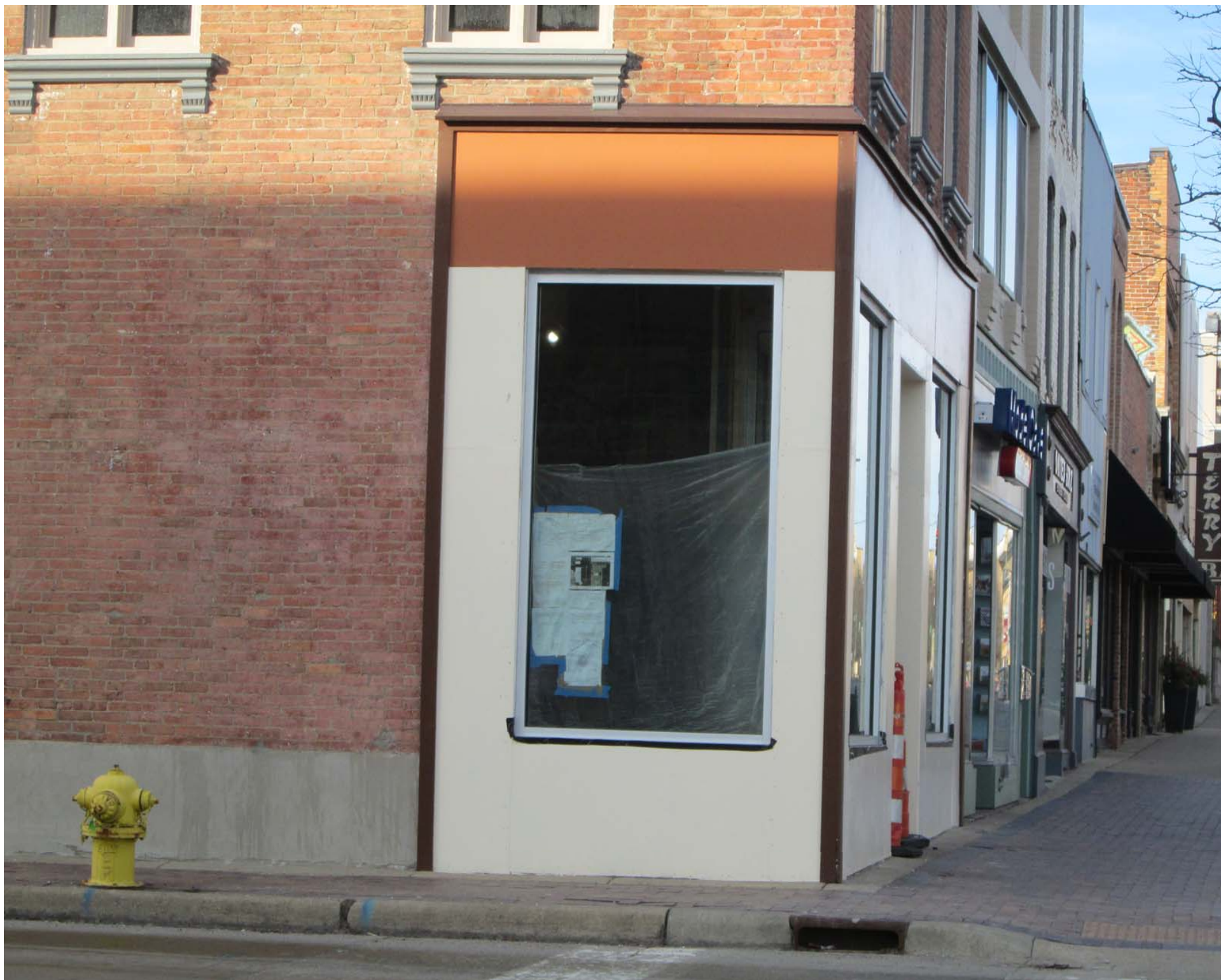
Detail of east elevation storefront window
