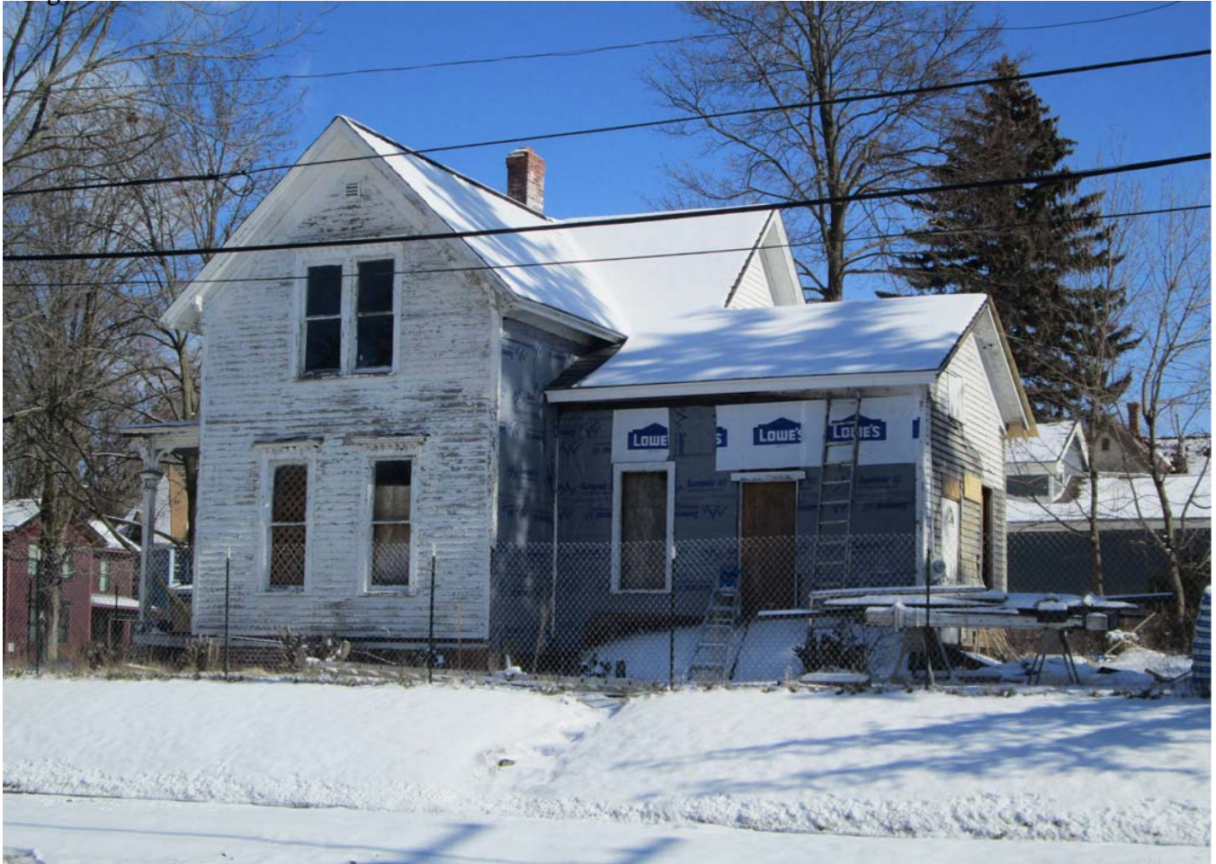
Facing northeast to west and south elevations.
