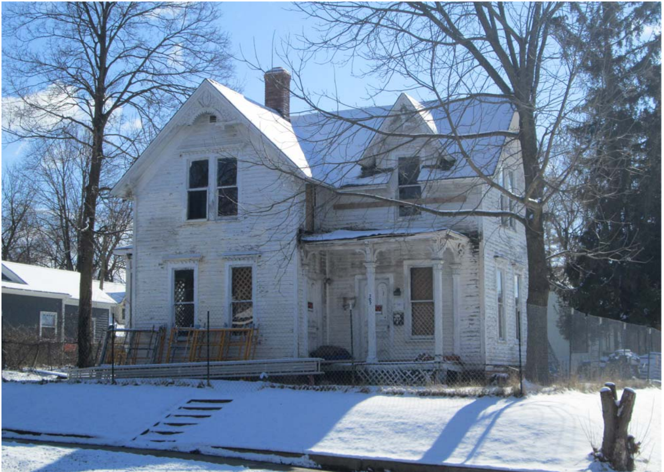
Facing south-southeast to facade and west elevation
