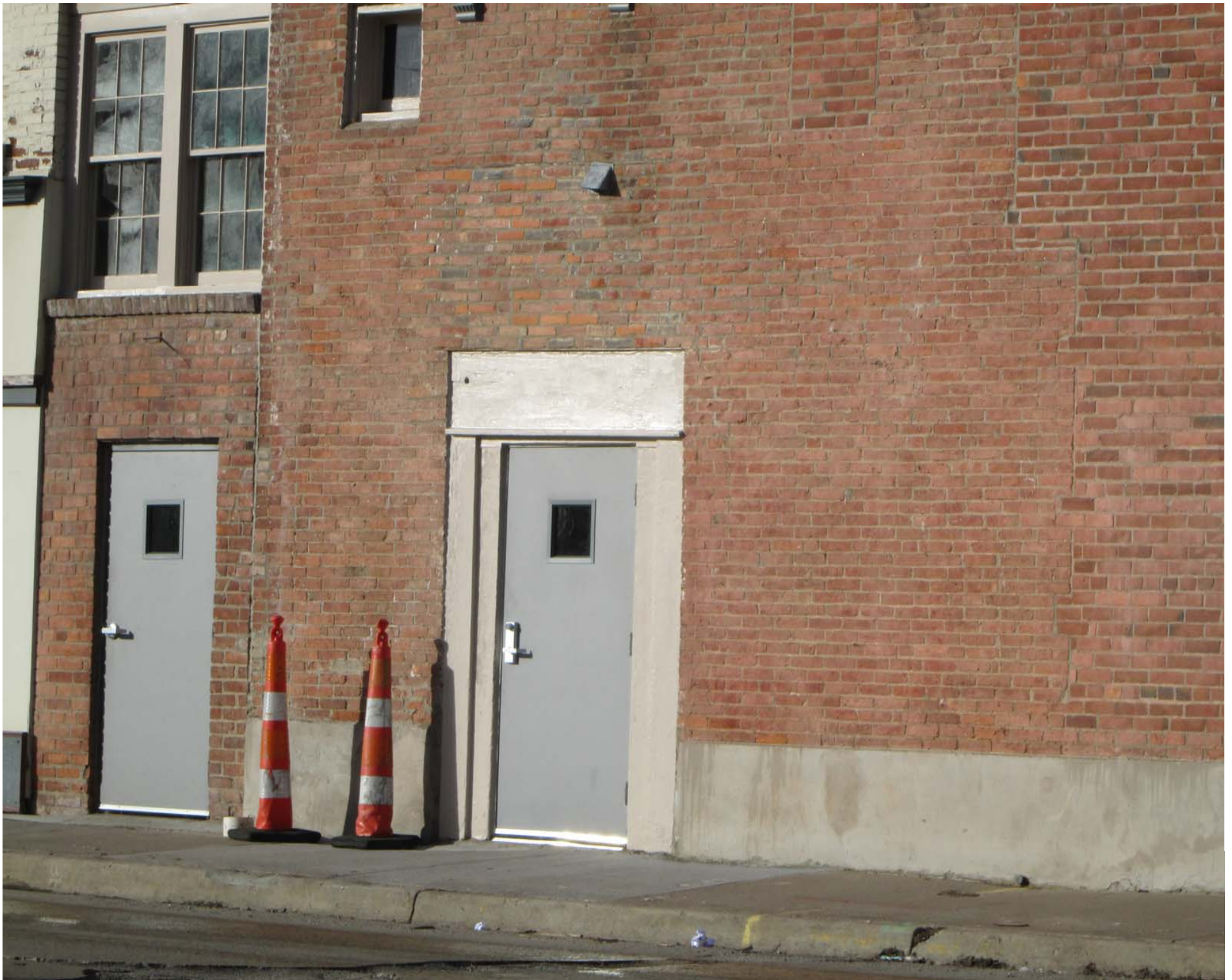
Detail of east elevation doors
