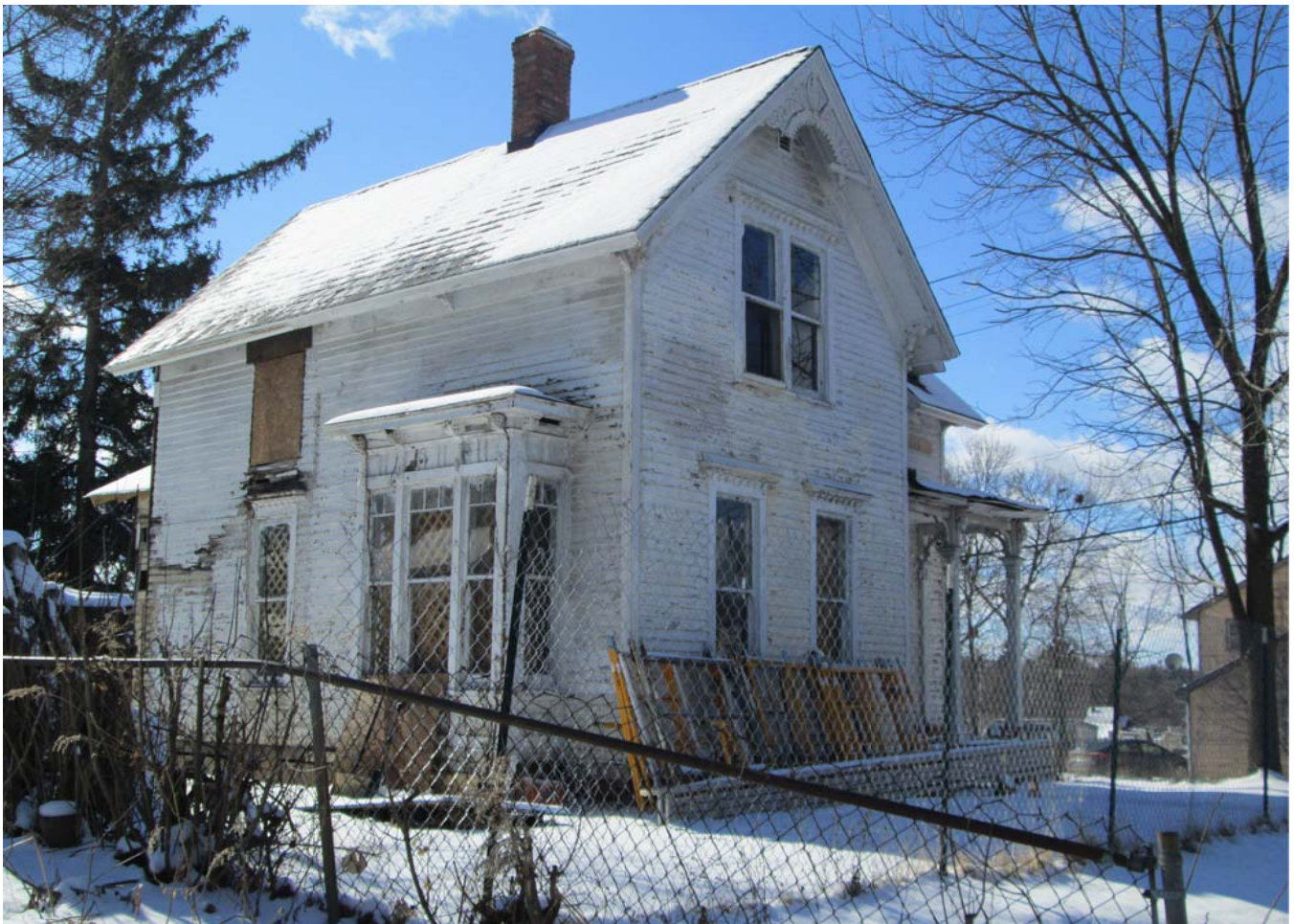
Facing southwest to facade and east elevation.
