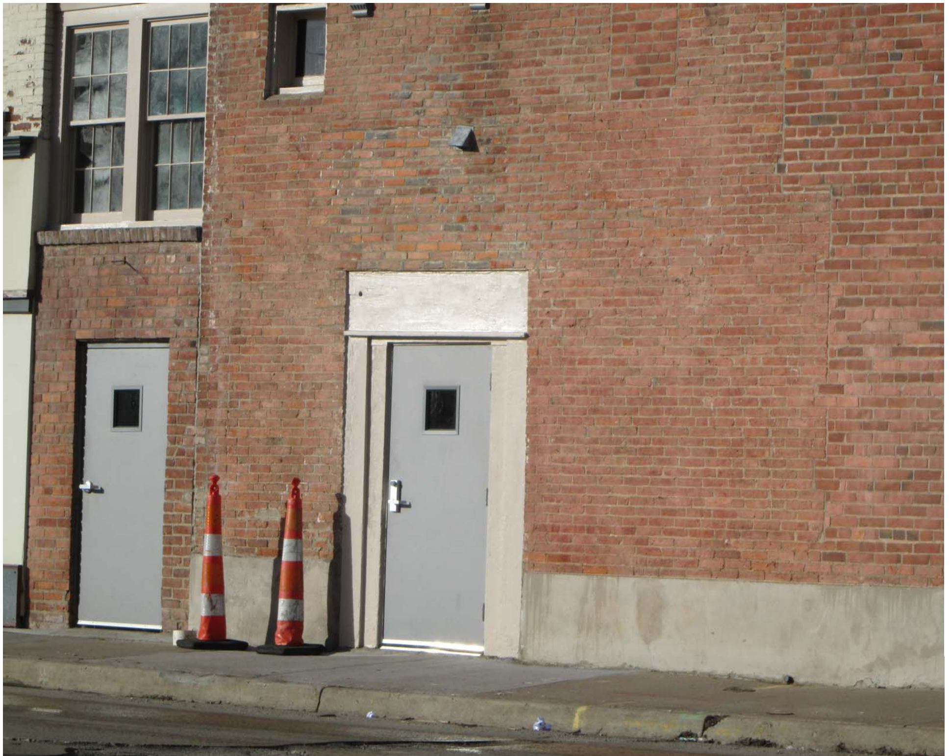
Detail of east elevation doors
