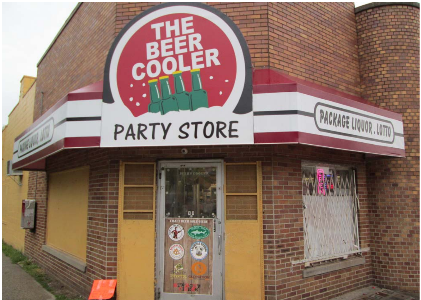
Detail of main entrance in 2016. The unapproved sign currently over the display window at right will be moved to the boarded-over window at left.
