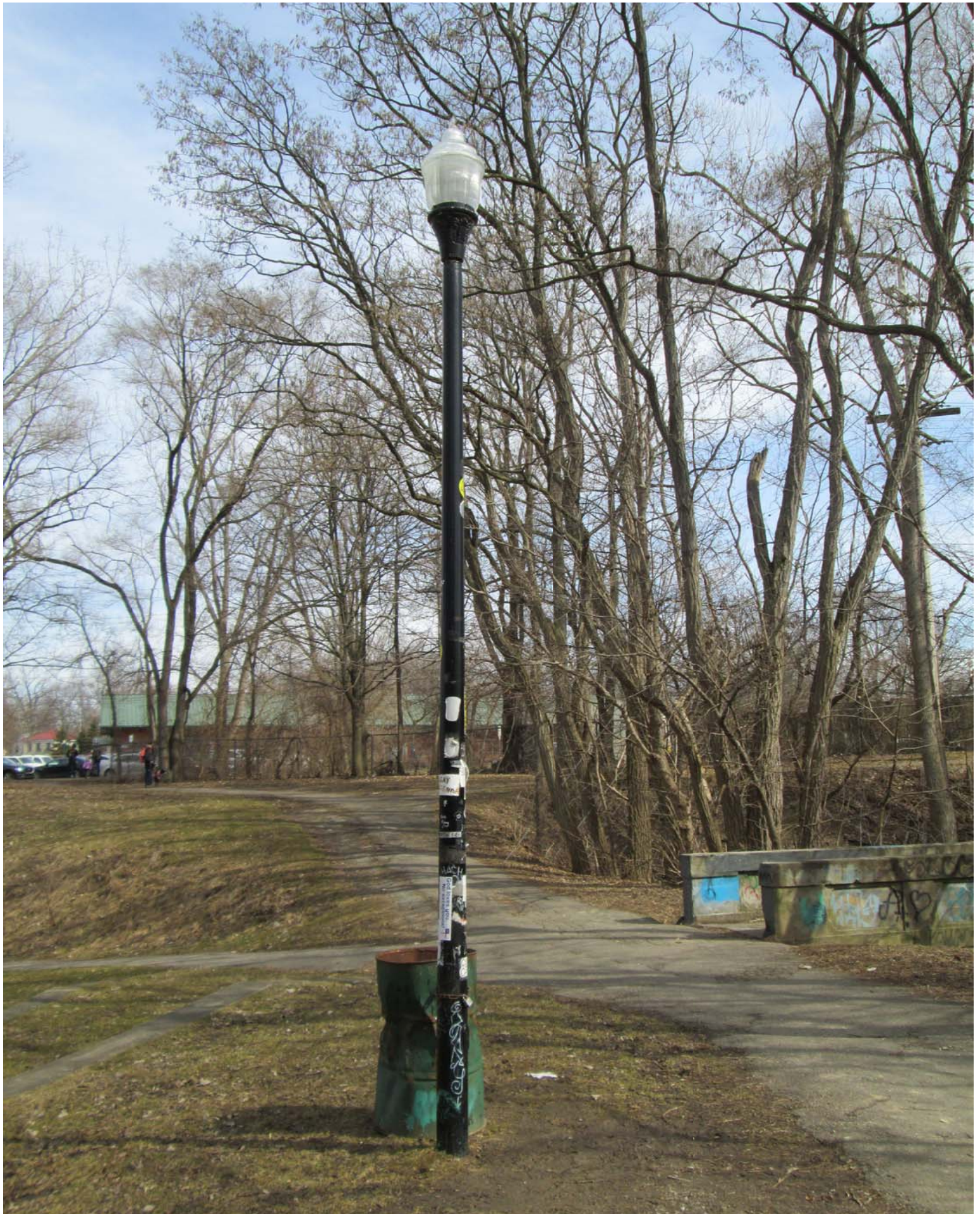
Light fixture currently in Frog Island Park
