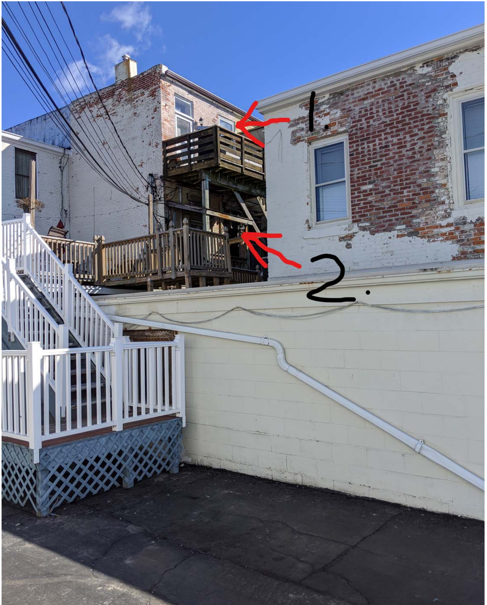
Facing northeast to south and west elevations.
