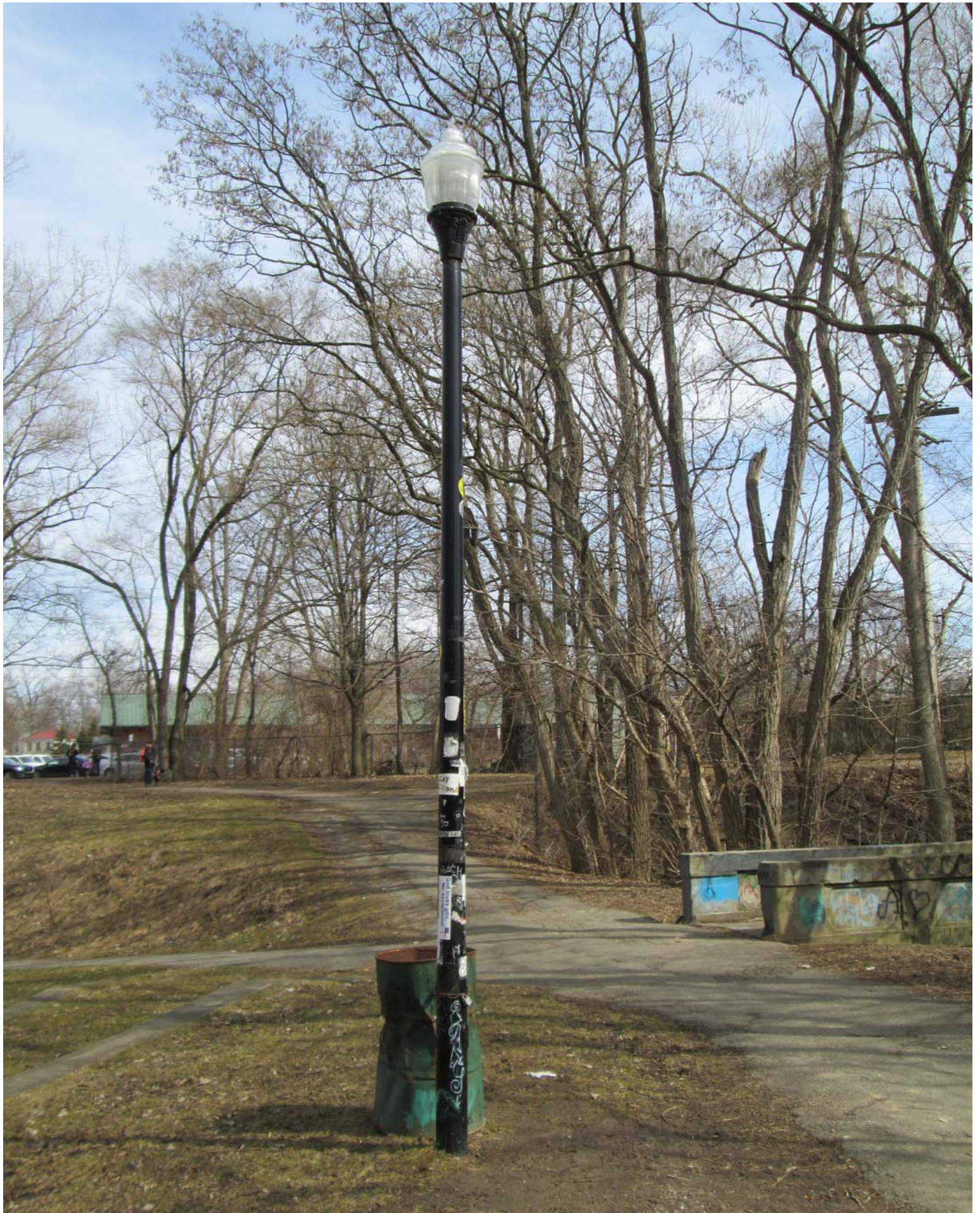
Light fixture currently in Frog Island Park
