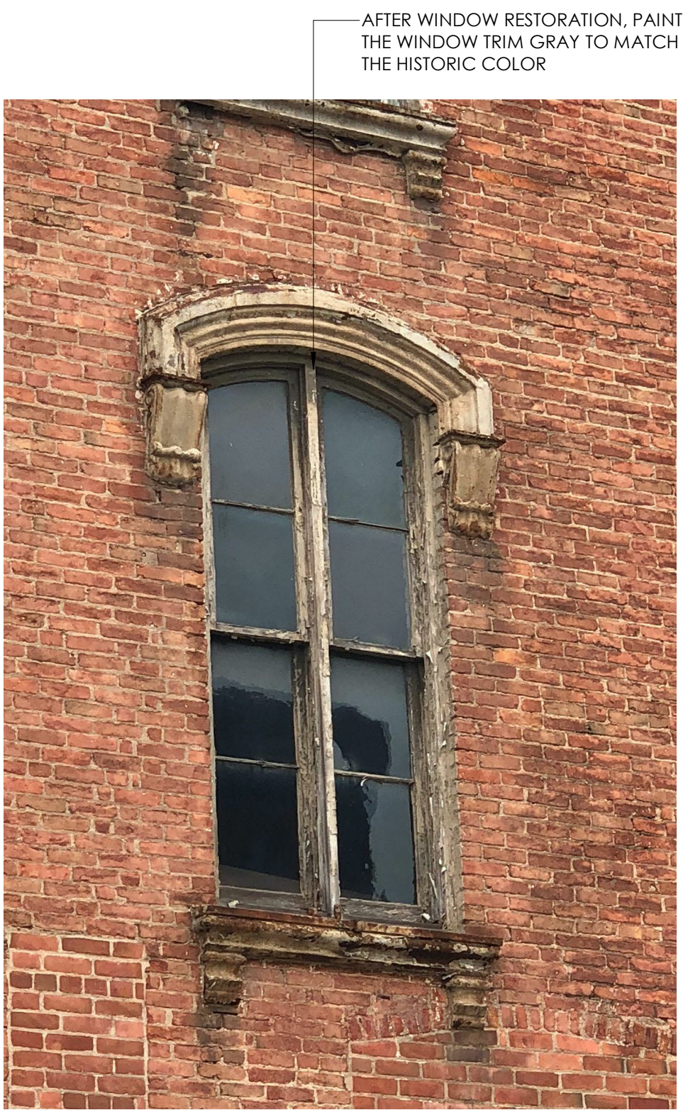
6 A401 EXISTING WINDOW IMAGES 1/8" = 1'-0"
