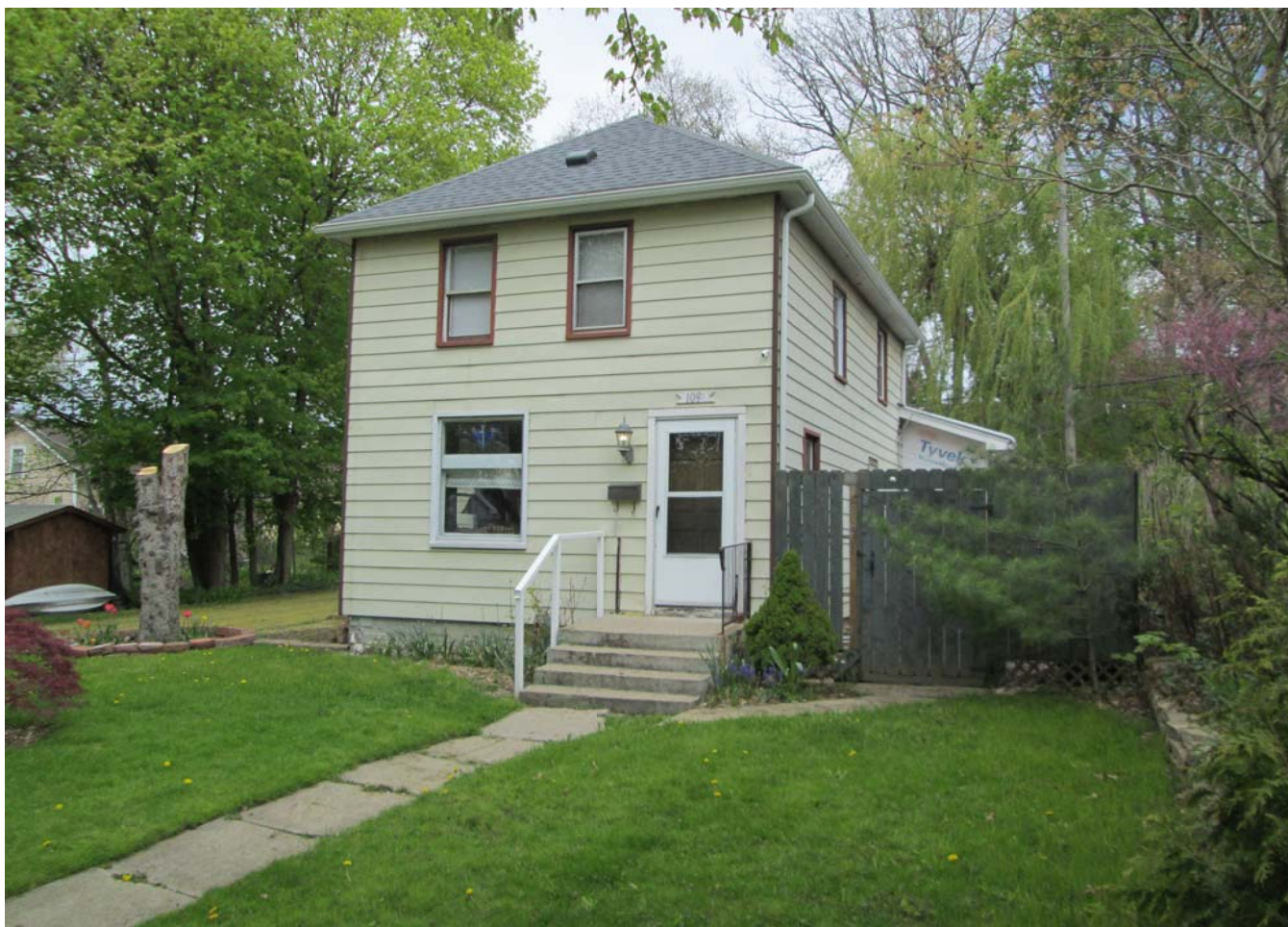
Facing north-northwest to facade and west elevation
