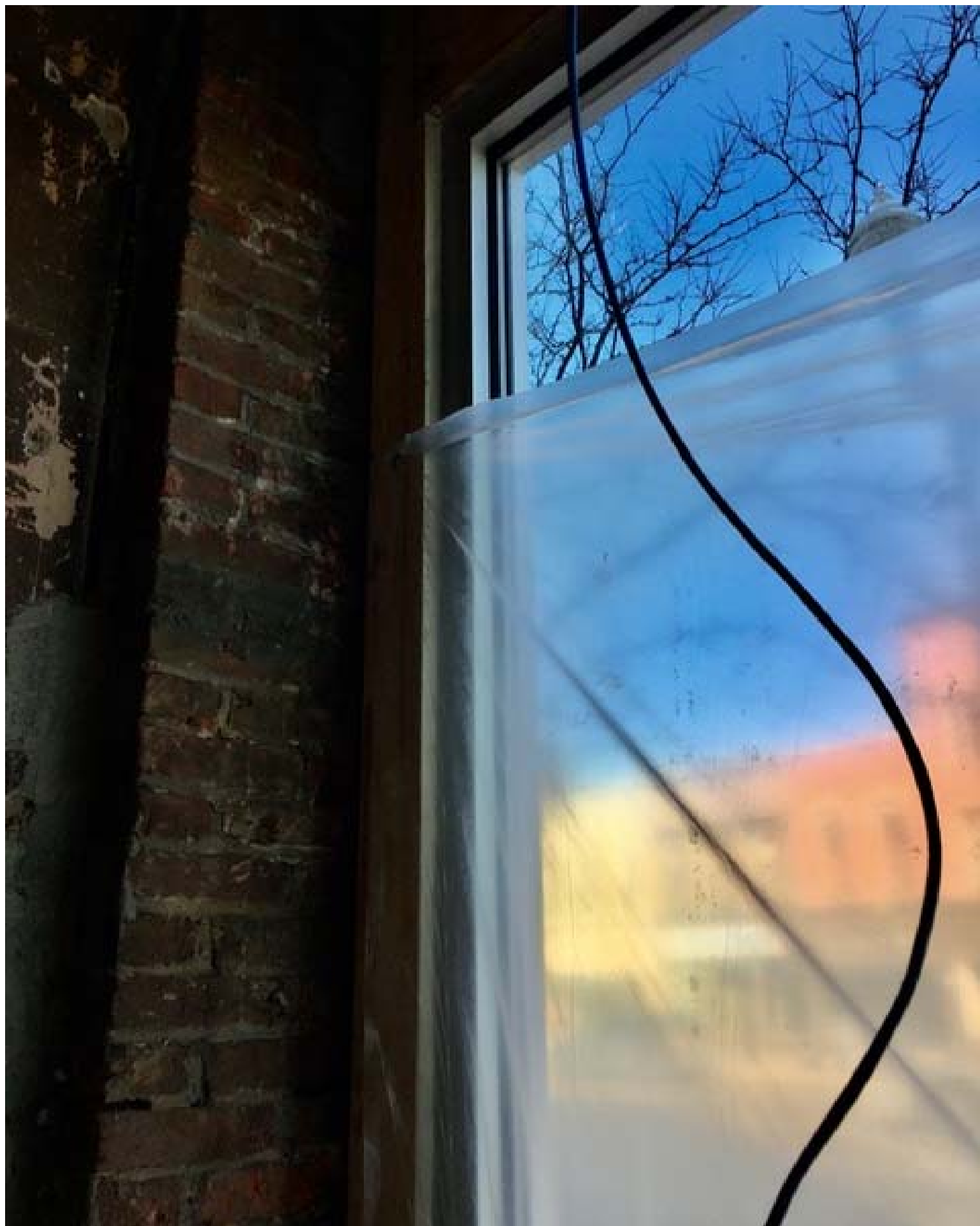
Photos showing interior structure.
