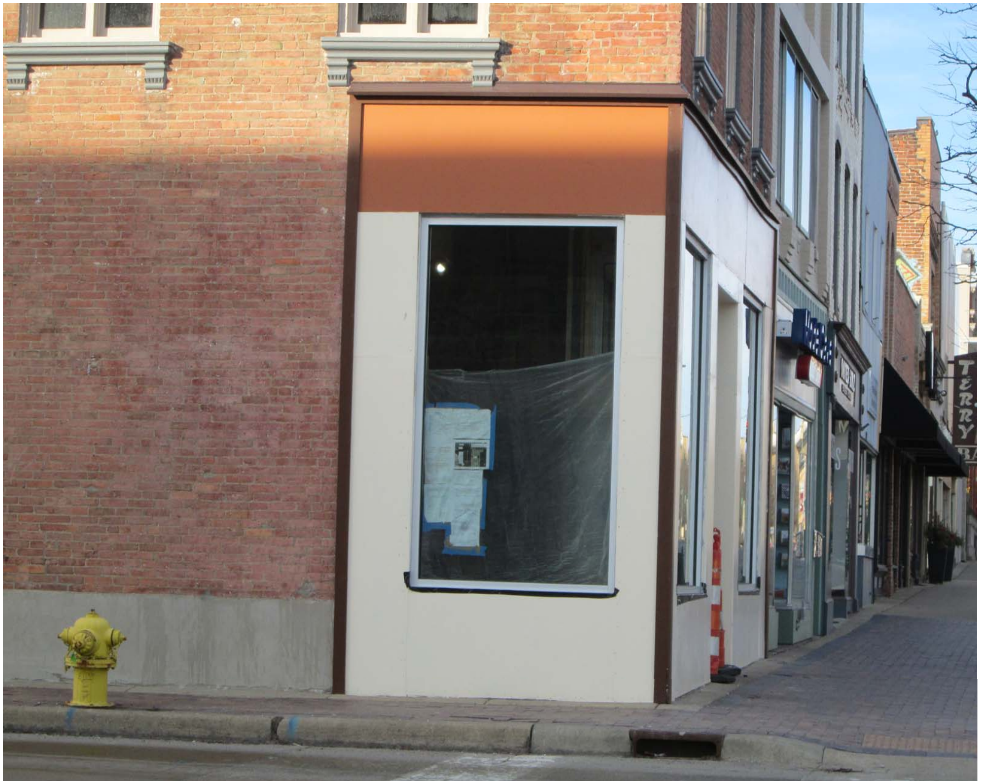
Facing west-southwet to northeast corner of storefront.
