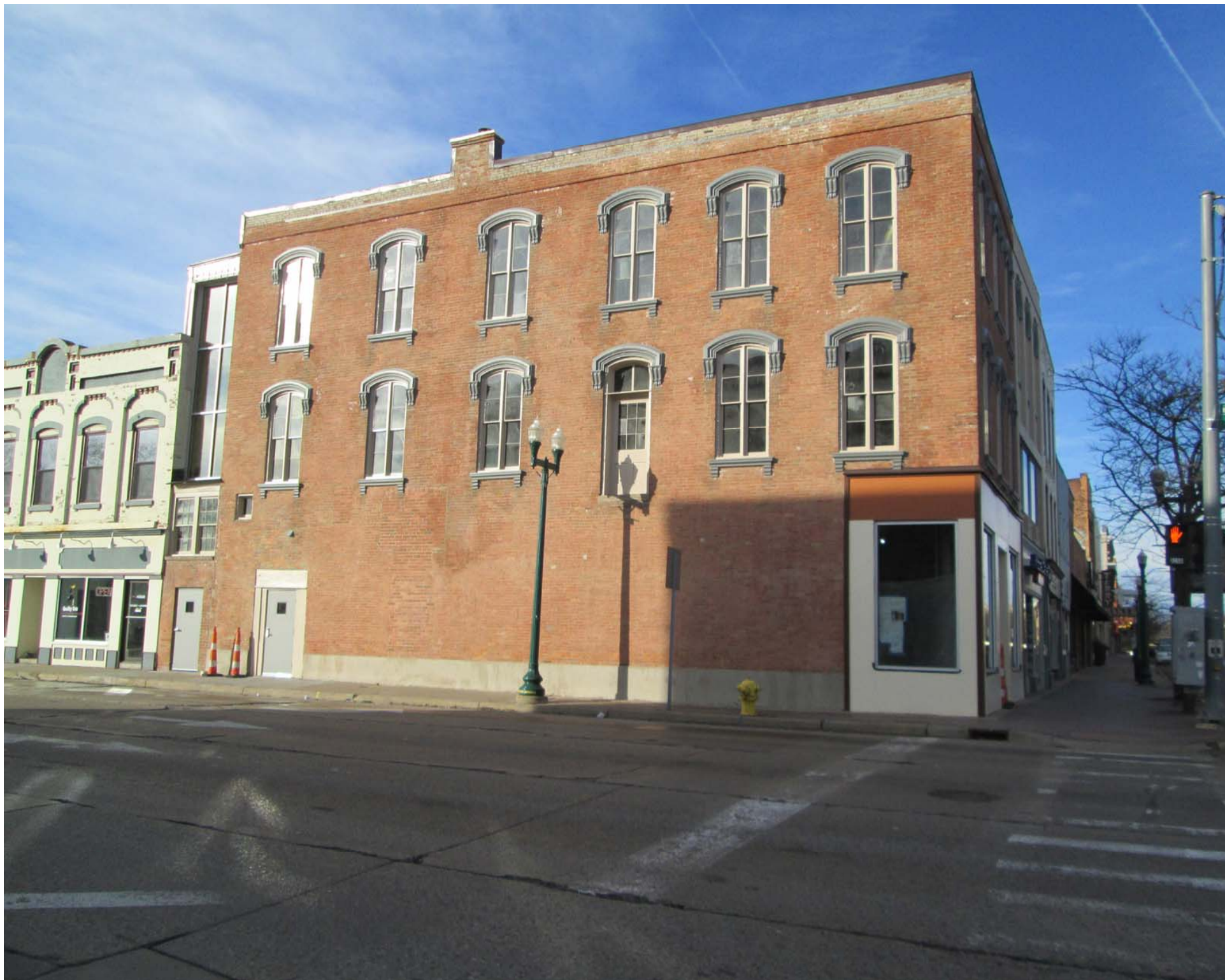
Facing west-southwest to east elevation.
