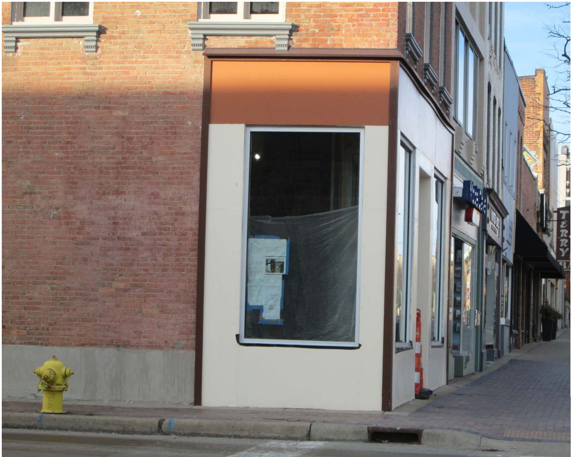
Facing west-southwet to northeast corner of storefront.
