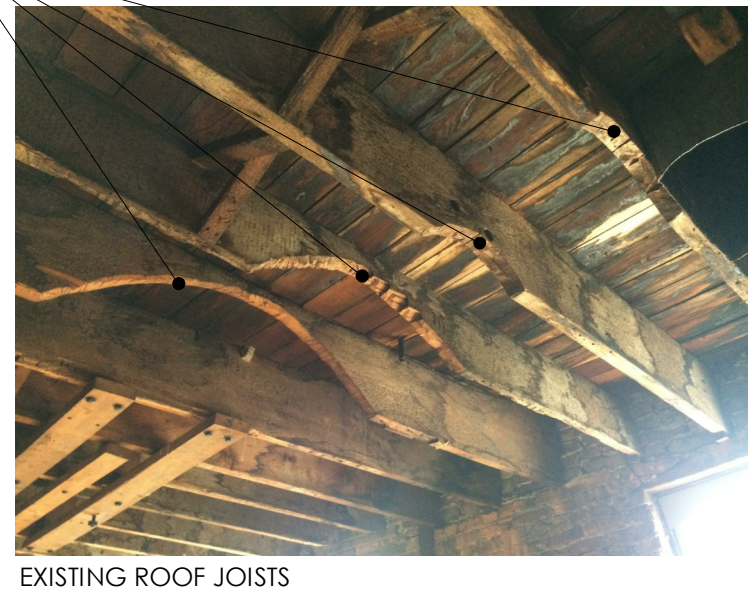
EXISTING ROOF JOISTS
