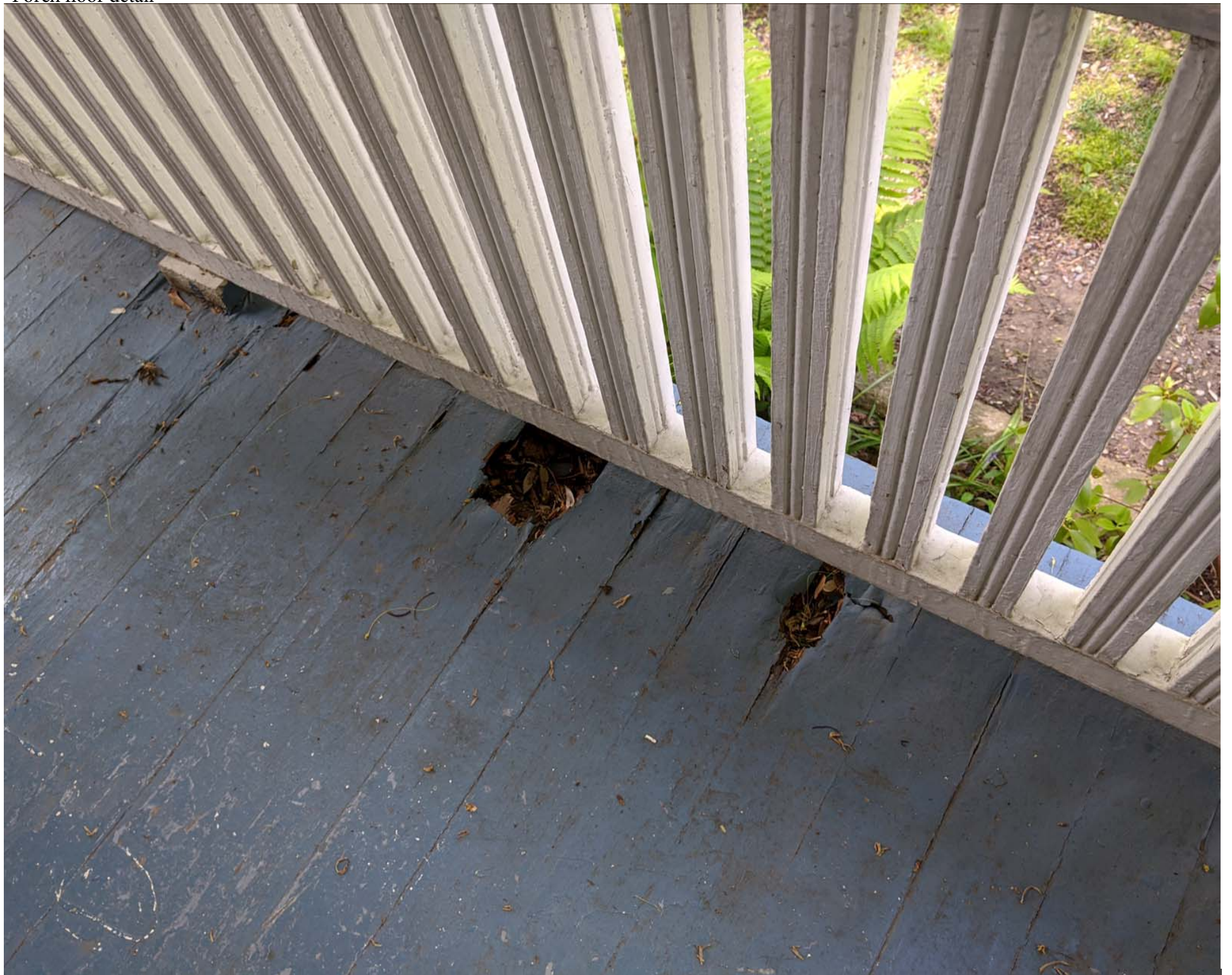
Porch floor detail
