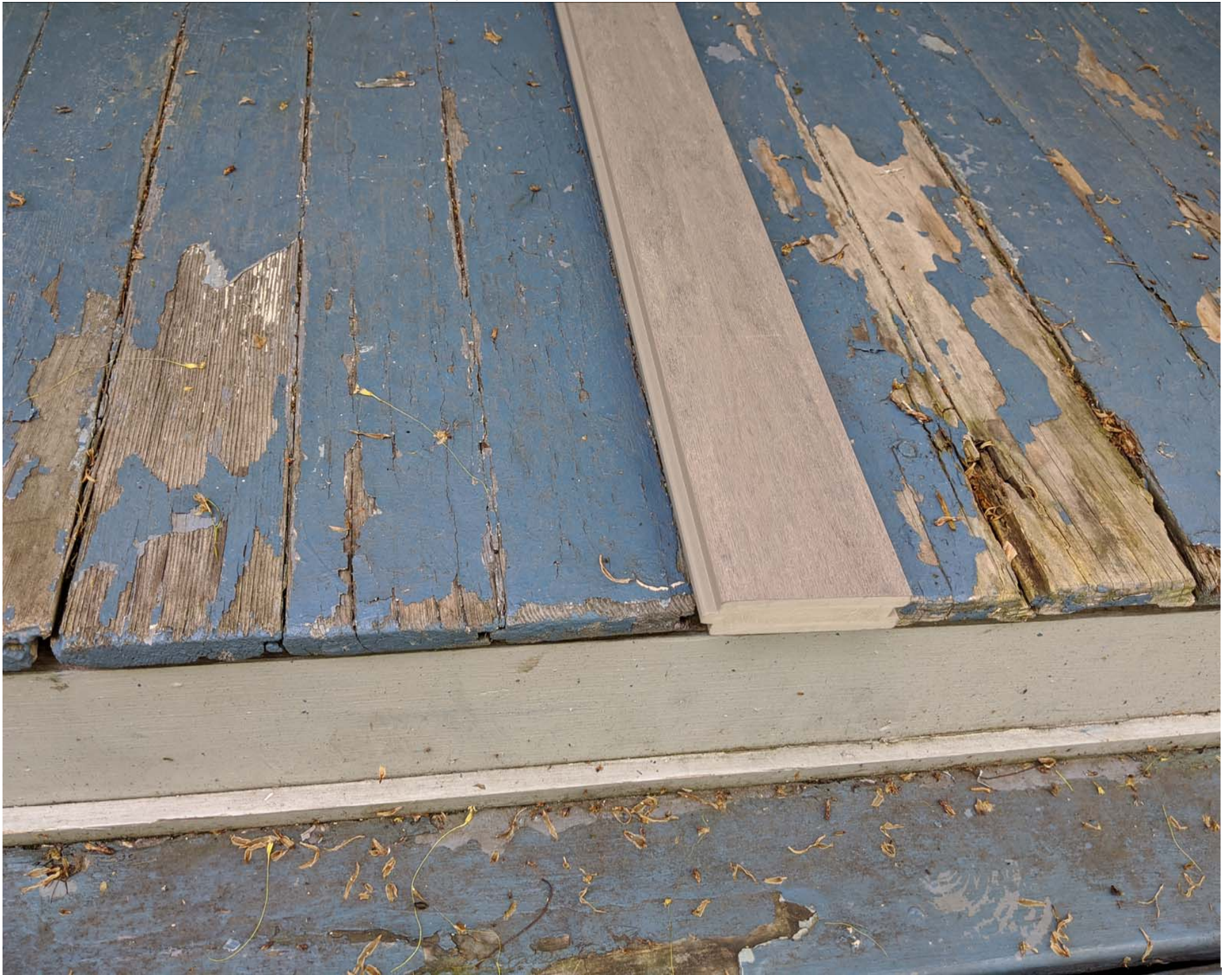
Porch floor detail- Sample of Azek material next to existing porch floor
