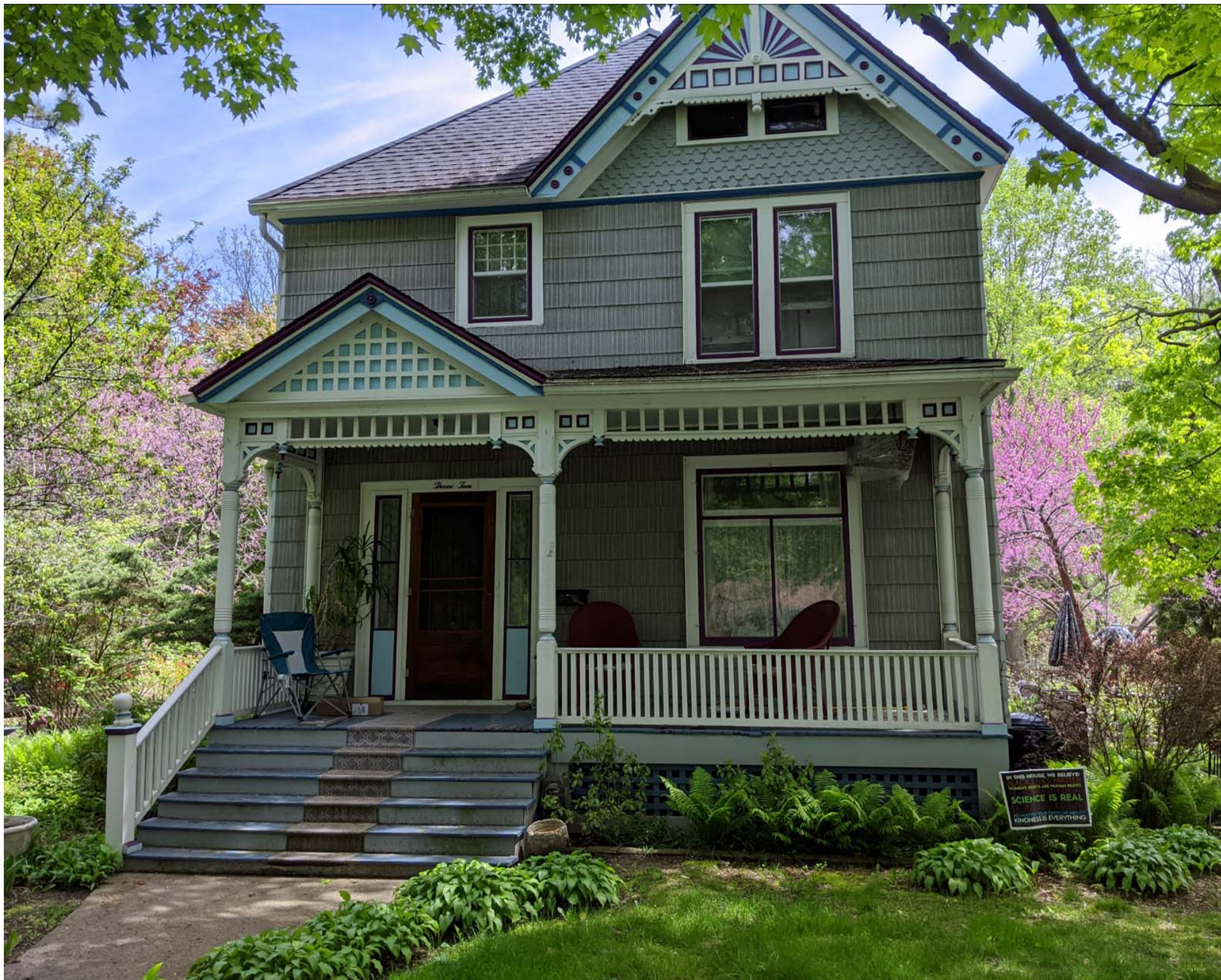
Facing east to facade
