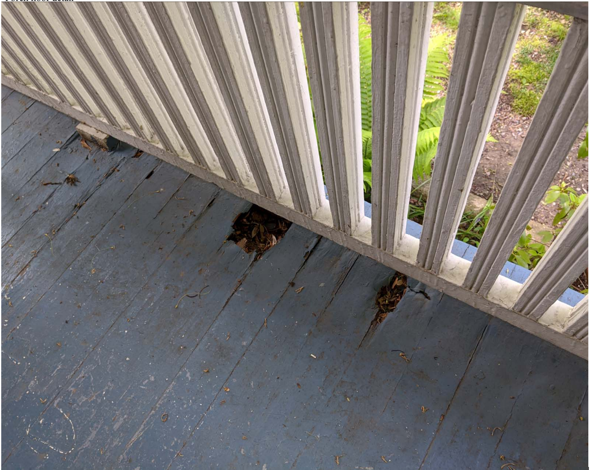
Porch floor detail
