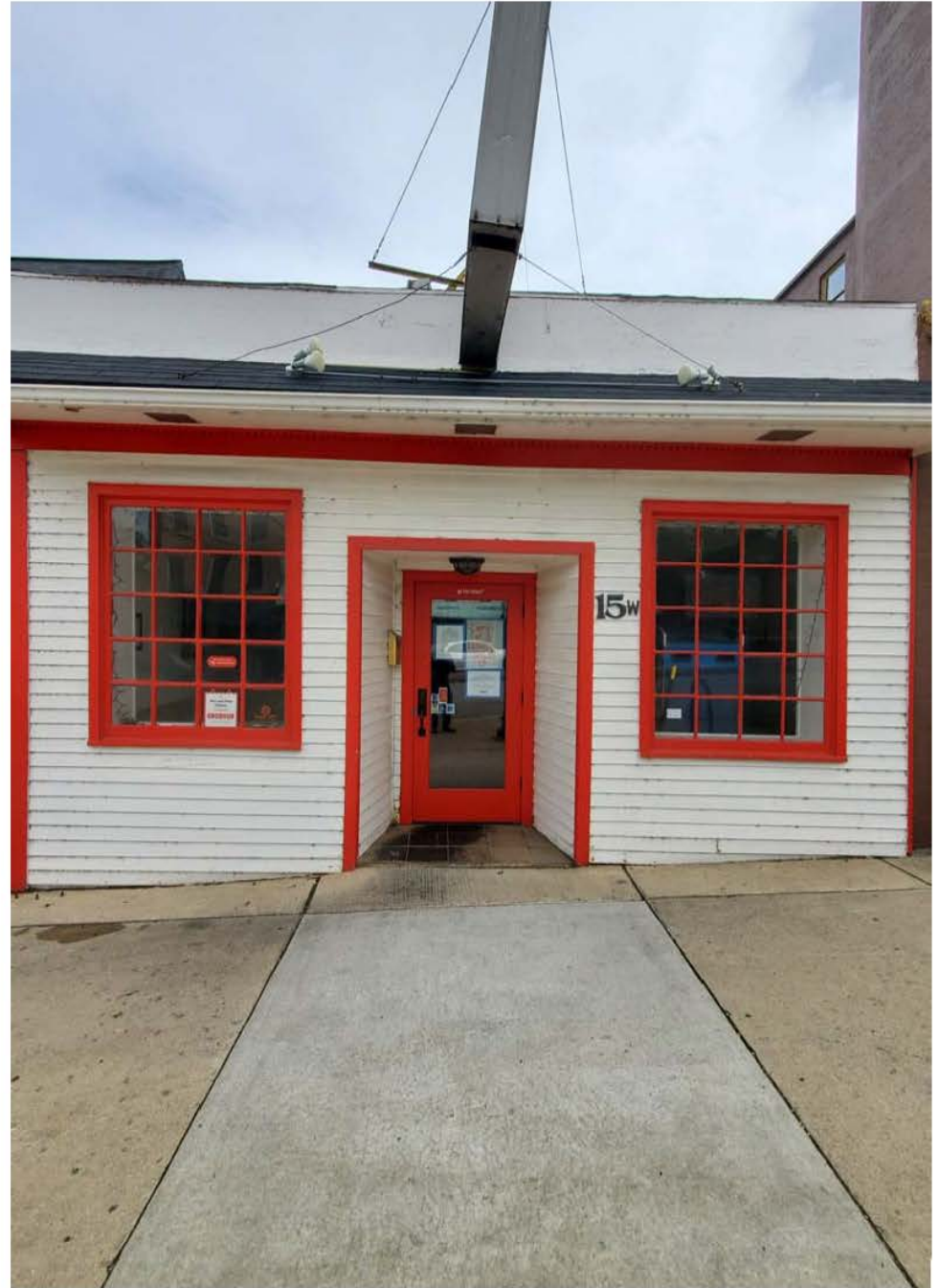
Facing south to facade, for reference.
