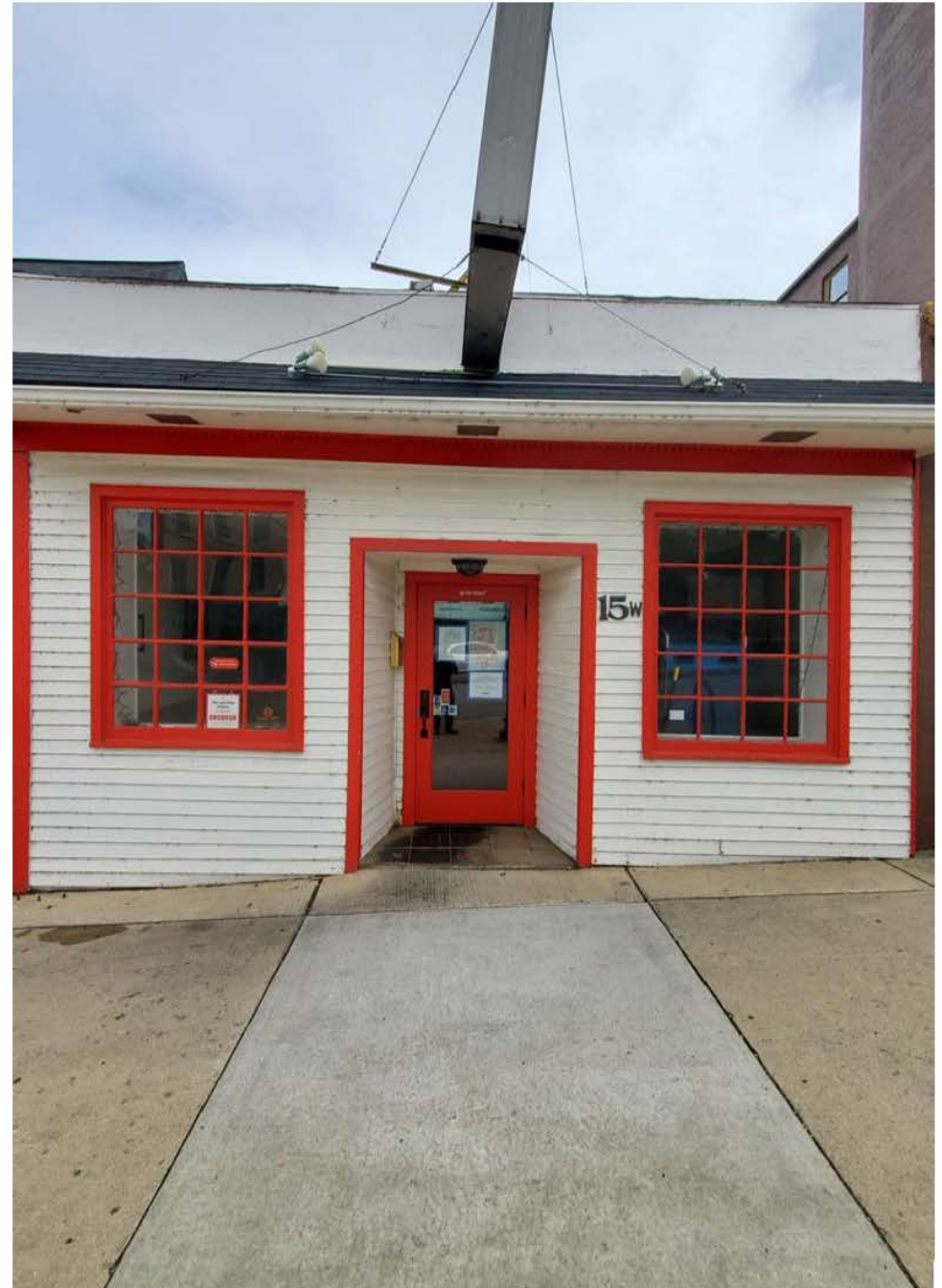
Facing south to facade, for reference.
