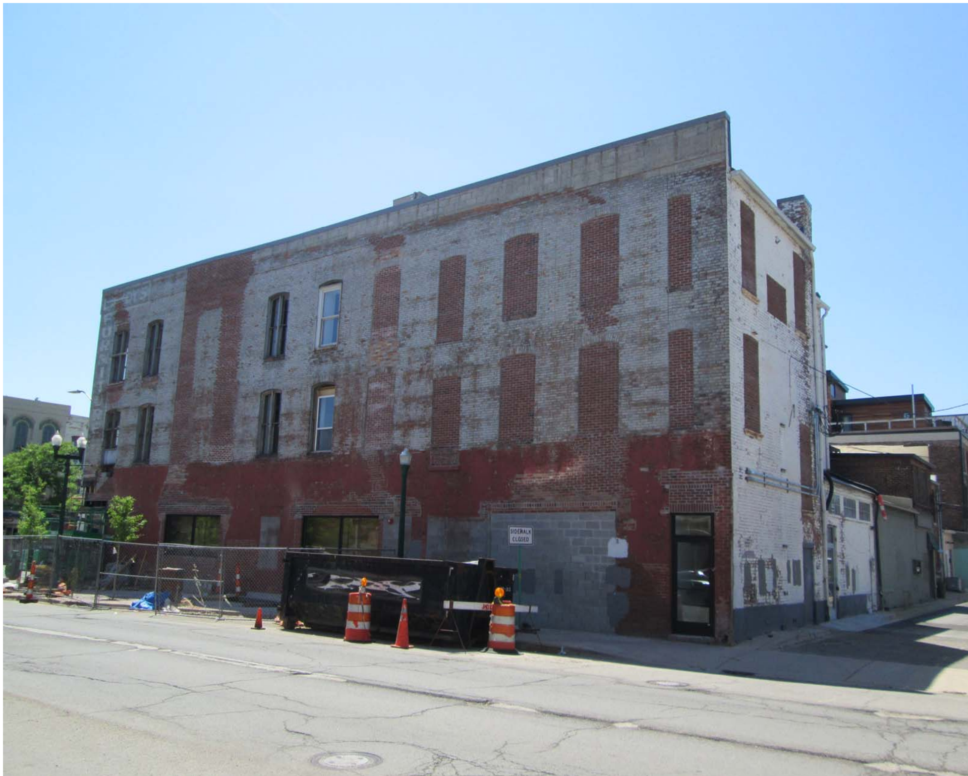
Facing southwest to north and east elevations
