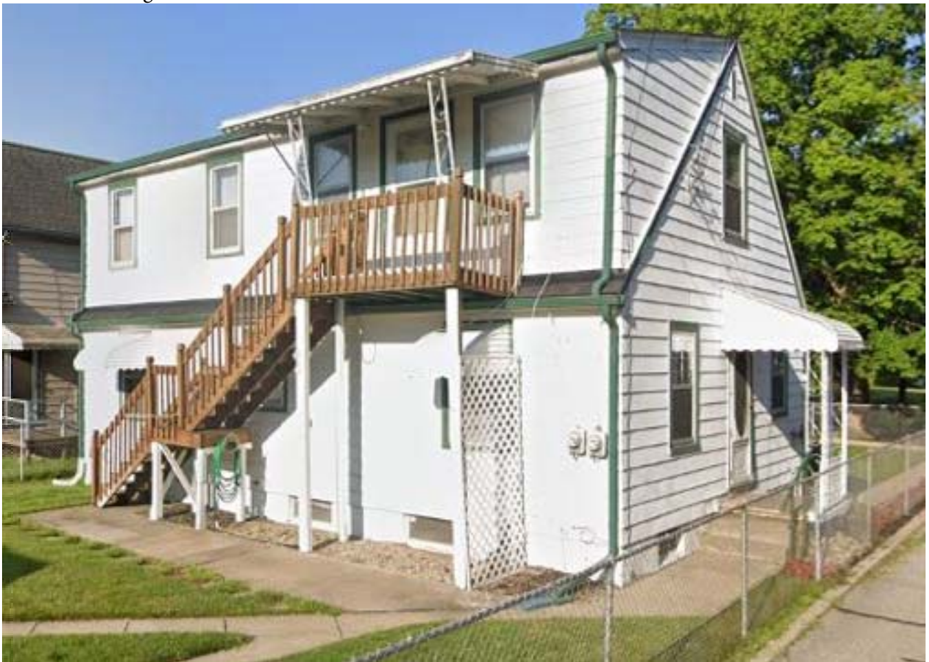
Facing southwest to north and east elevations.
