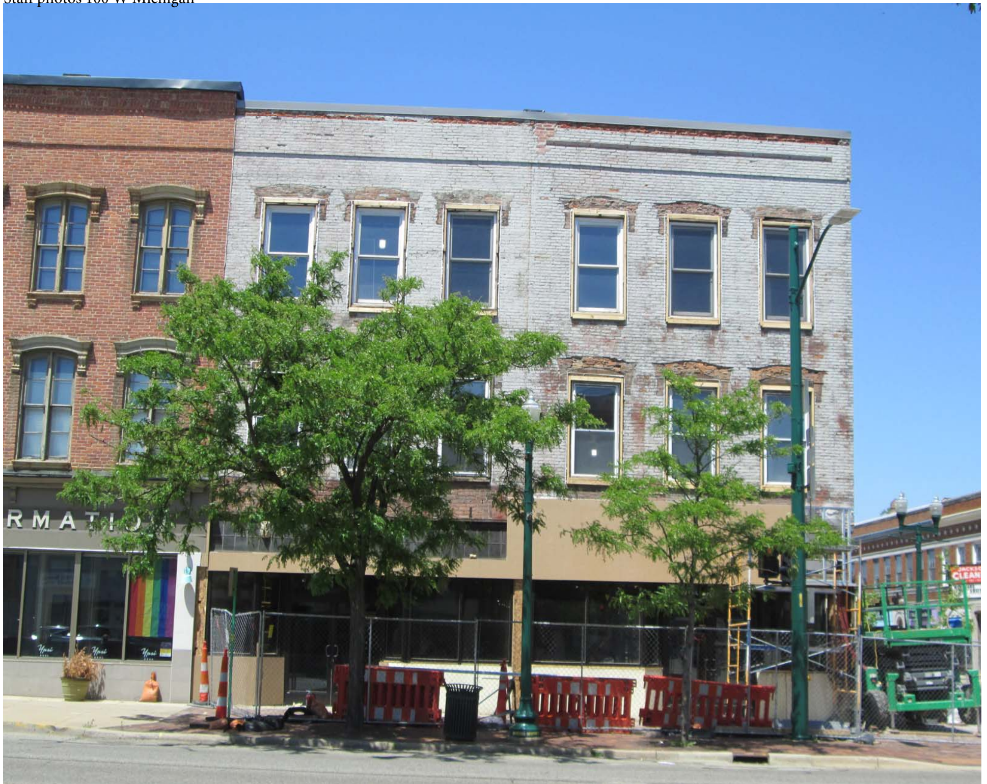
Facing north to facade
