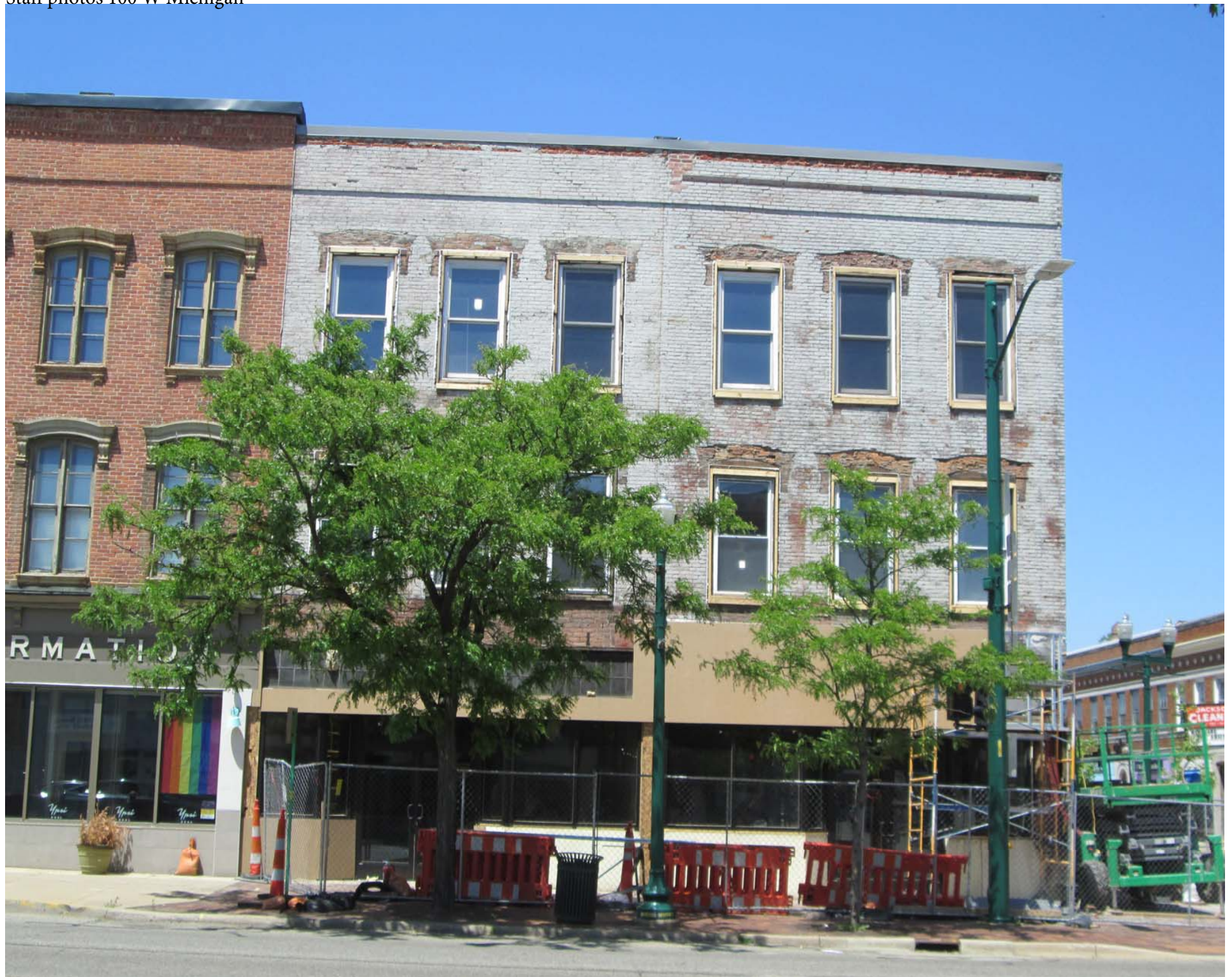
Facing north to facade
