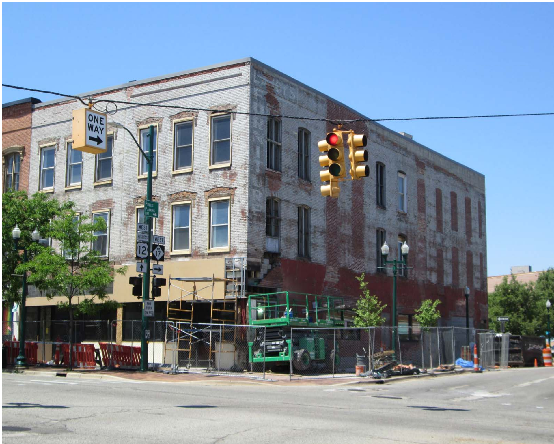
Facing northwest to facade and east elevation
