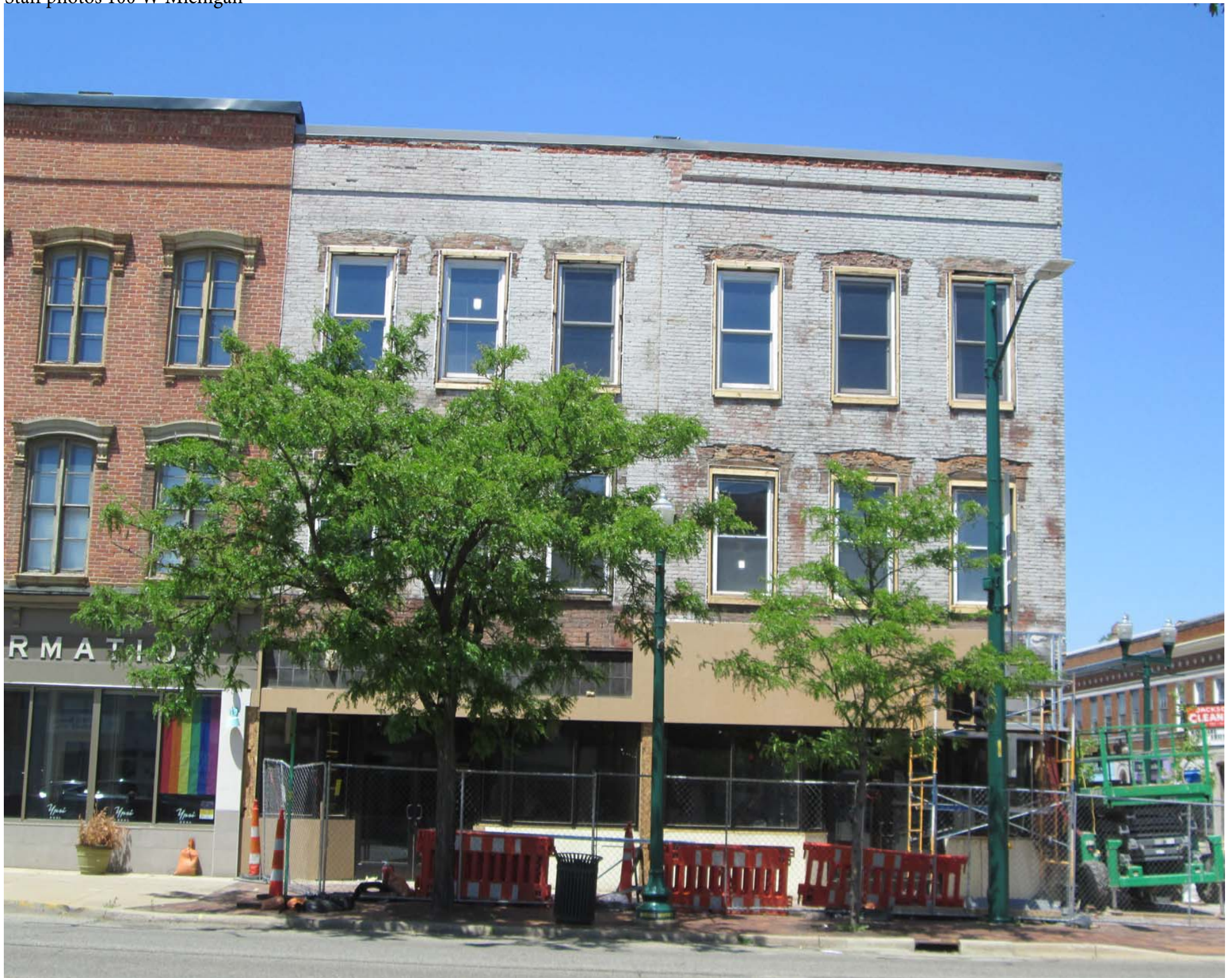
Facing north to facade
