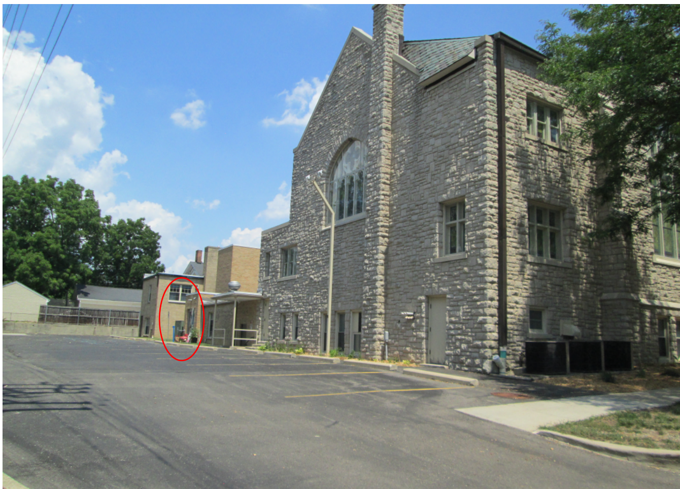
Facing northeast to west elevation from parking lot.
