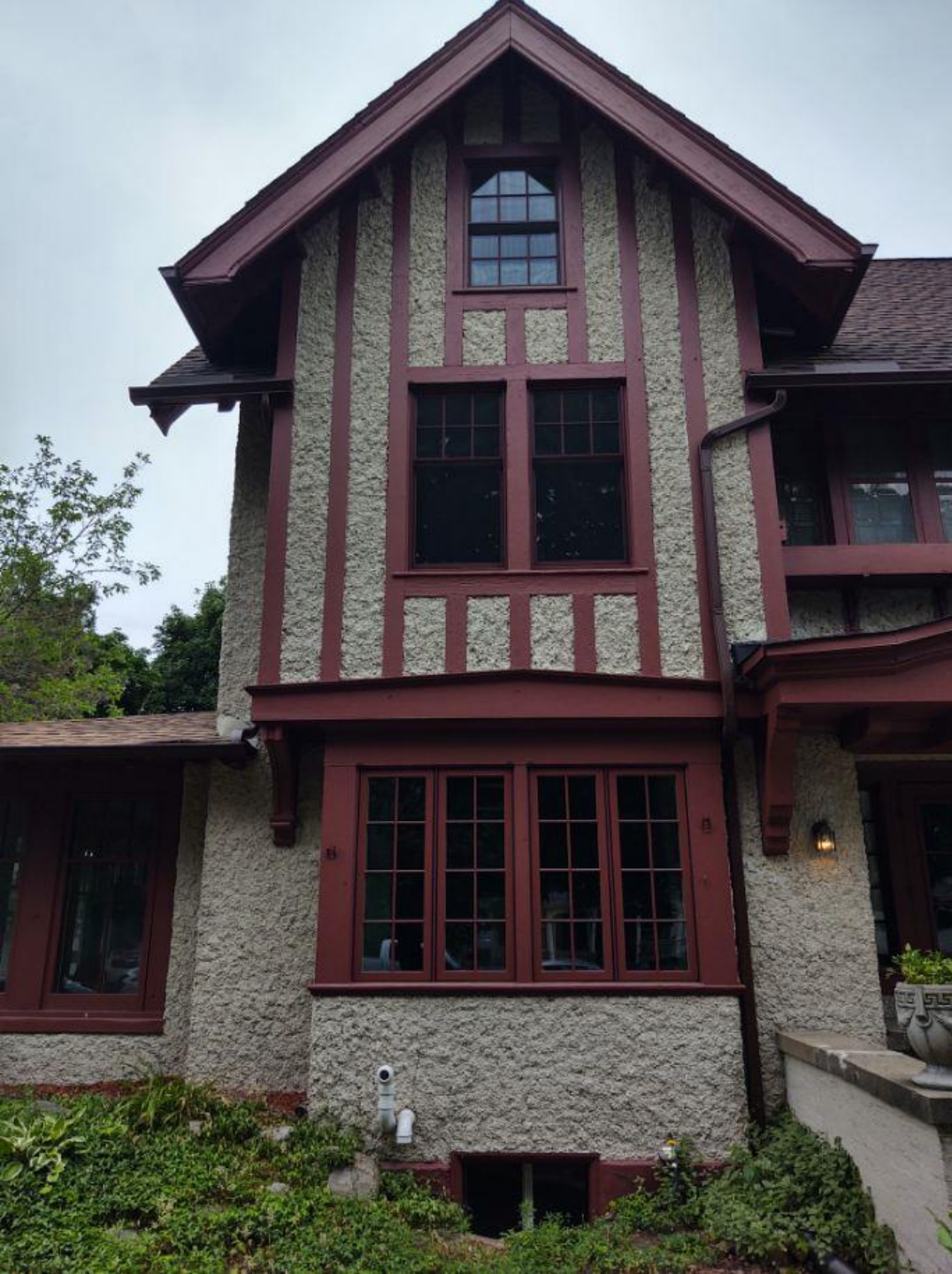
2019 Phase (Front of house)
