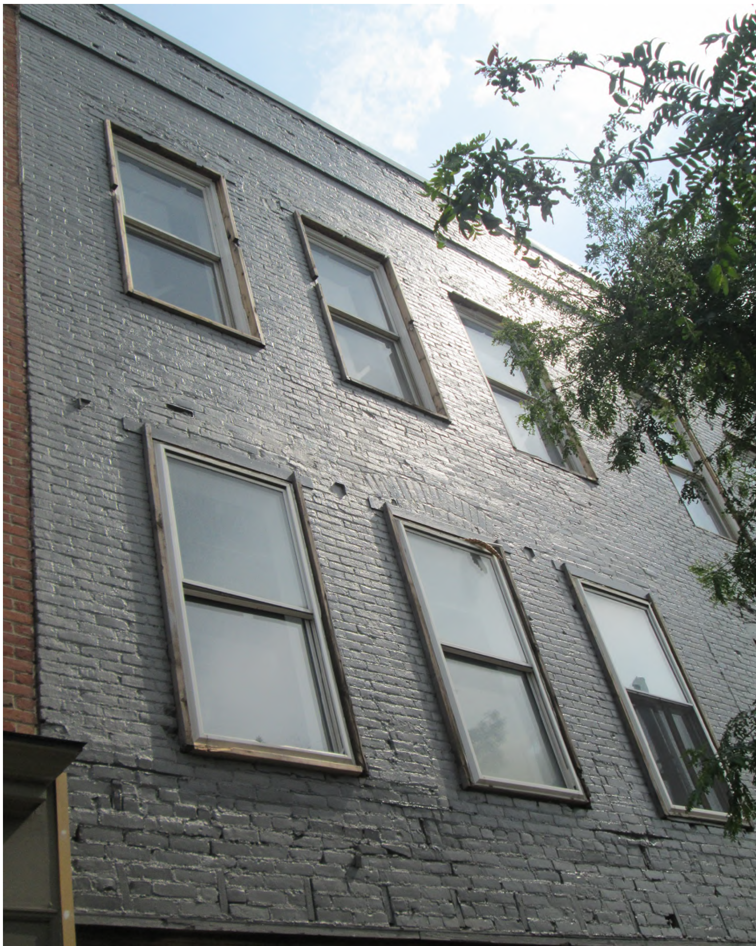
Facing northeast to upper stories of 102 W Michigan.
