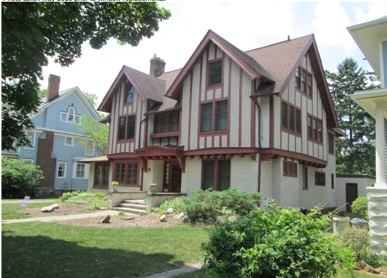
Photo taken July 2020 after window replacements.
