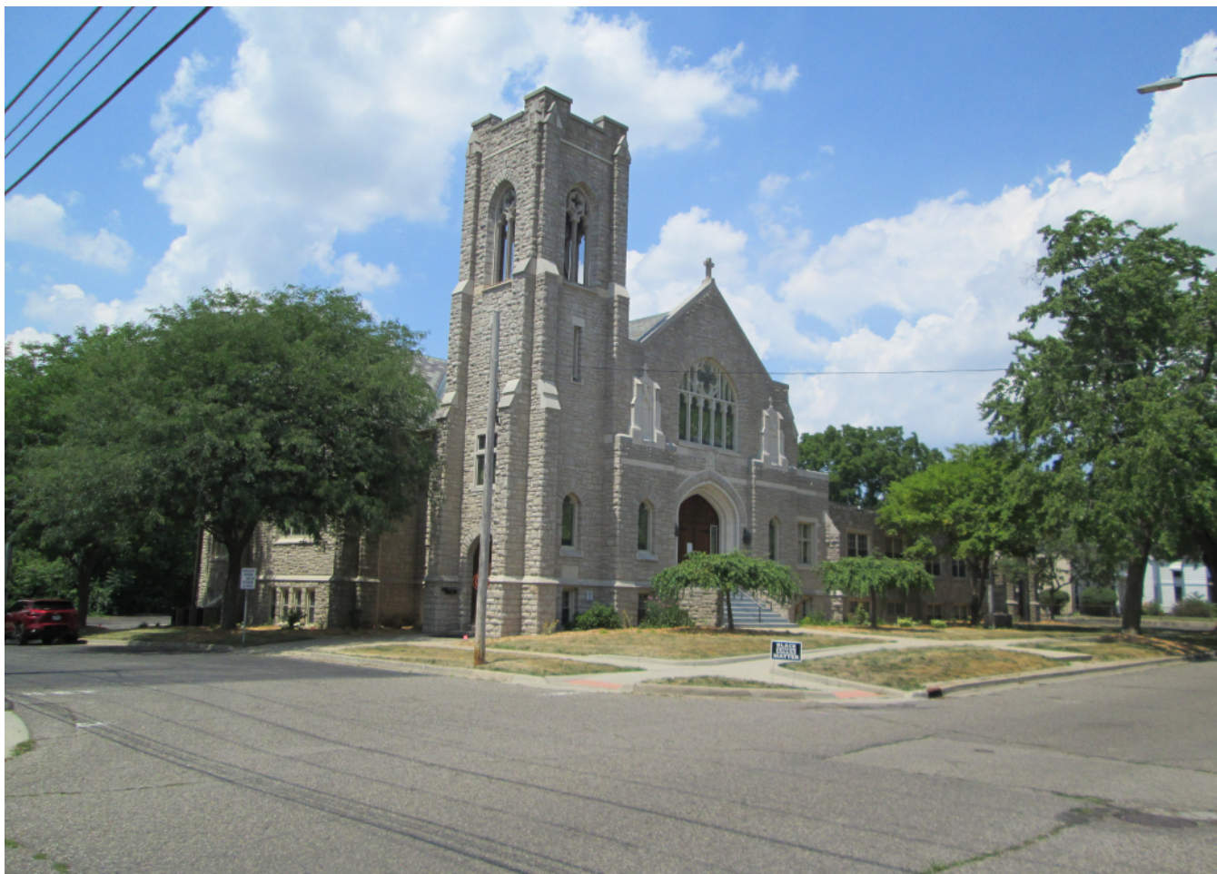
Facing northwest from River and North Streets to facade and south elevation (for reference).
