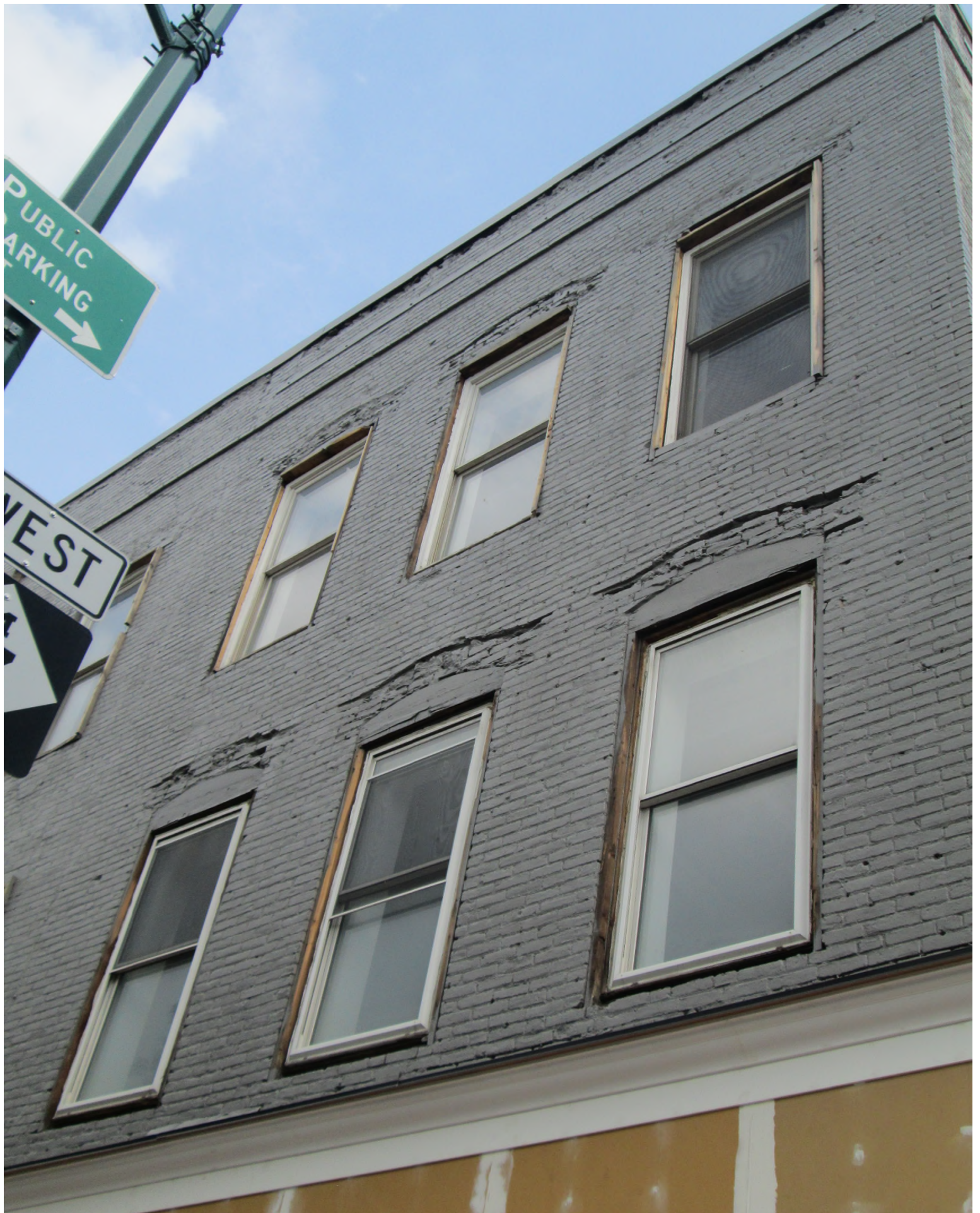
Facing northwest to upper stories of 100 W Michigan.
