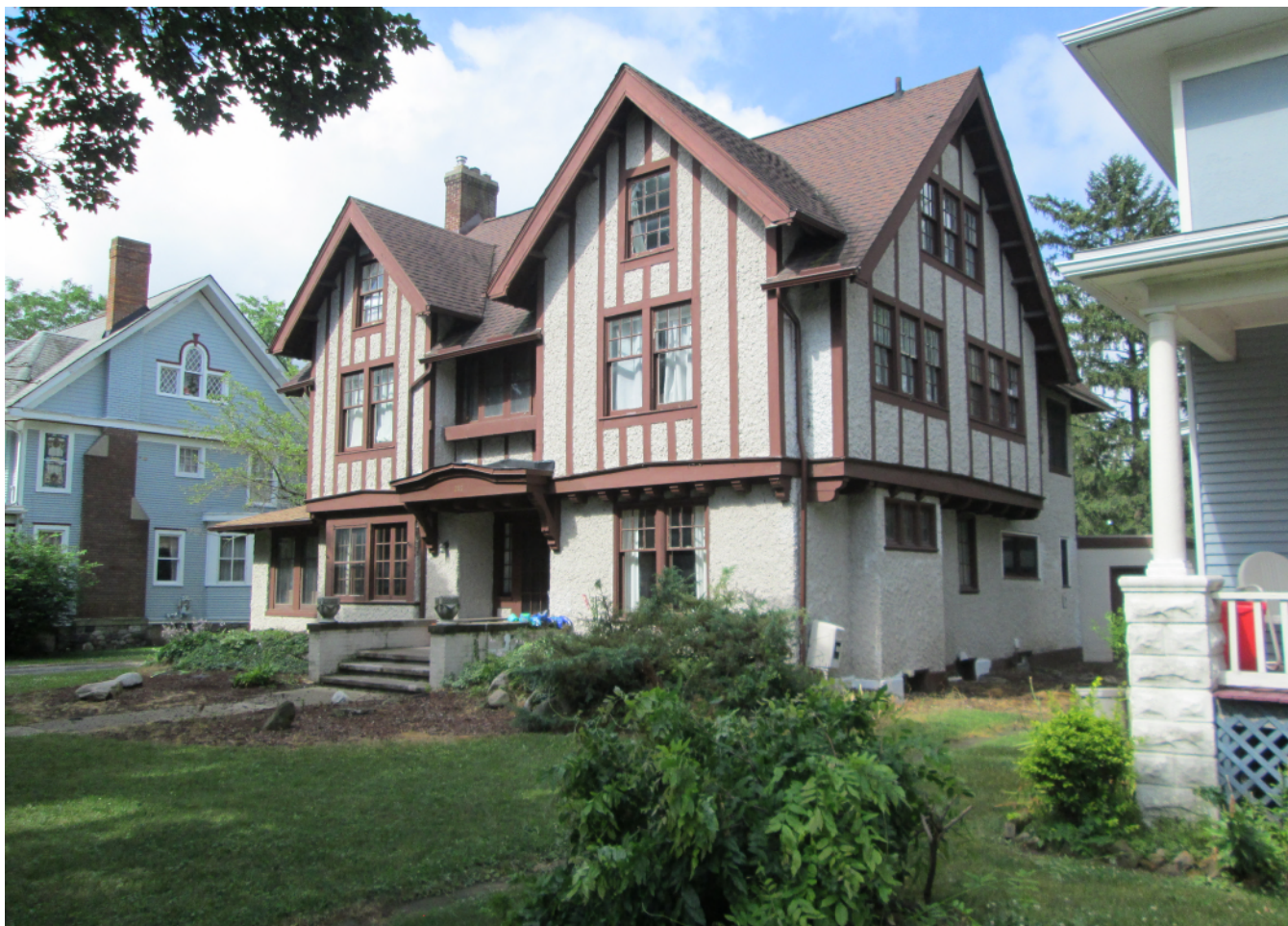
Photo taken May 2019 prior to window replacements.
