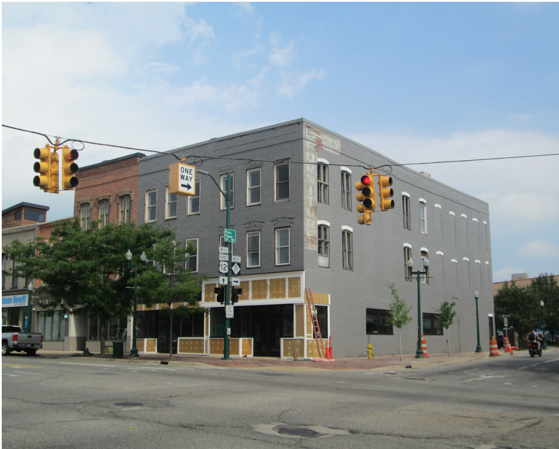
Facing northwest to facade and east elevation.
