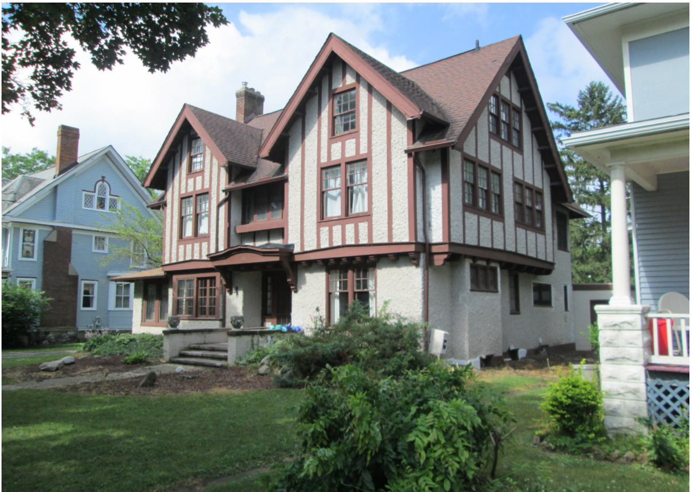
Photo taken May 2019 prior to window replacements.
