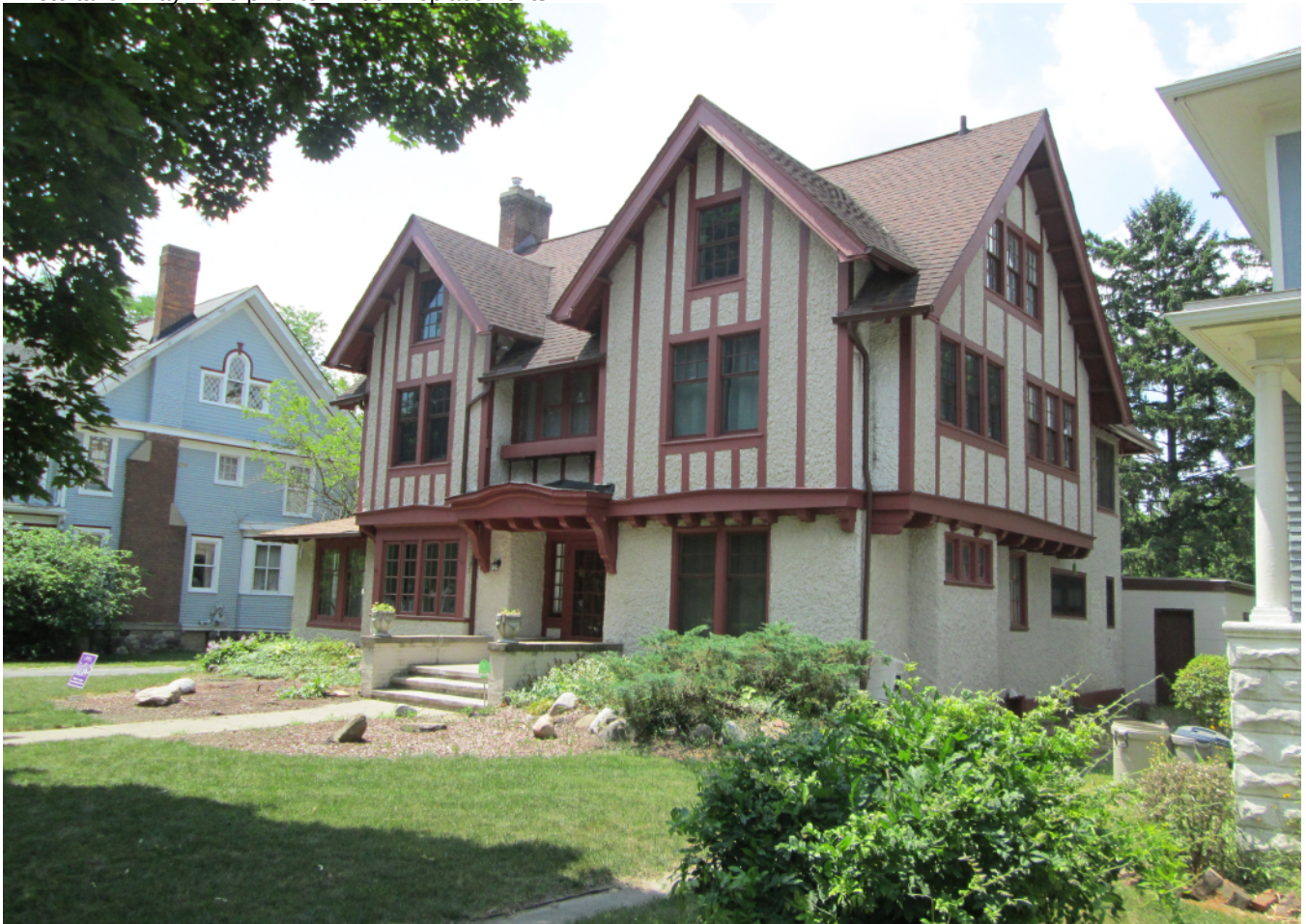
Photo taken July 2020 after window replacements.
