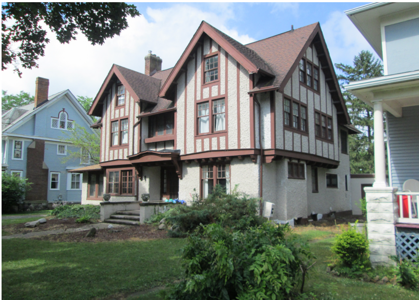
Photo taken May 2019 prior to window replacements.
