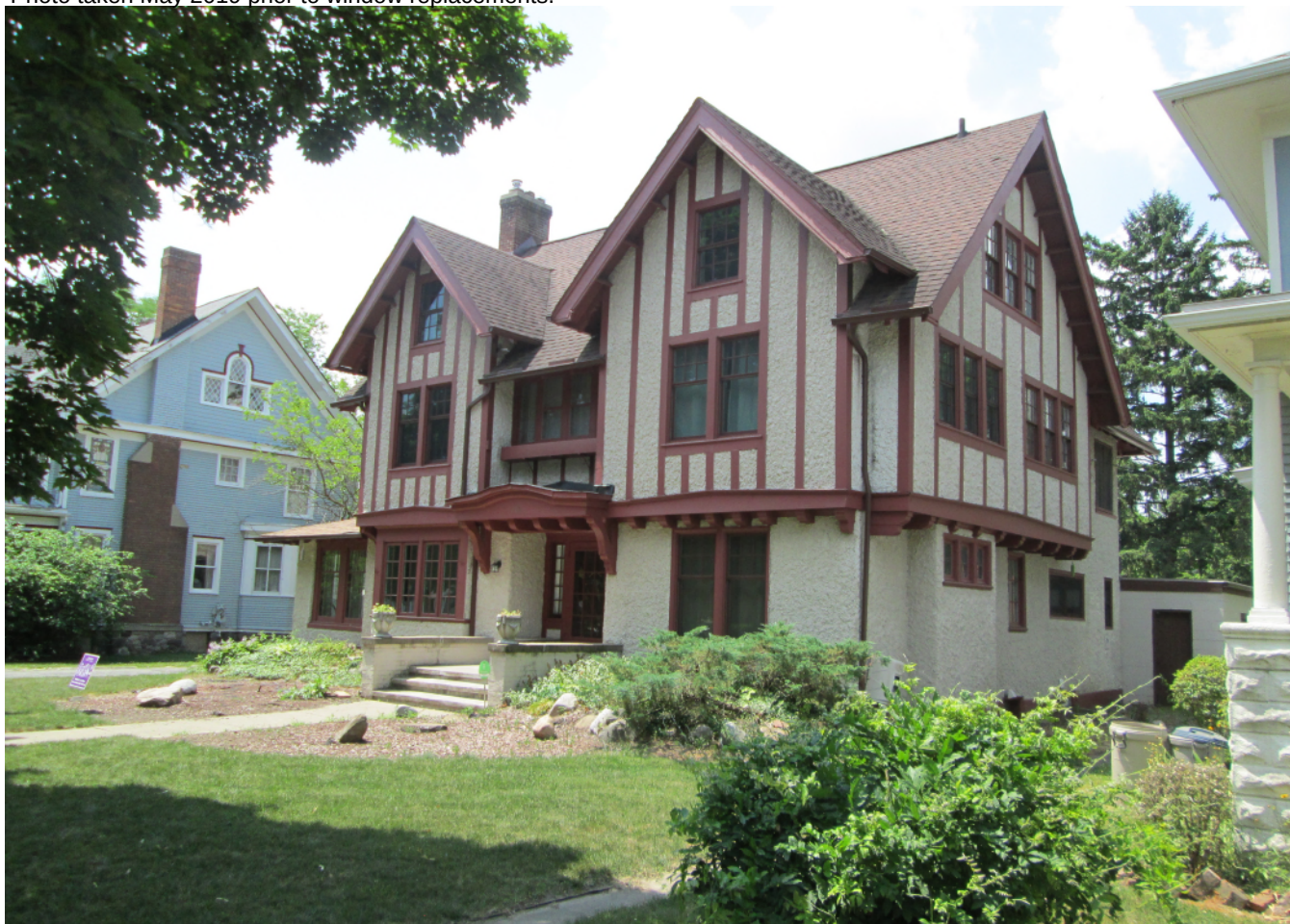
Photo taken July 2020 after window replacements.
