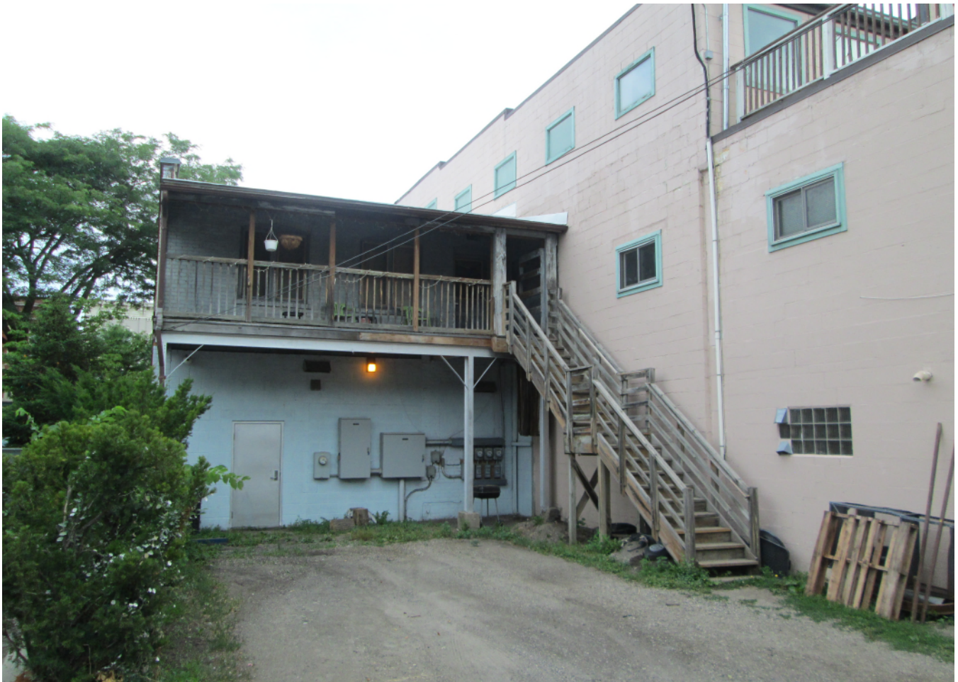
217 W Michigan, facing north-northeast to south elevation
