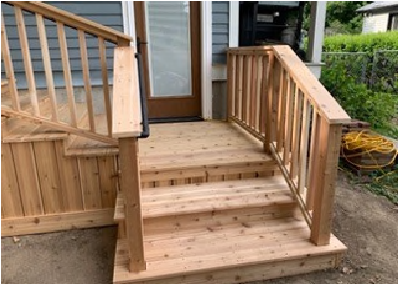
Sample deck boards and balustrade.
