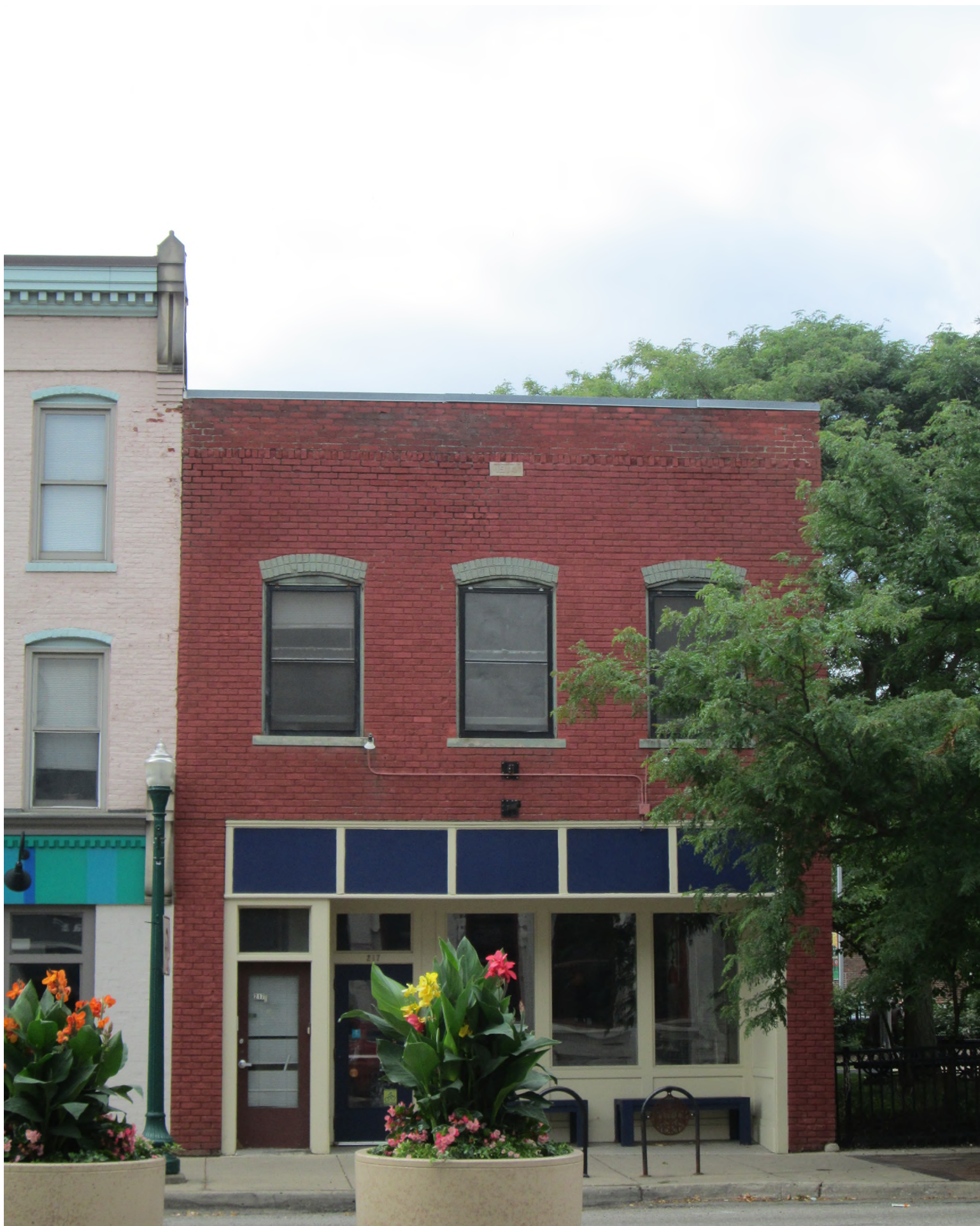
217 W Michigan, facing south to facade (for reference)
