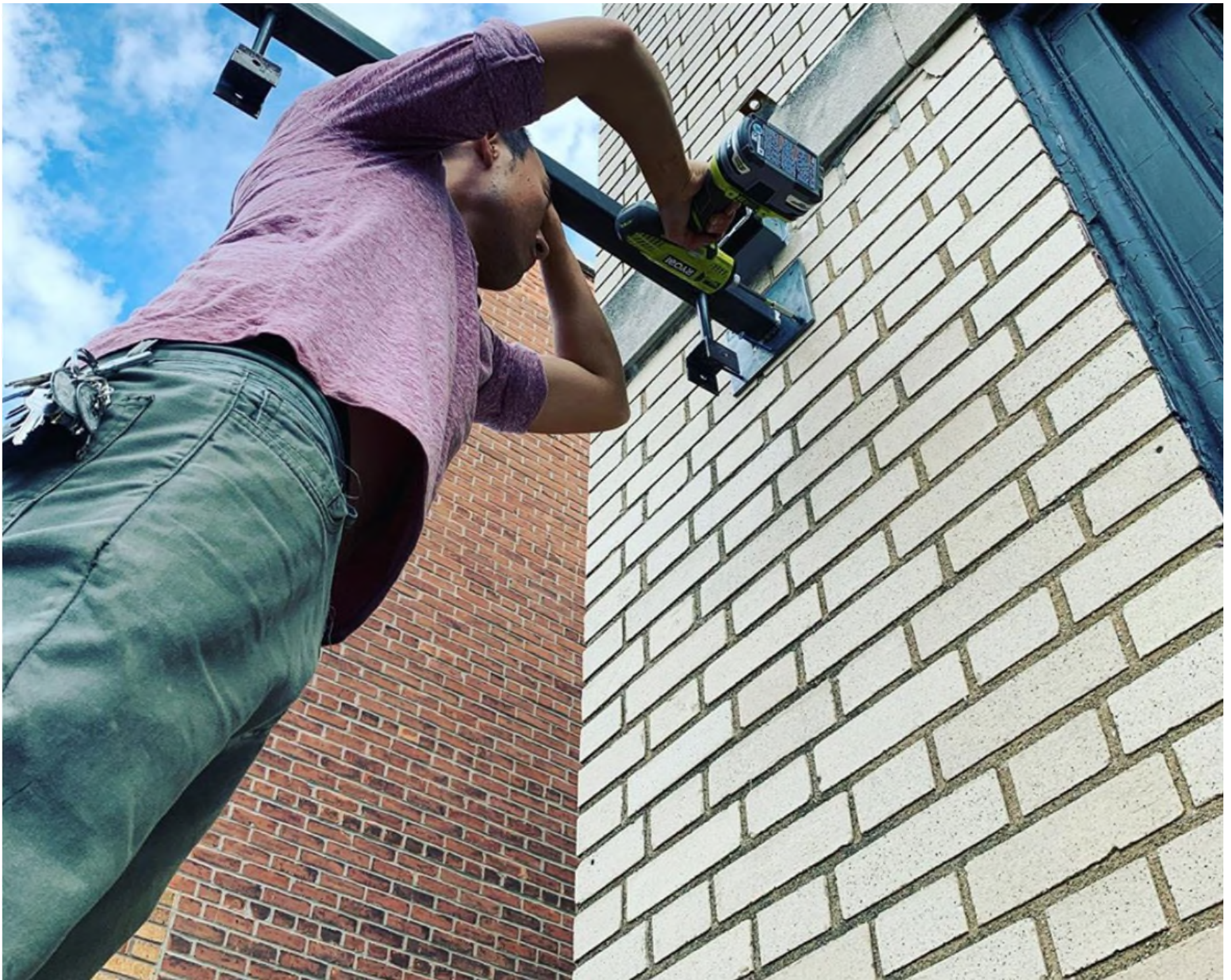
Facing southeast to installed bracket.
