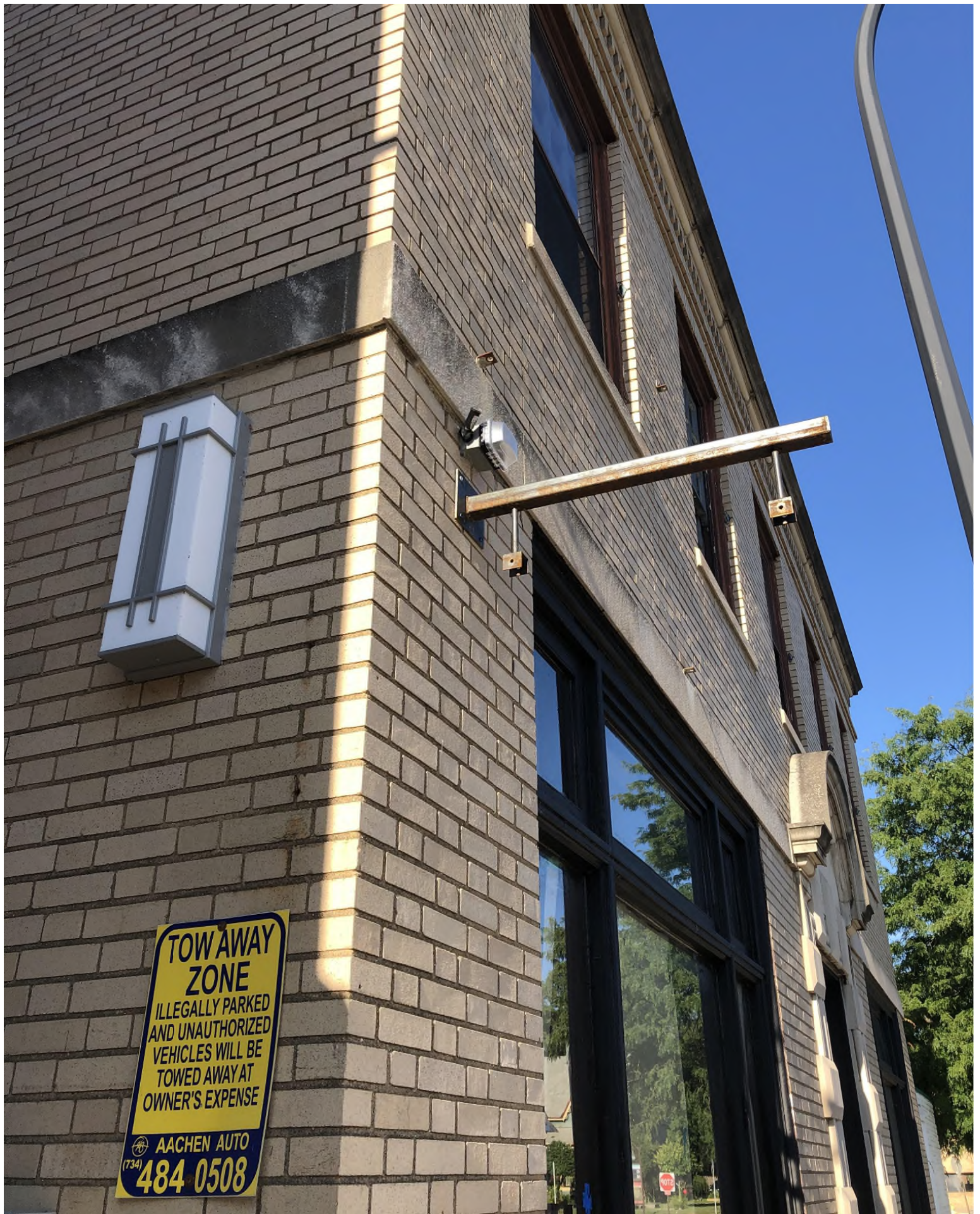
Facing southwest to installed bracket.
