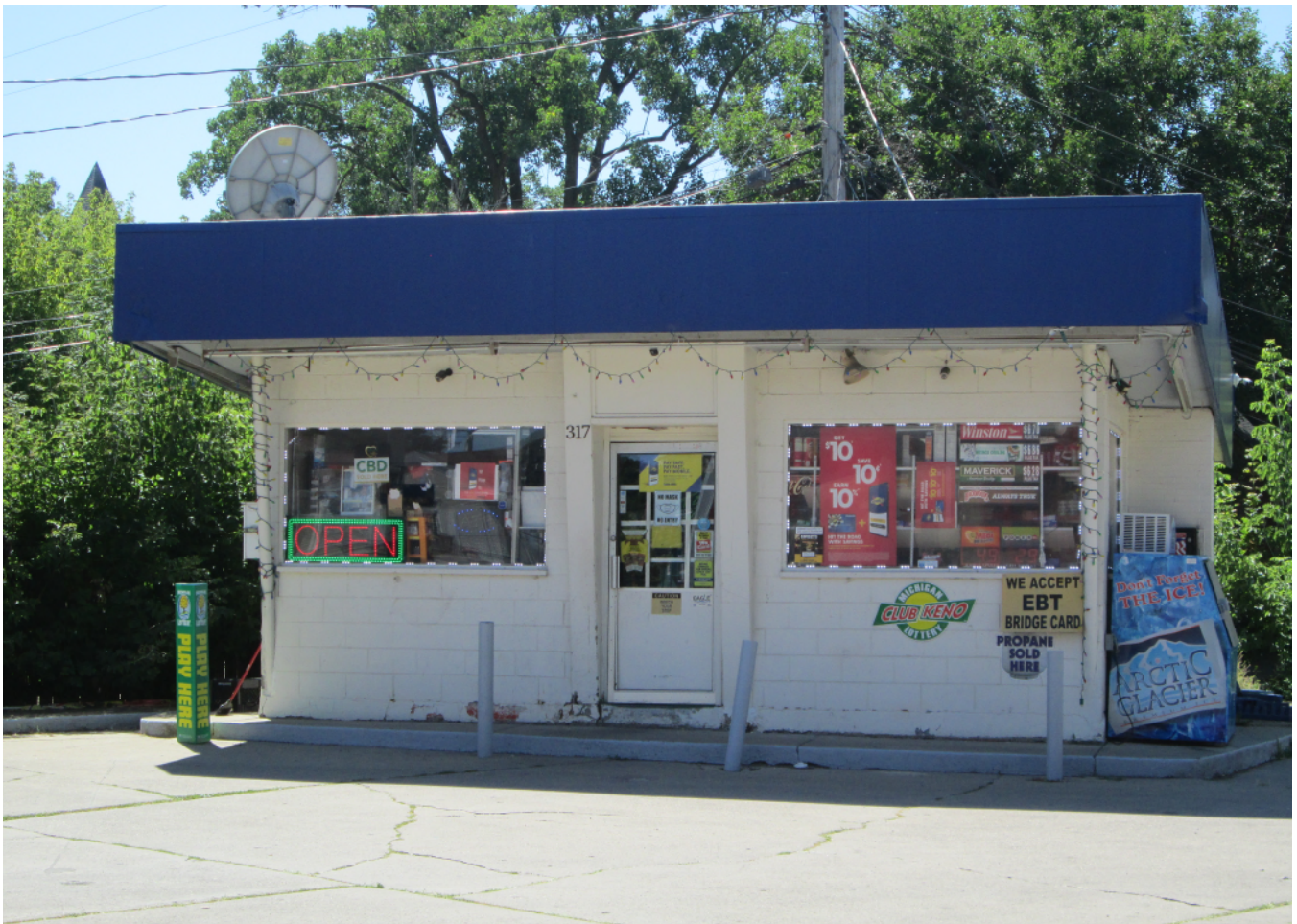
Facing southwest to building.
