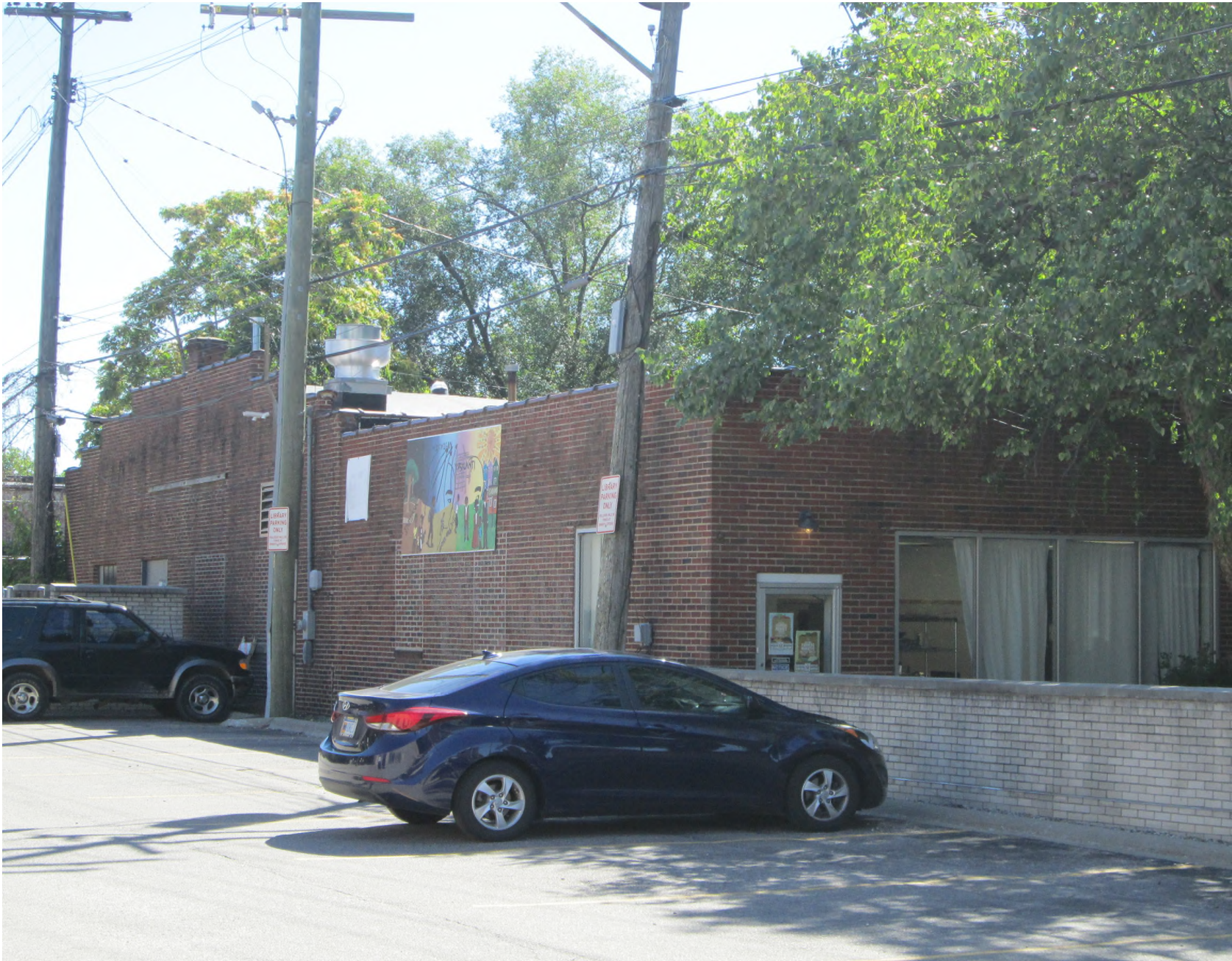
Facing southeast to facade and north elevation.
