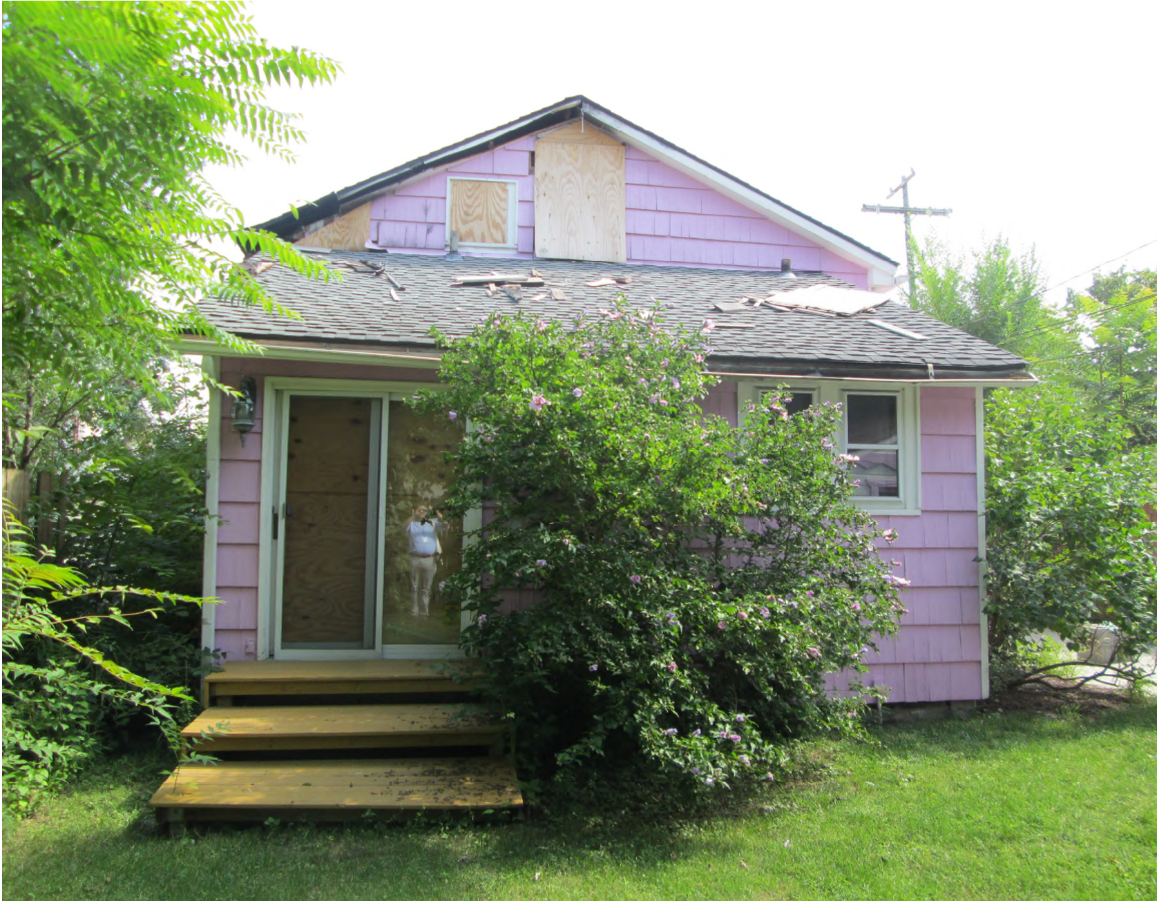
Facing east to west elevation
