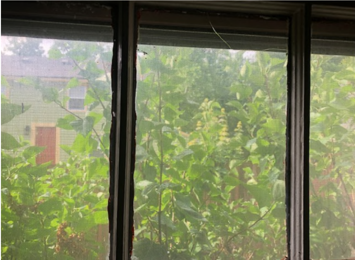
Kitchen windows- south elevation.
