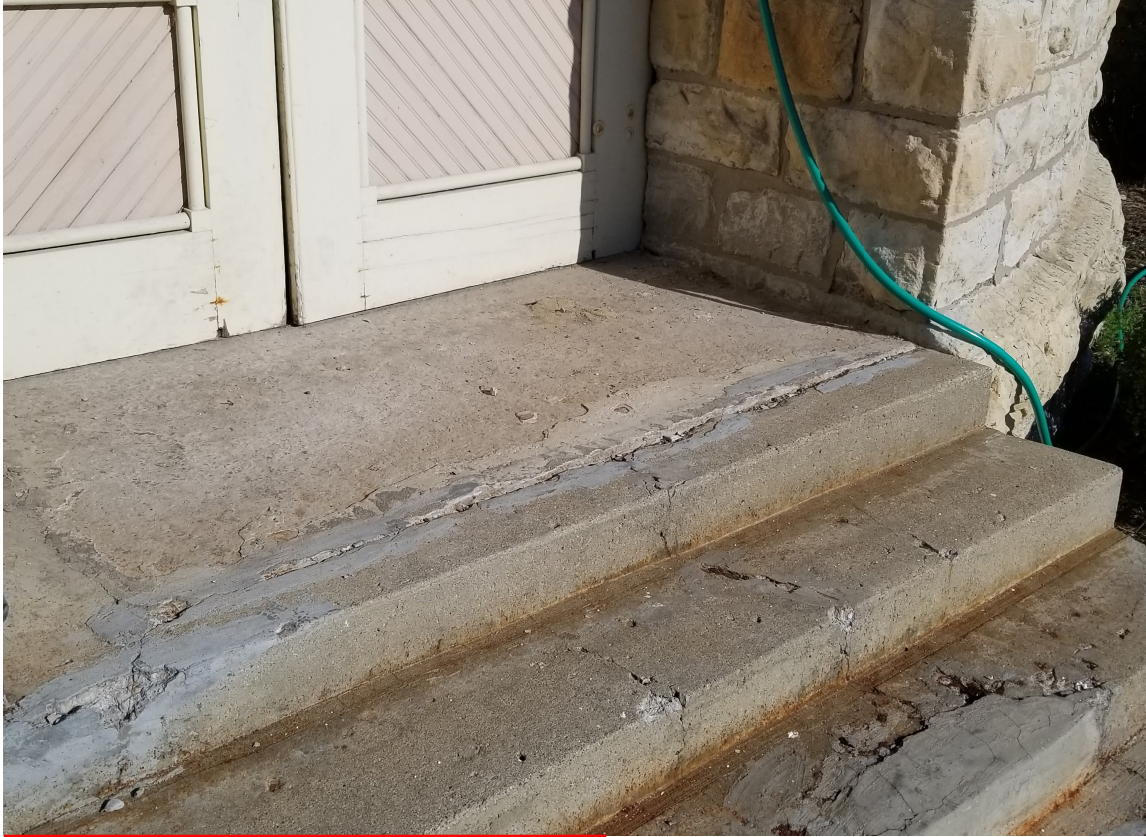
Concrete steps on the east side of Stone Tower
