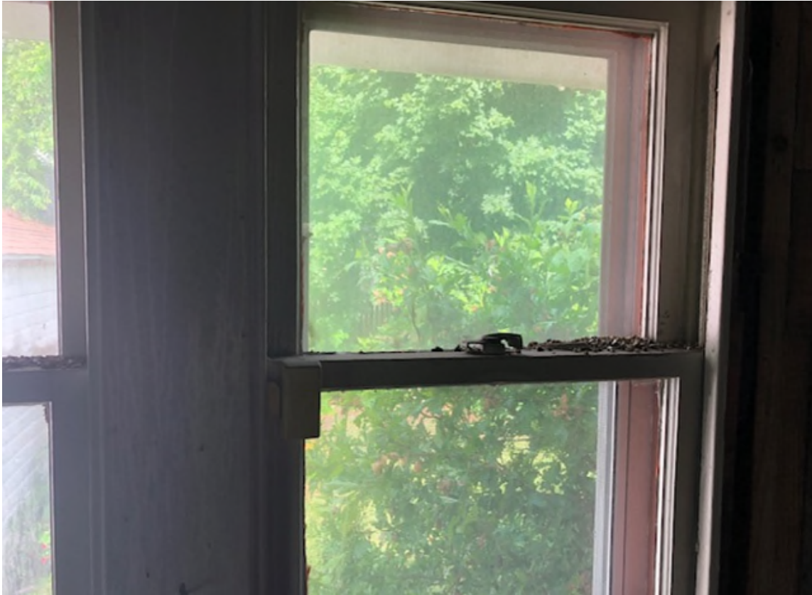
West Elevation, First Story Windows
