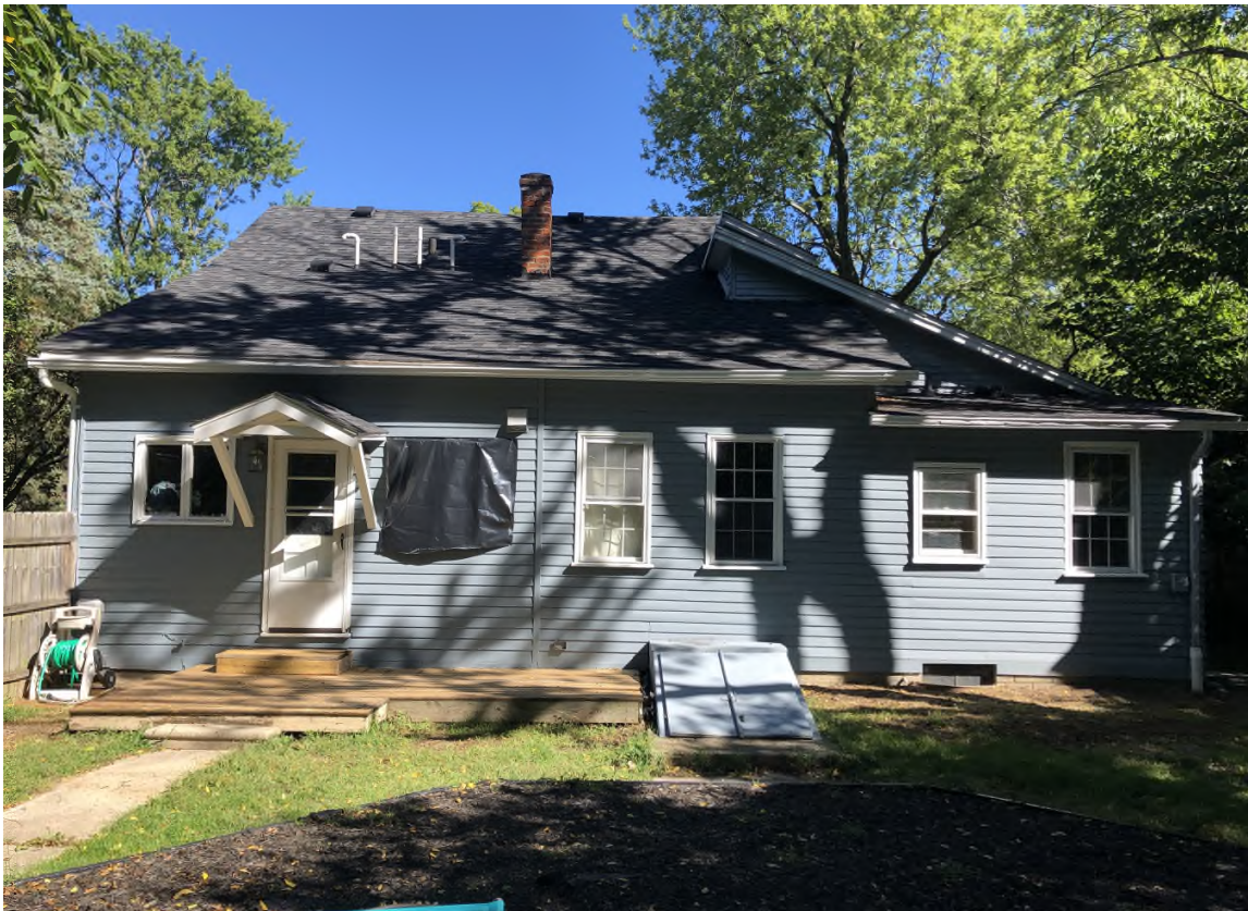
Facing north to south elevation. Window to be replaced is to the right of the door, to match the casement window to the left of the door.
