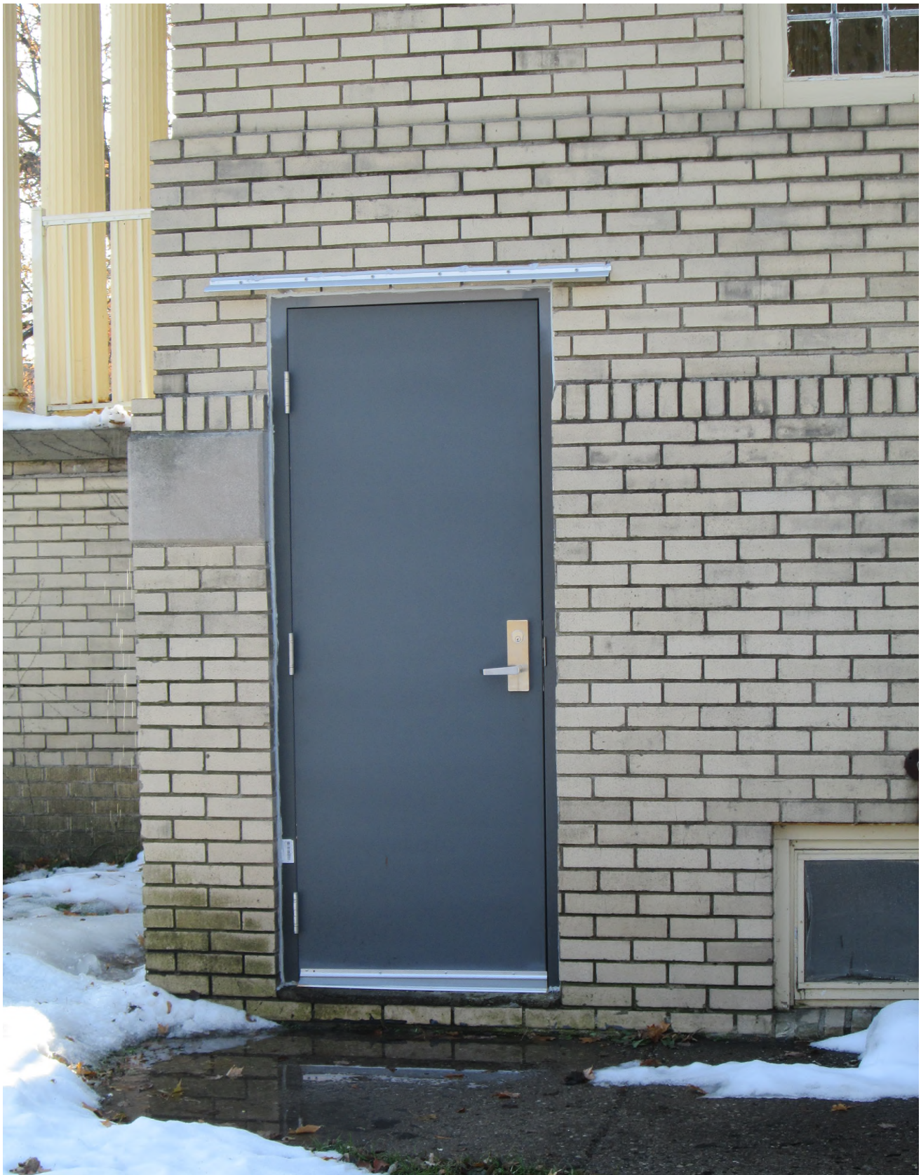
Replacement door as identified in property monitoring, November 2019.
