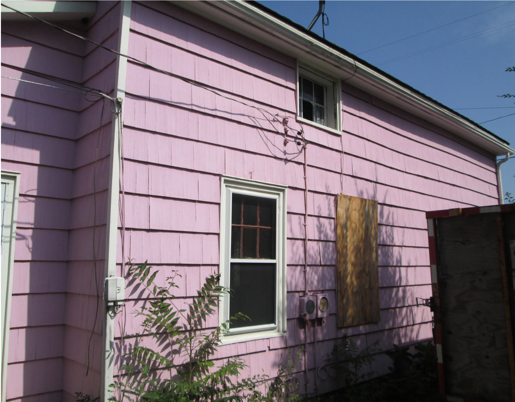
Facing north-northeast to south elevation.
