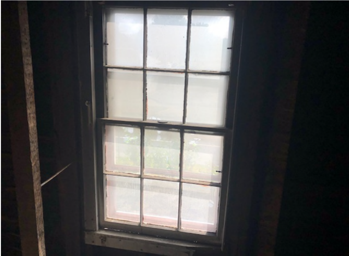
Facade second story windows. (Hallway)
