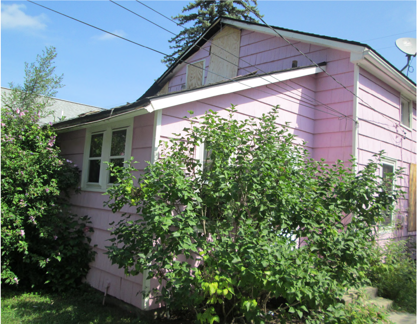
Facing northeast to south and west elevations
