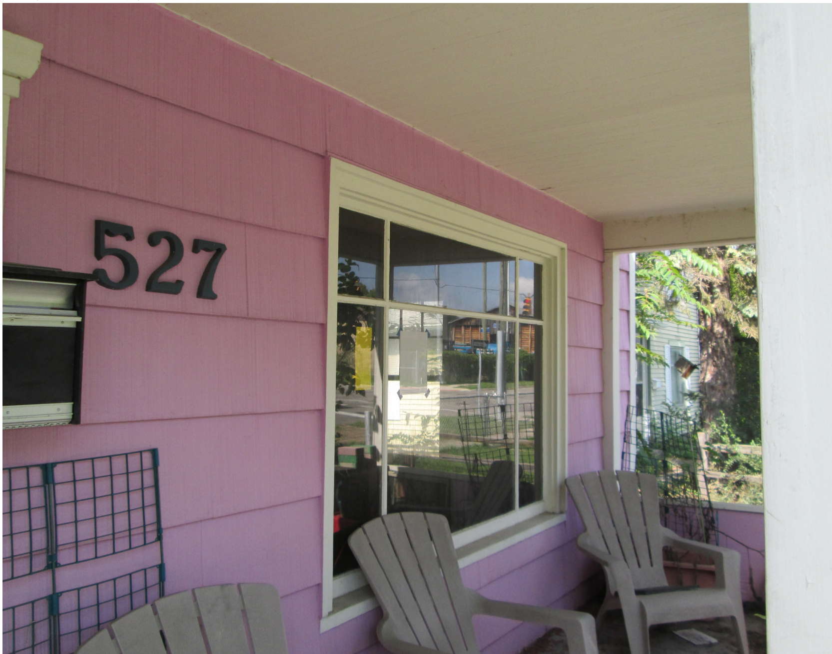
Facing northwest to facade picture window.
