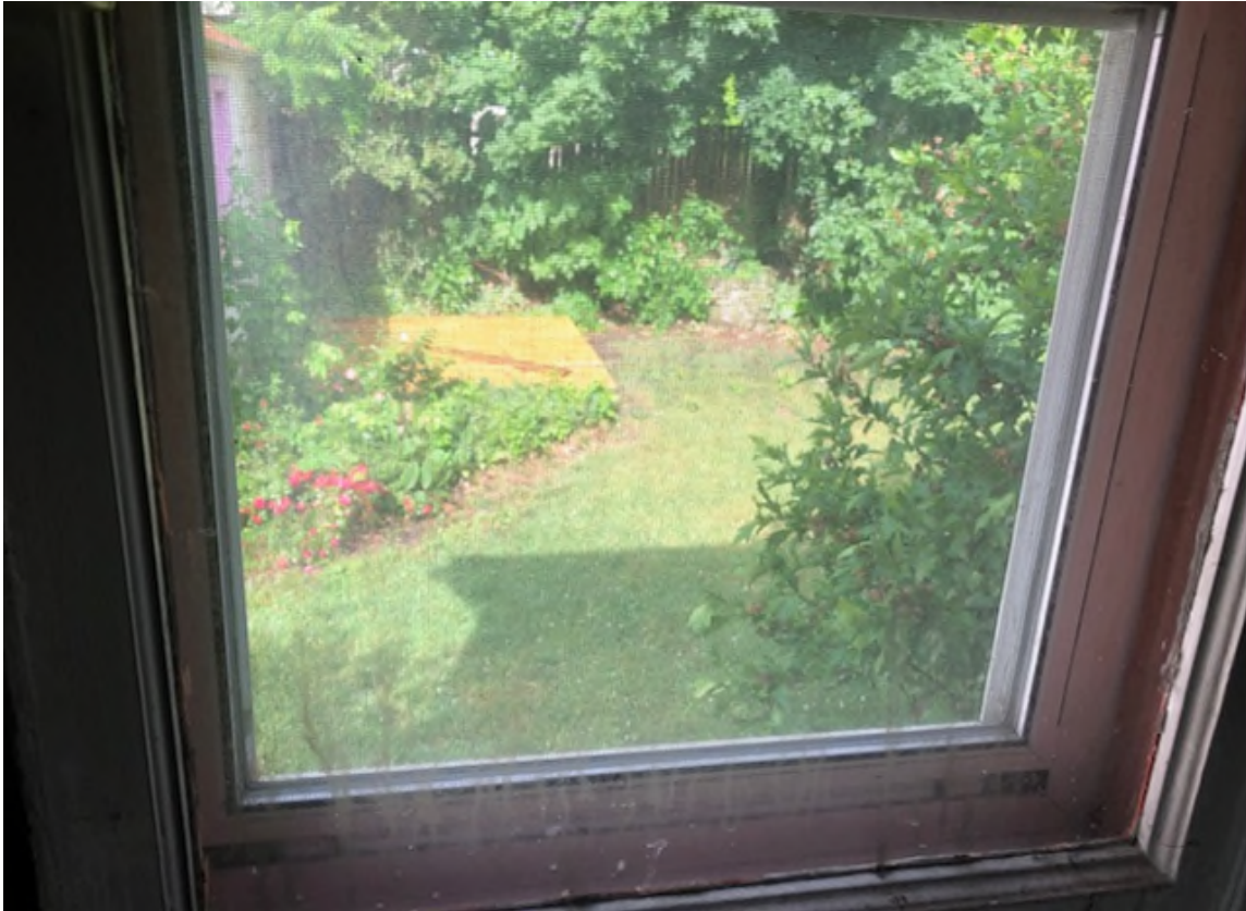
West elevation, first story windows. (Kitchen)
