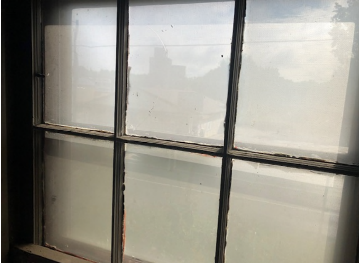
Facade second story window
