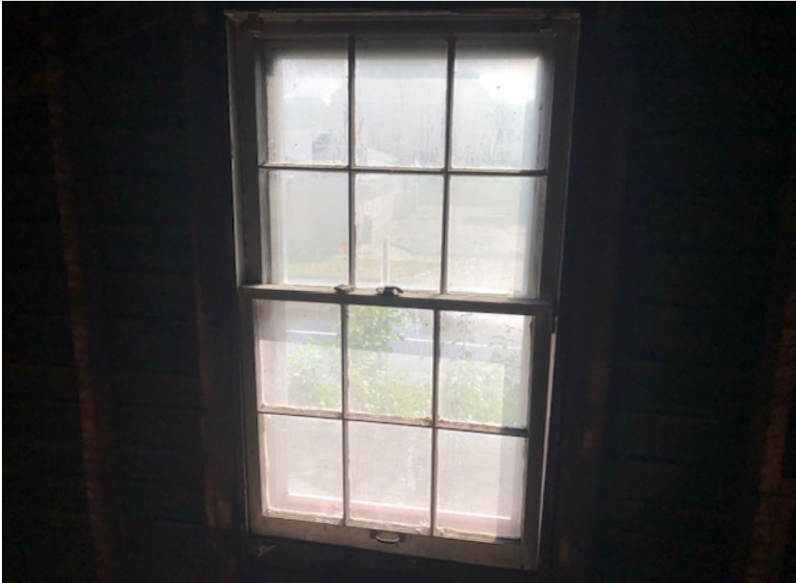
Facade second story windows (Bedroom)
