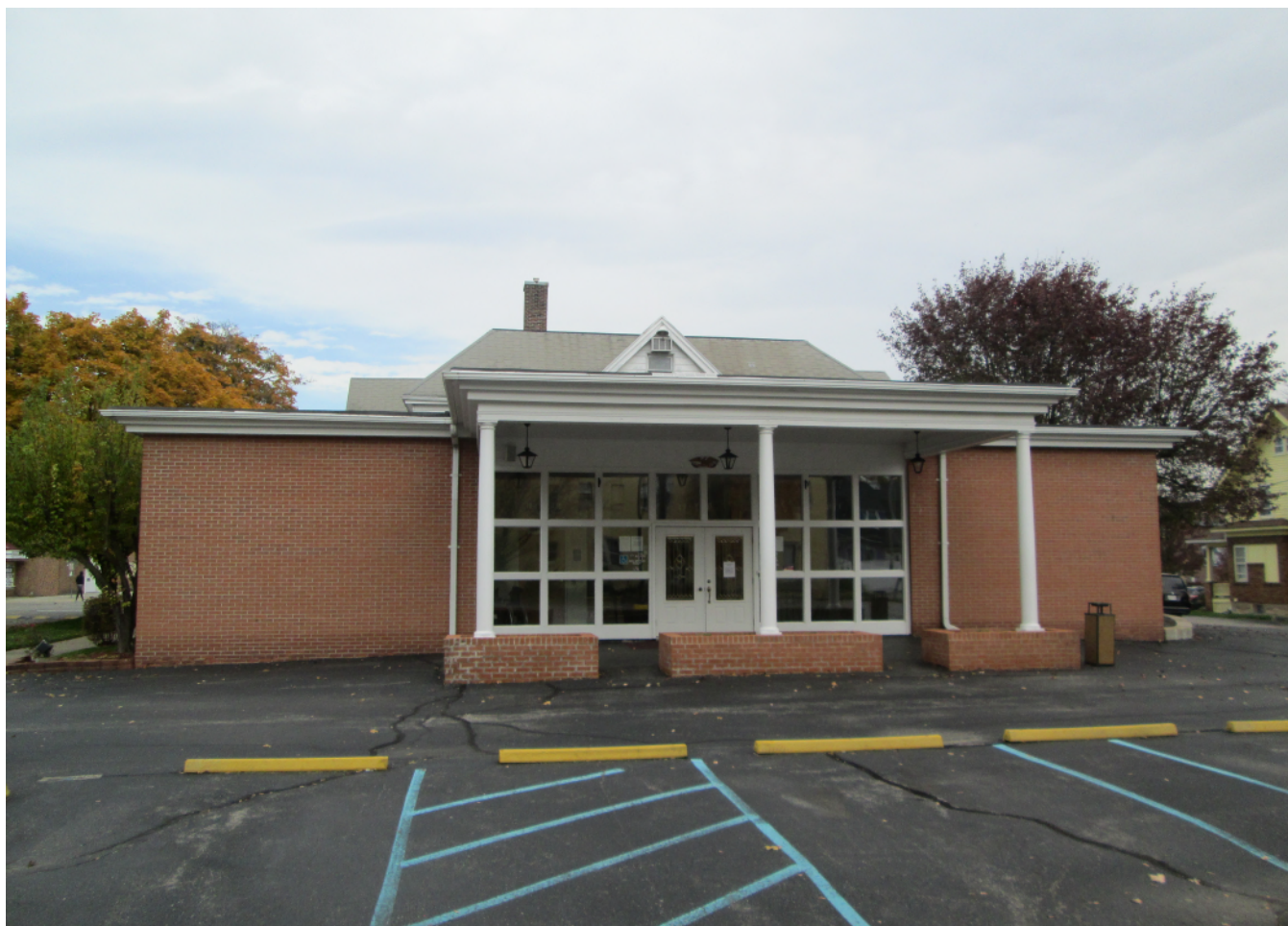
Facing north to south elevation where wall-mounted sign will go
