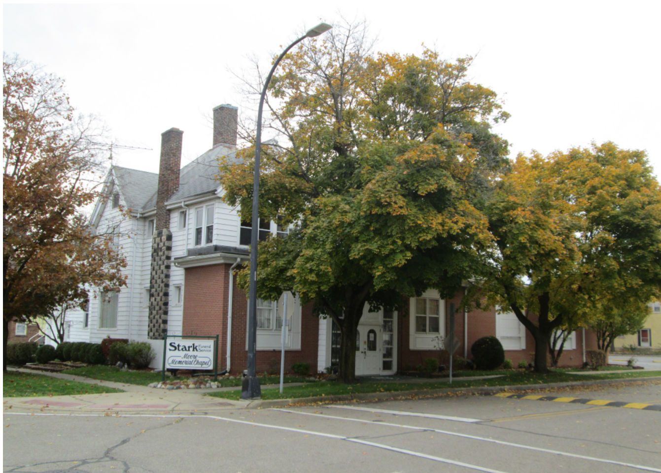
Facing southeast to property overview of facade and north elevation
