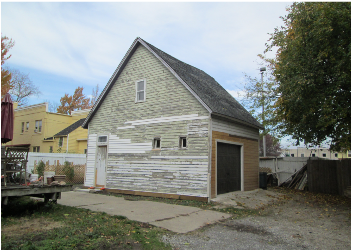
Facing northwest to south and east elevations of carriage barn
