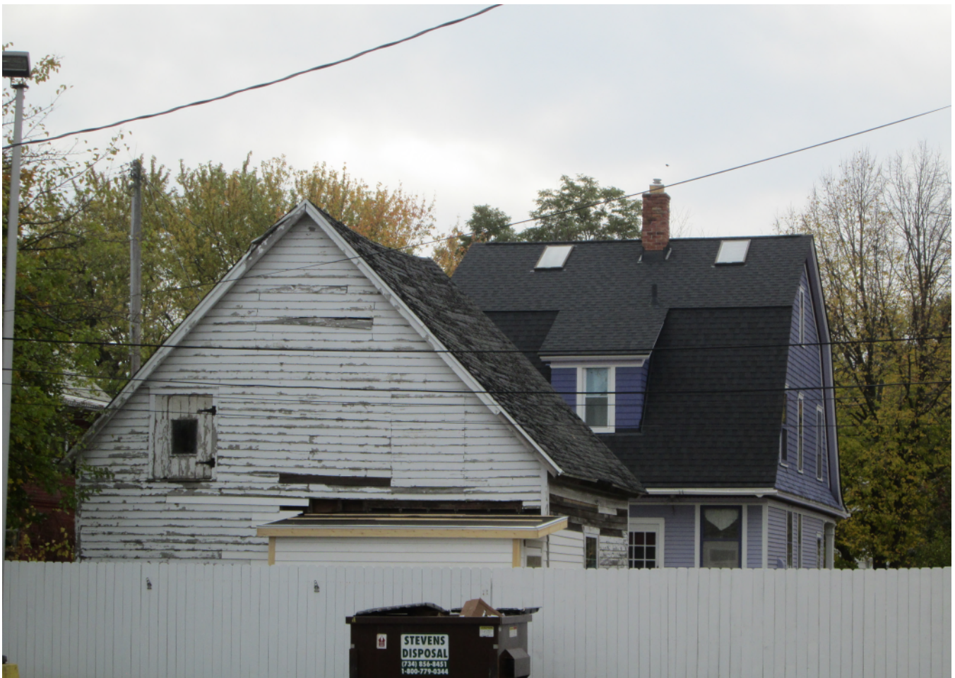
Facing south to north elevation of carriage barn.
