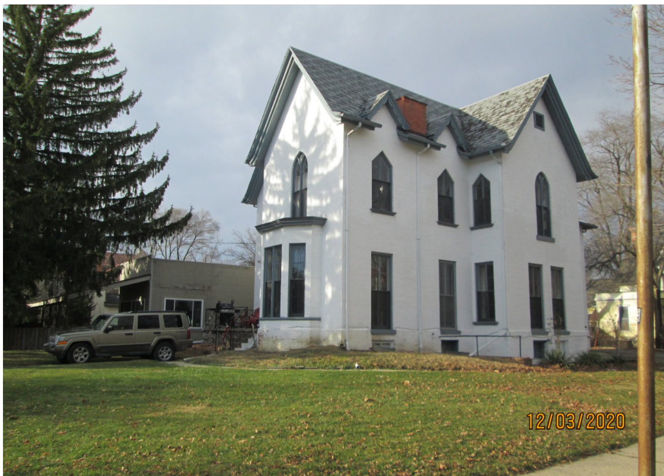
Facing northwest to 302 W Cross from light pole.
