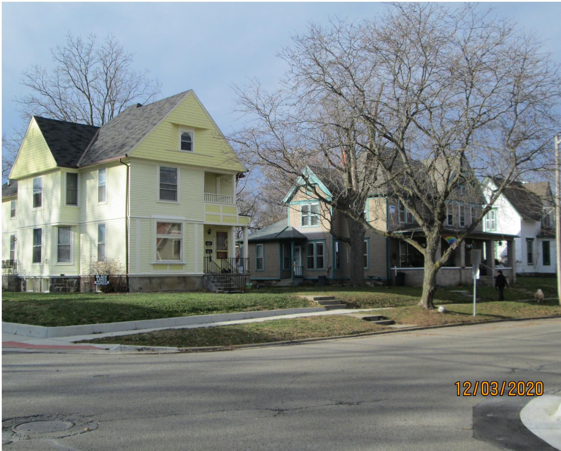
Facing northwest from light pole.
