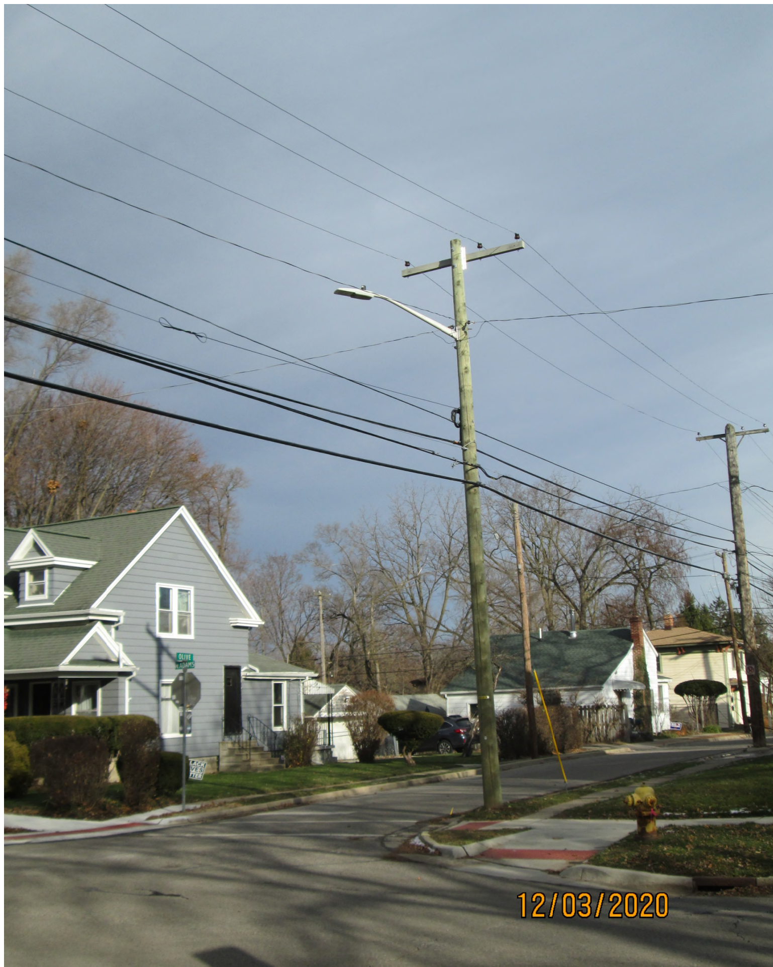
Facing northeast to light pole.
