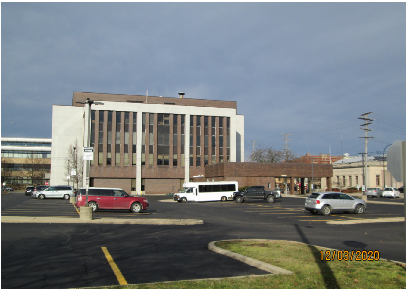
Facing northeast from light pole.
