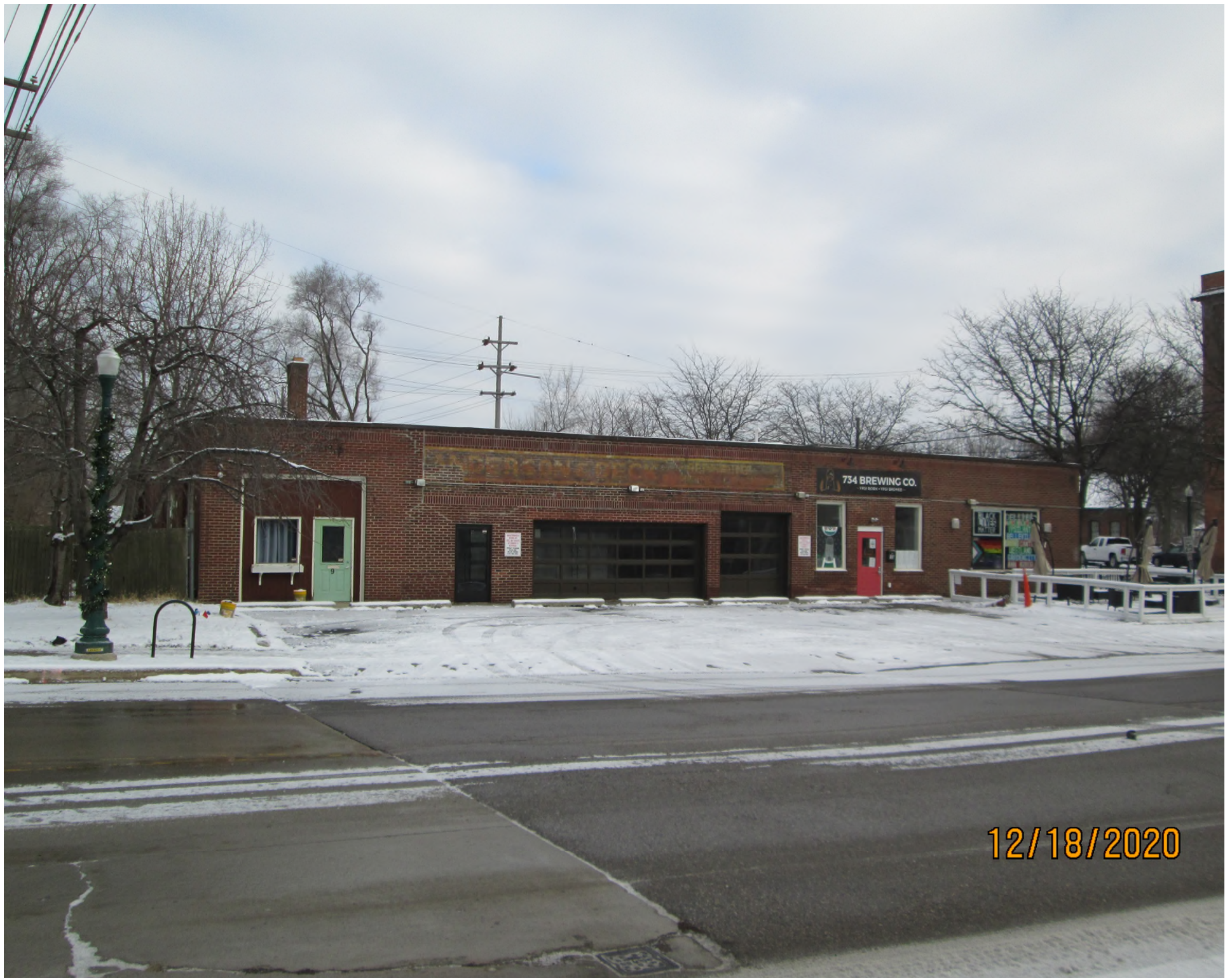
Facing north-northeast to whole building.
