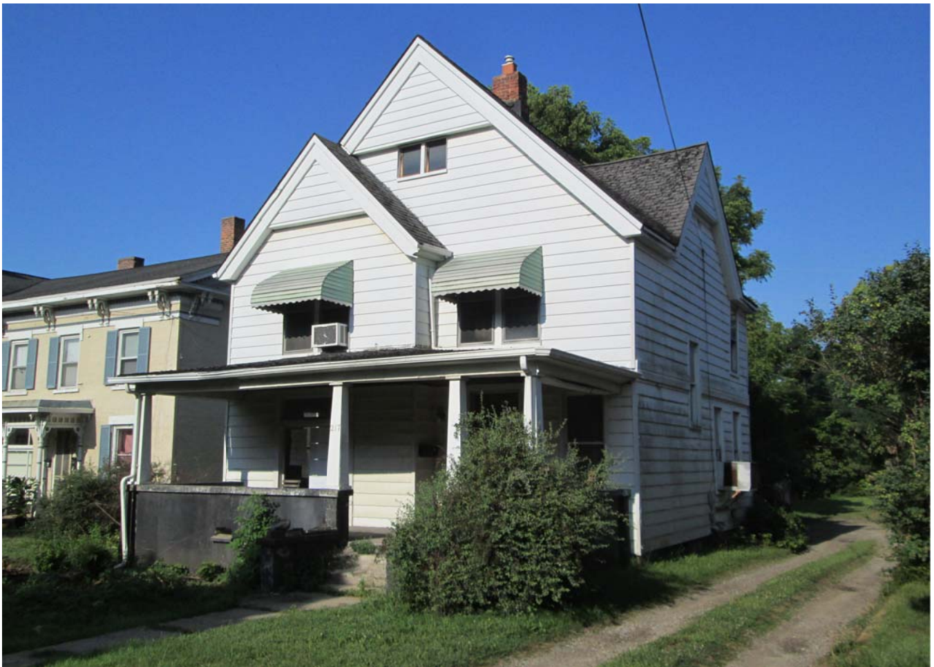
Facing southwest to facade and north elevation.
