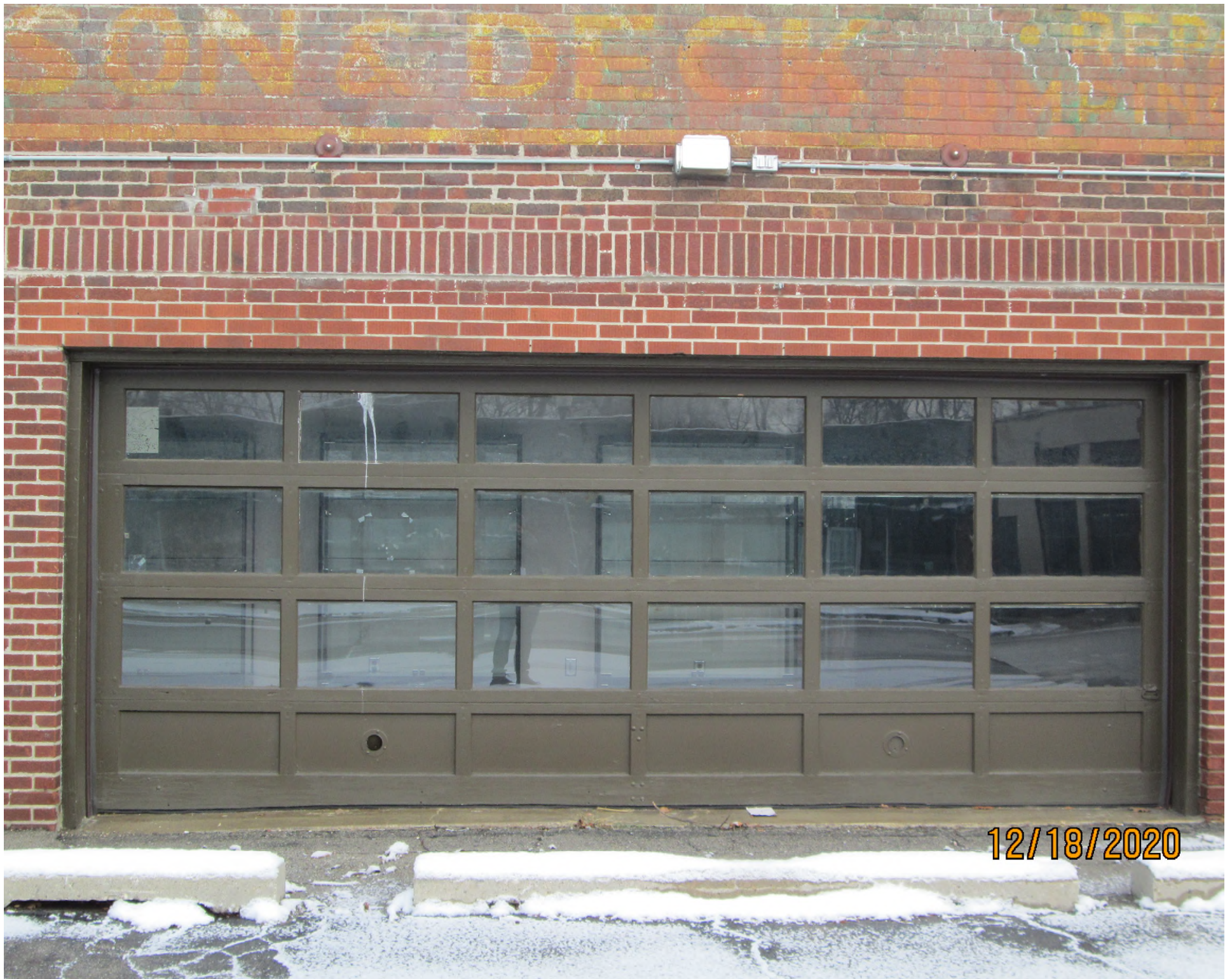
Detail of restored garage bay.
