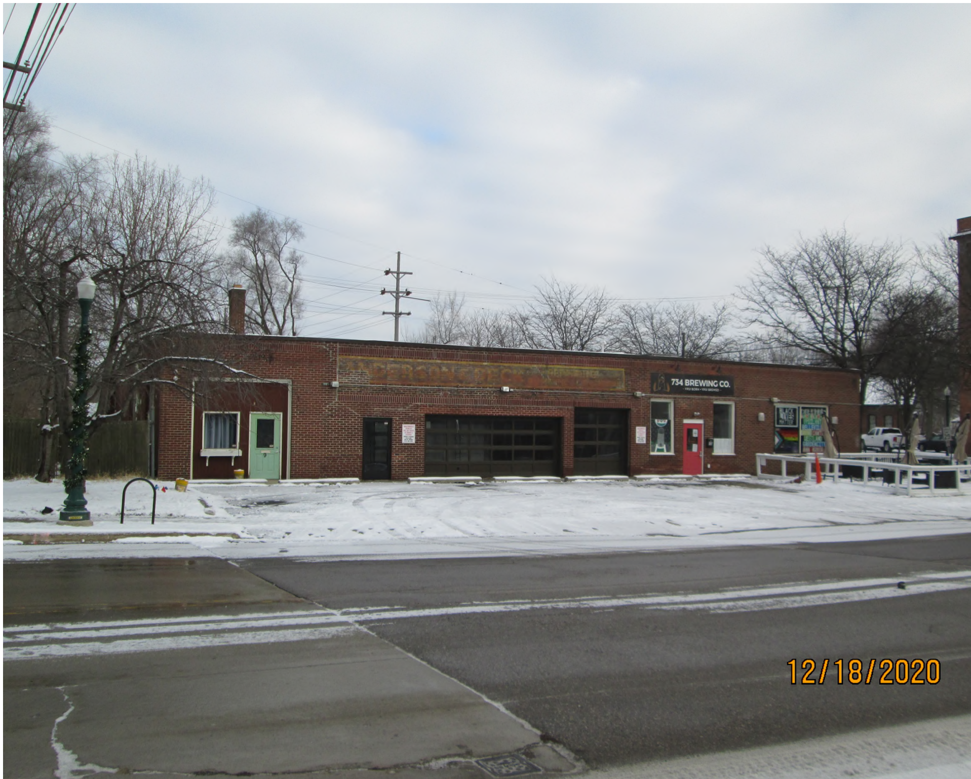
Facing north-northeast to whole building.
