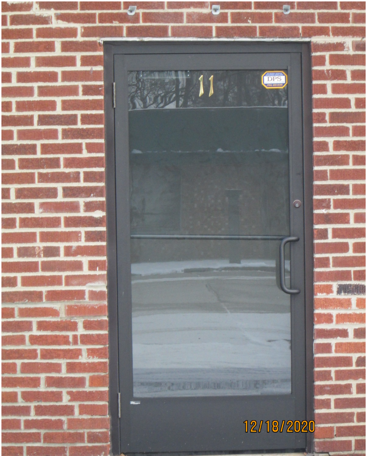
Detail of replacement door.
