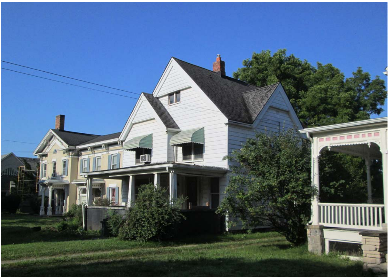
Facing southwest to facade and south elevation.
