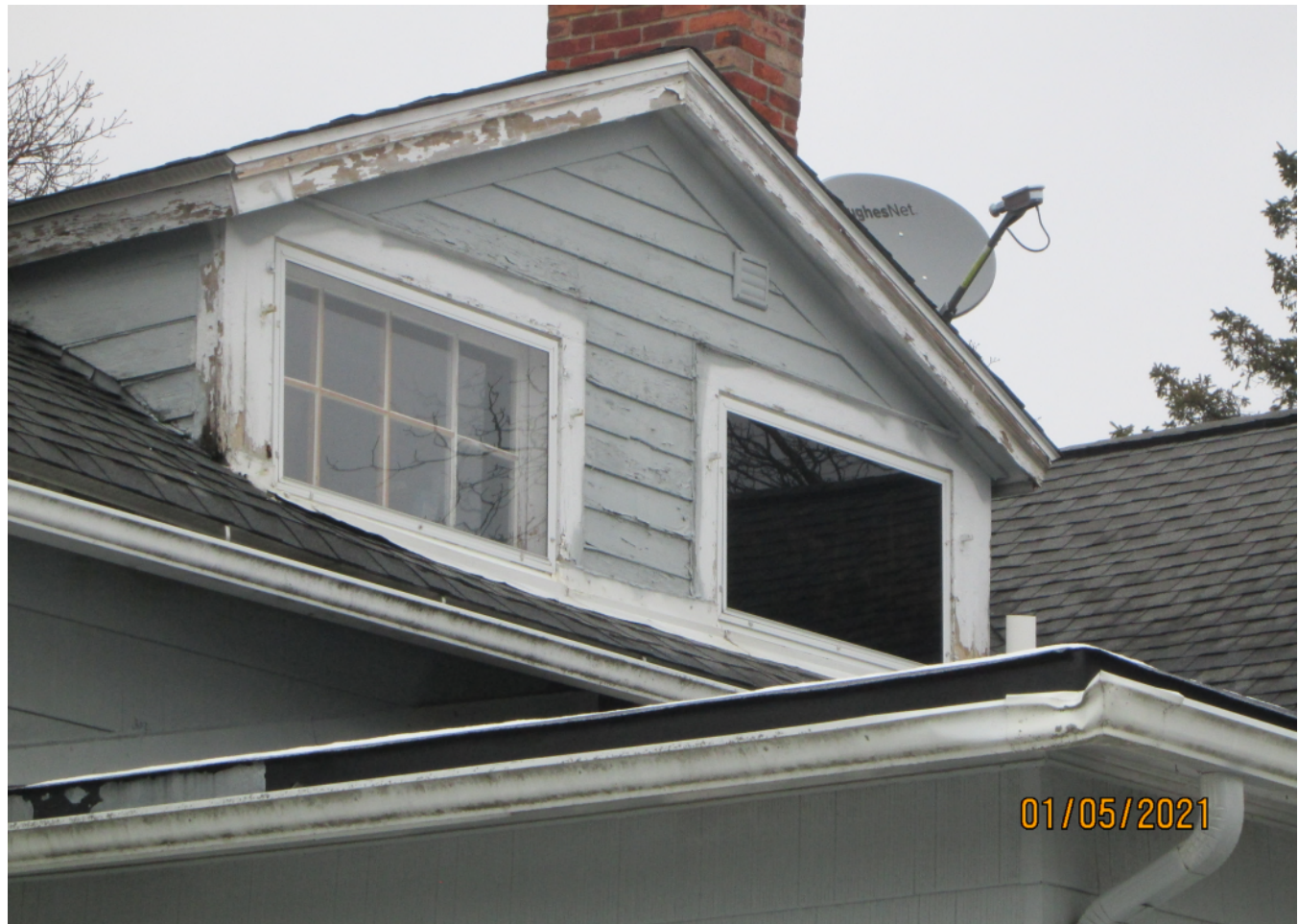
Detail of extant siding on dormer
