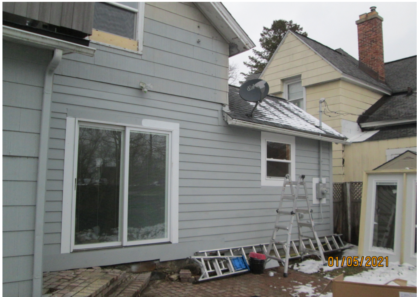
New siding on south elevation
