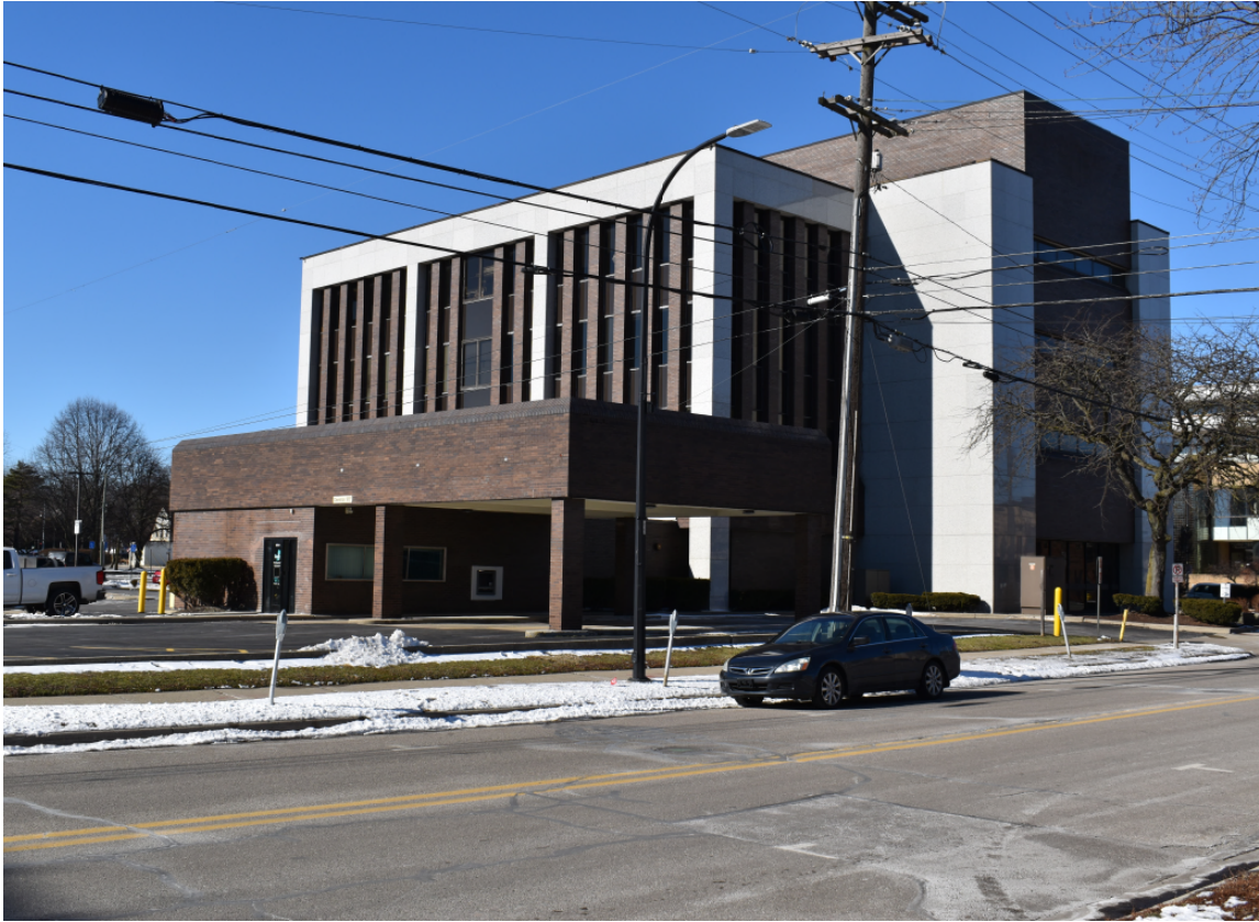
Facing northwest to drive-in section of building.
