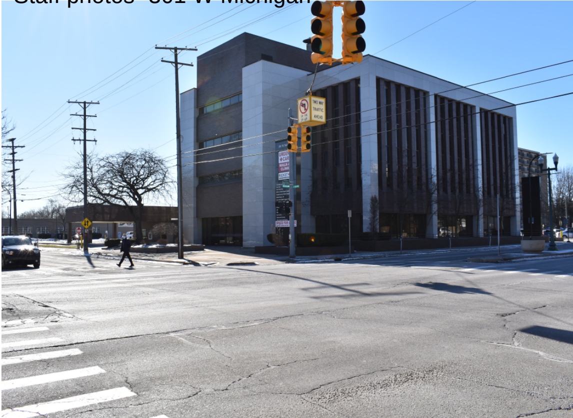
Facing southwest to facade and east elevation
