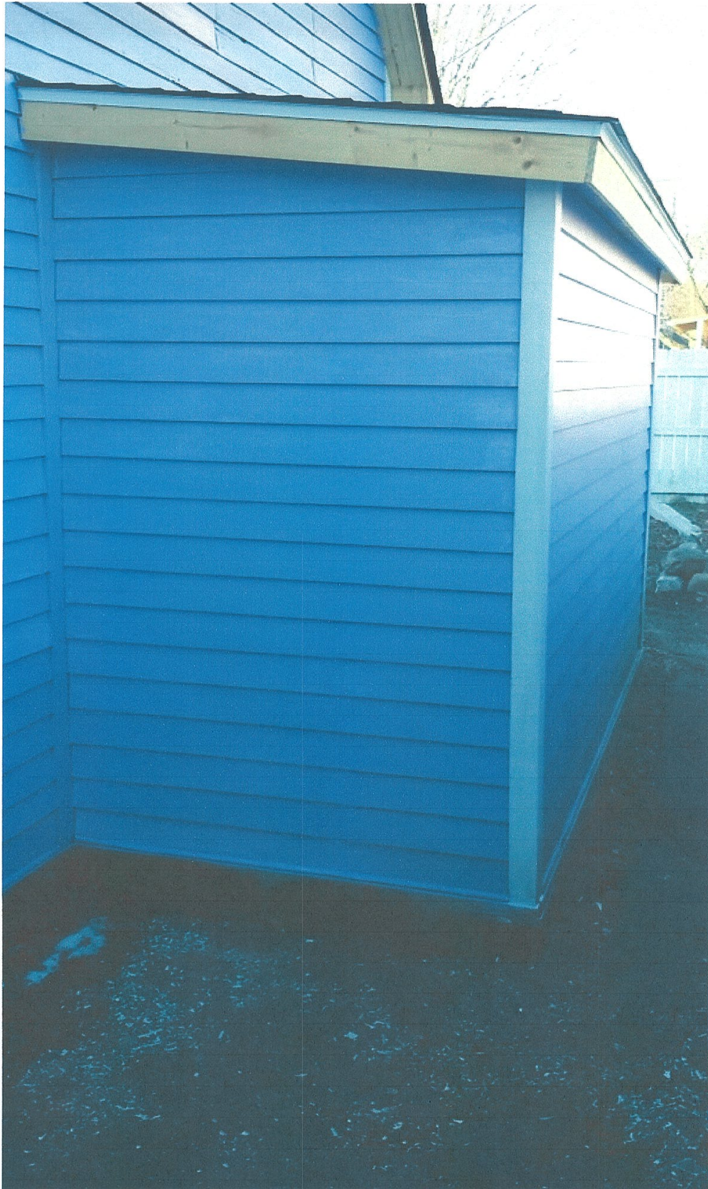
p3 East side of shed
