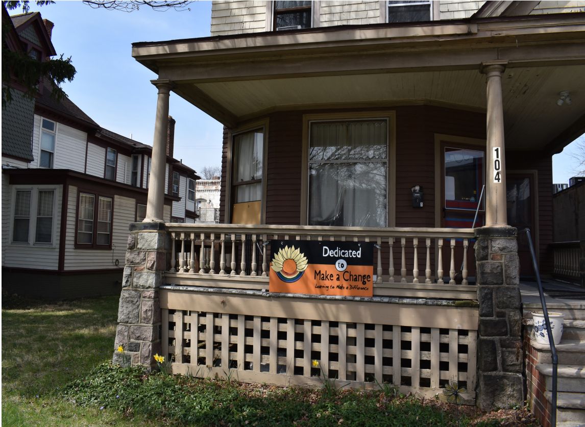
Facing west to detail of porch.
