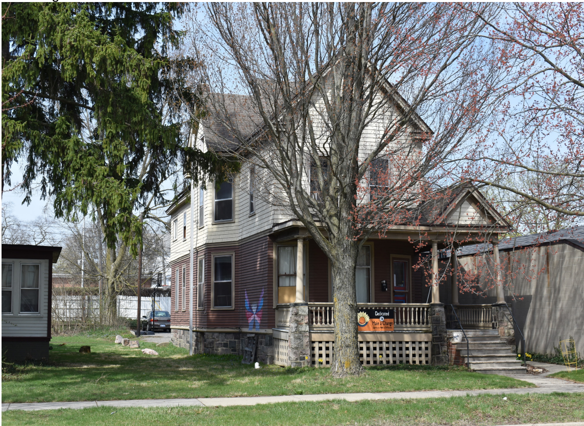
Facing northwest to facade and south elevation.
