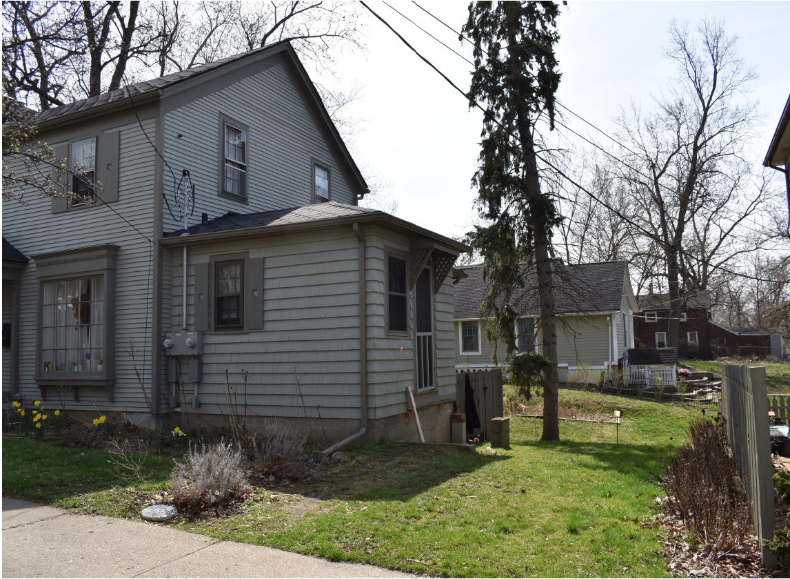
Entry porch and fence location
