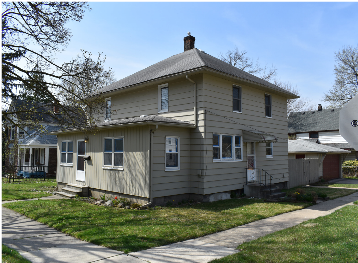
Facing southwest to facade and north elevation
