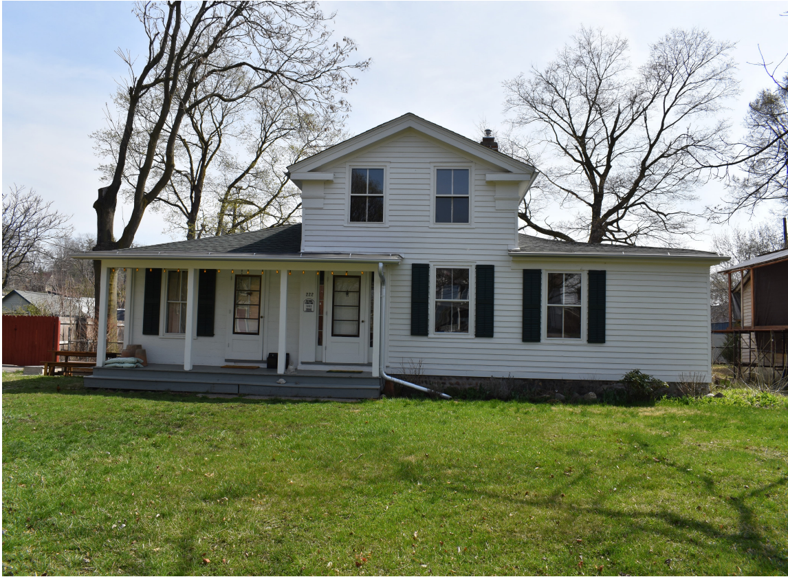
Photo of 222 N River Facade from right-of-way.
