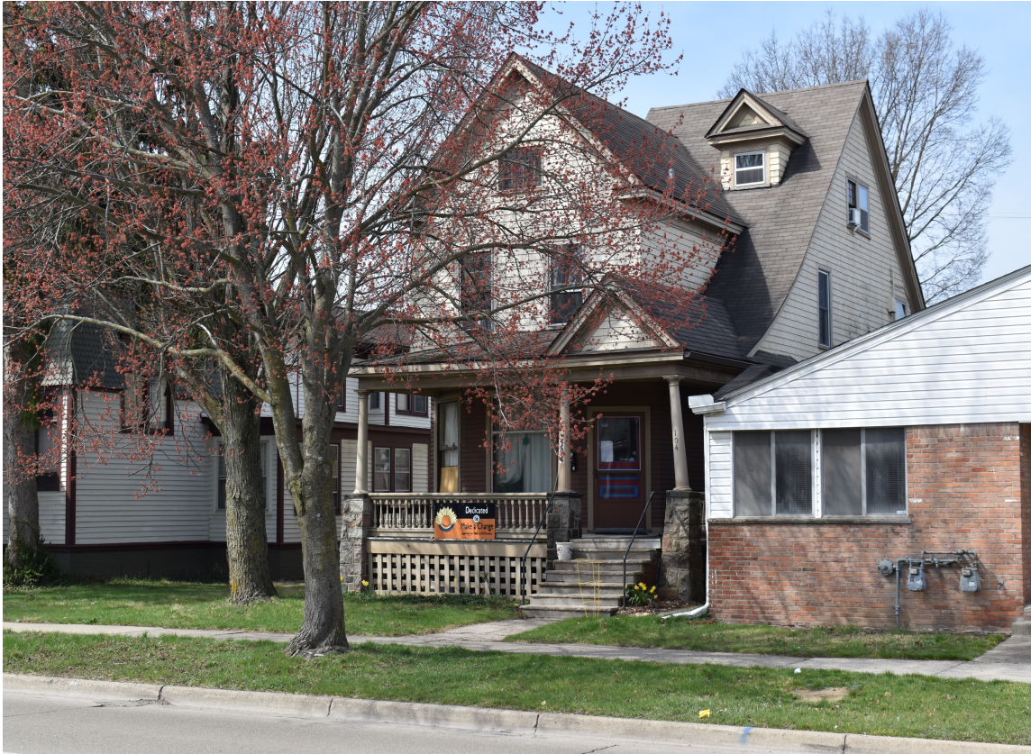
Facing southwest to facade and north elevation.
