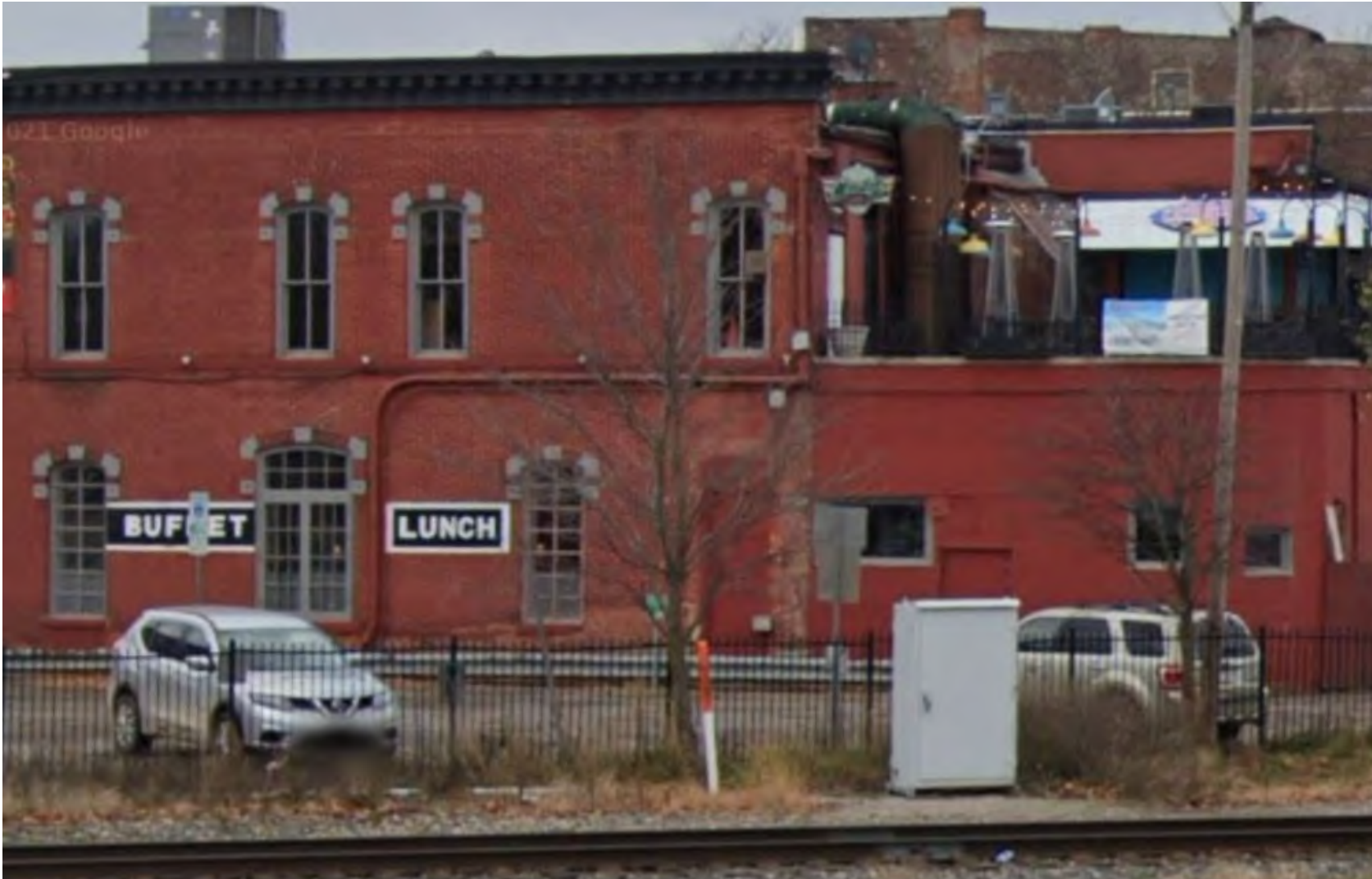
Photo from Google Street-View showing the roof-top dining area in 2020. View facing west from N River.
