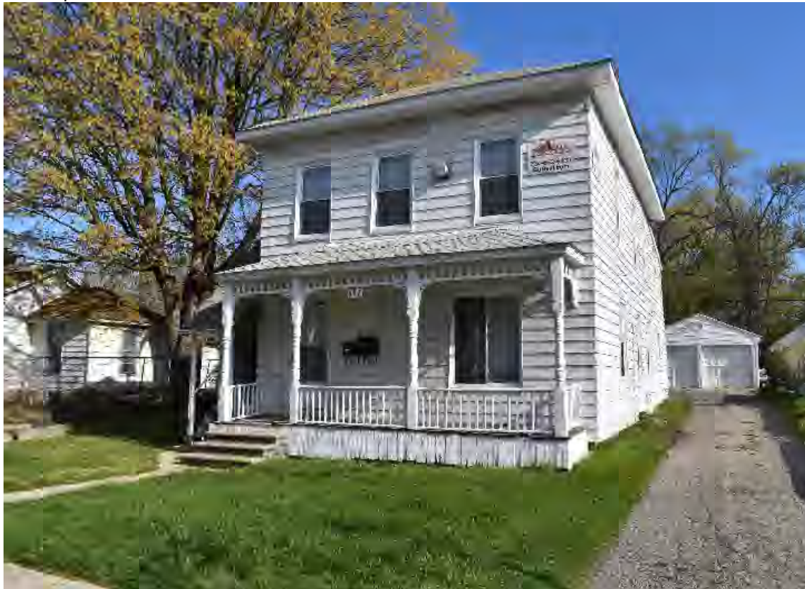
Facing northwest to facade and east elevation.
