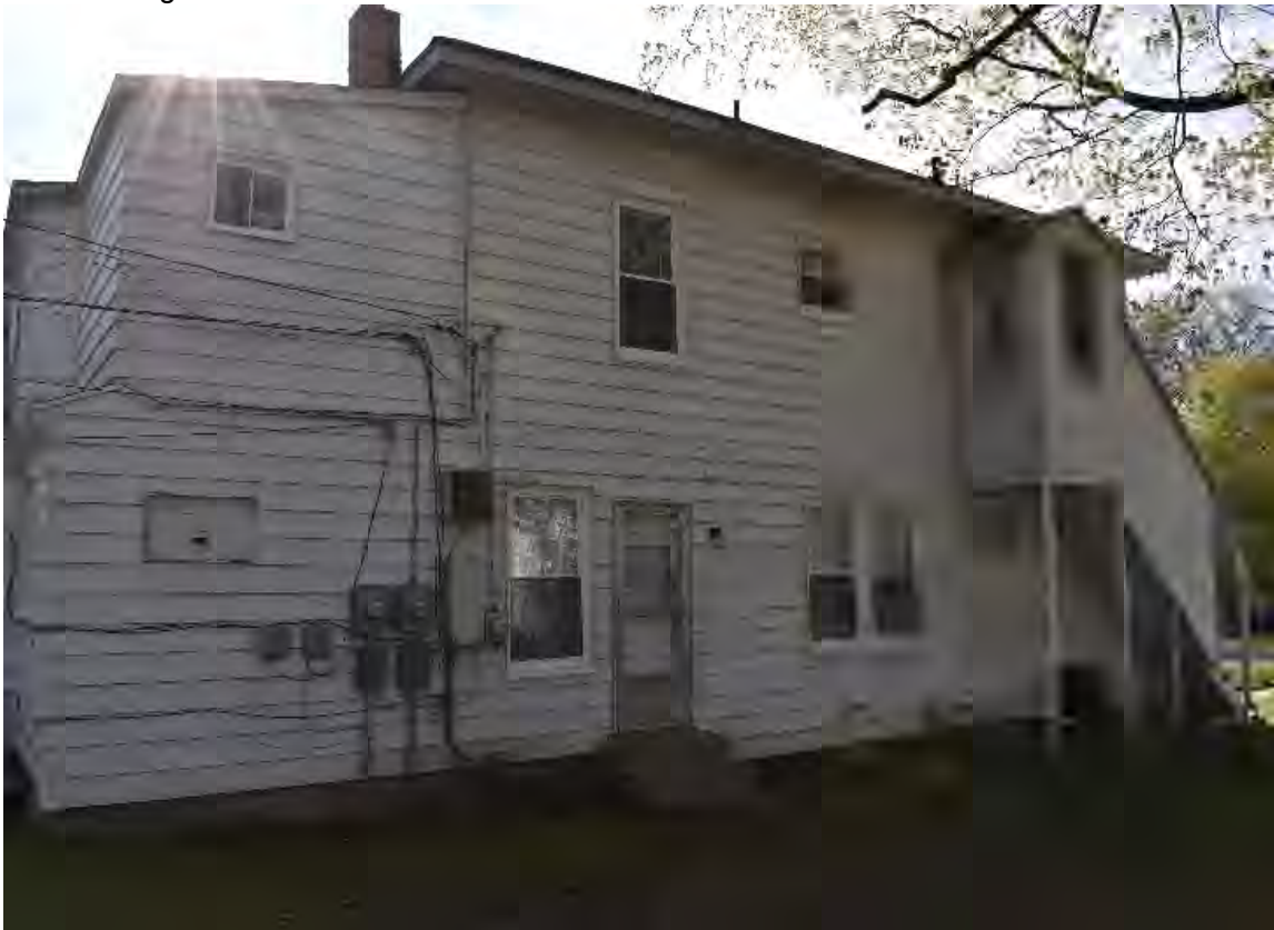
Facing southeast to west elevation.
