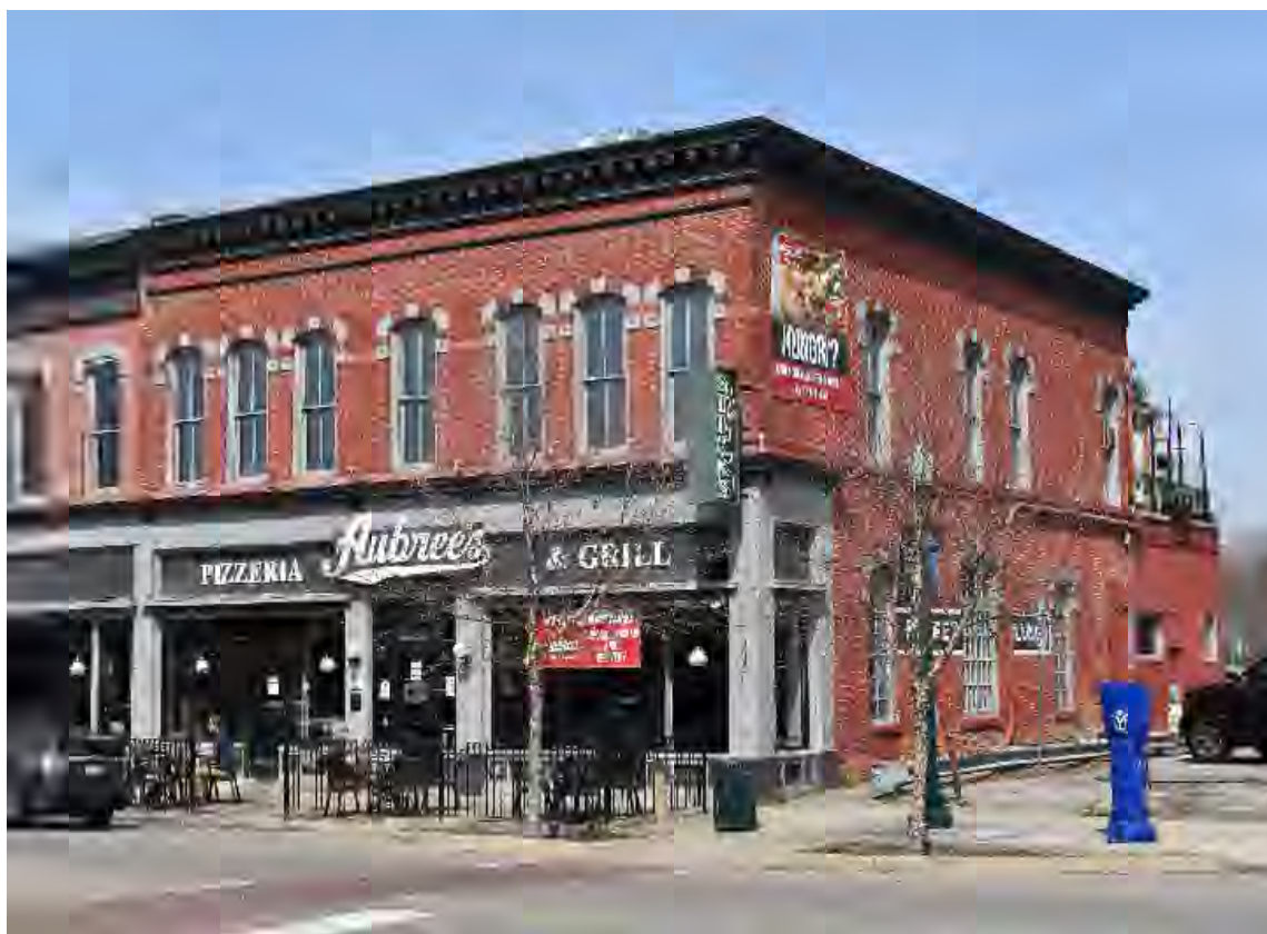
Staff photos of 39 E Cross. Above, facing northwest to facade and east elevation. Patio at rear.
