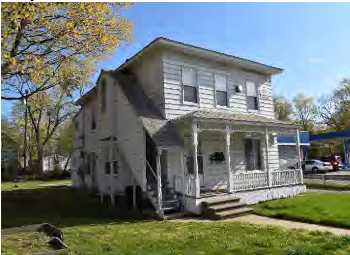
Facing northwest to facade and west elevation.
