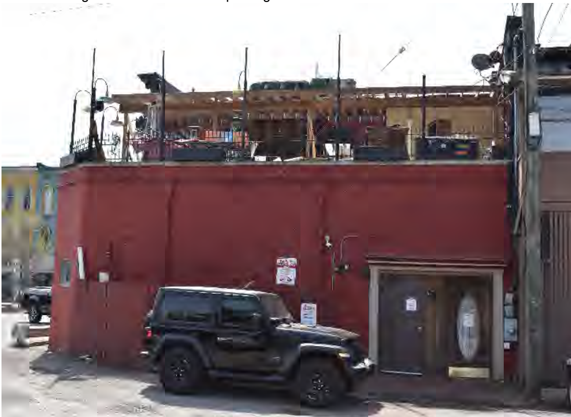
Facing south from parking area.
