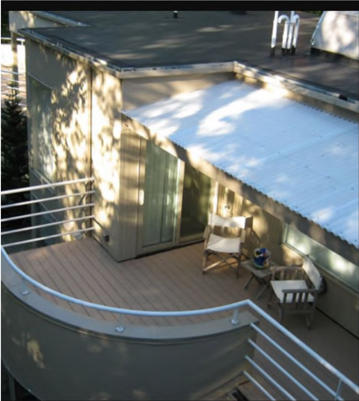
Metal roof example.
