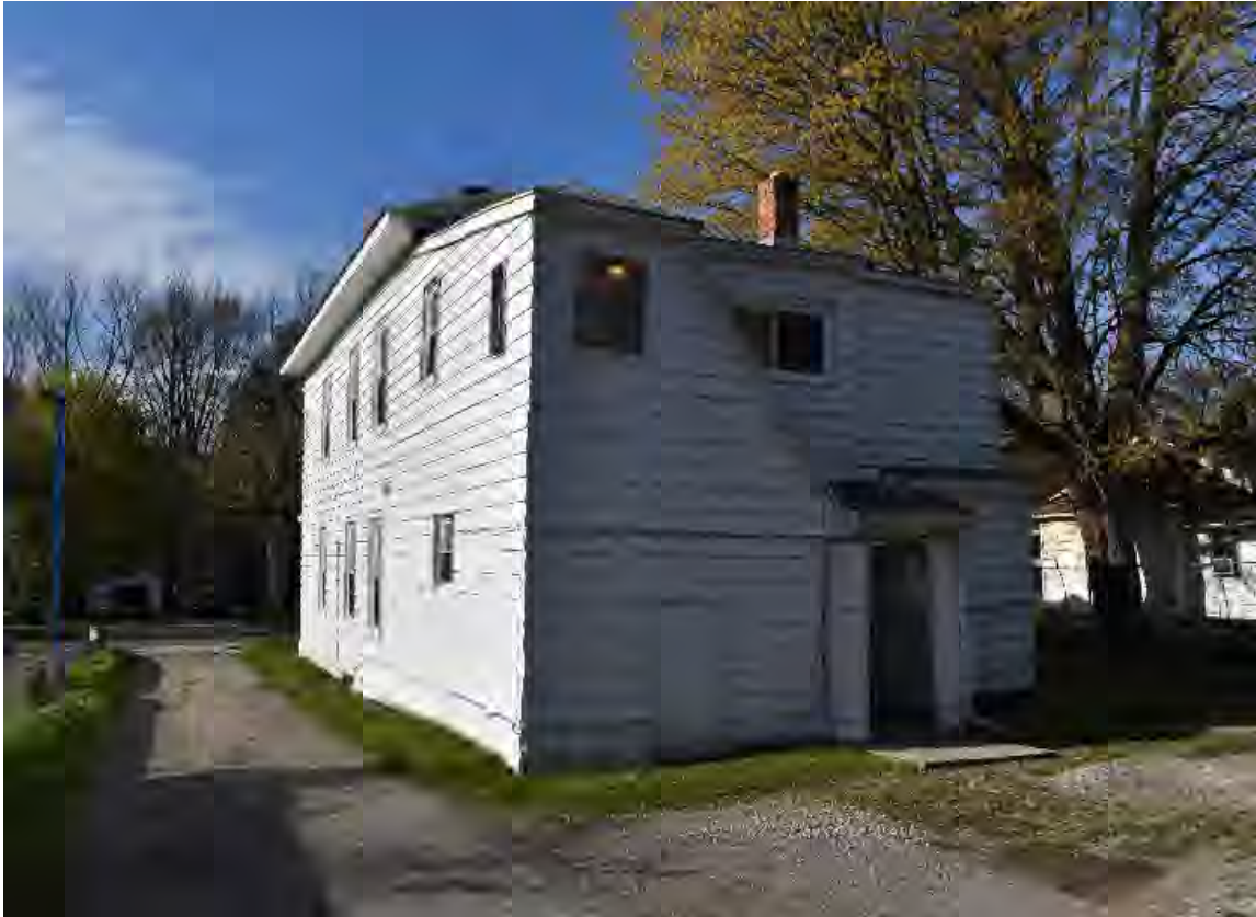
Facing southwest to east elevation.
