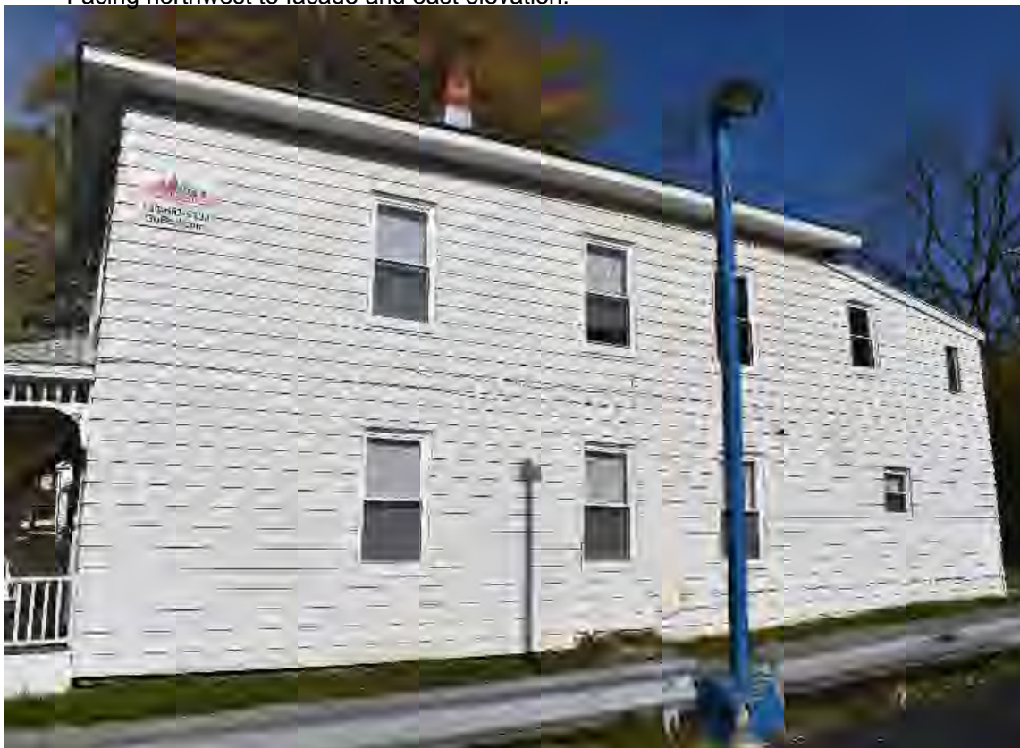
Facing northwest to east elevation.
