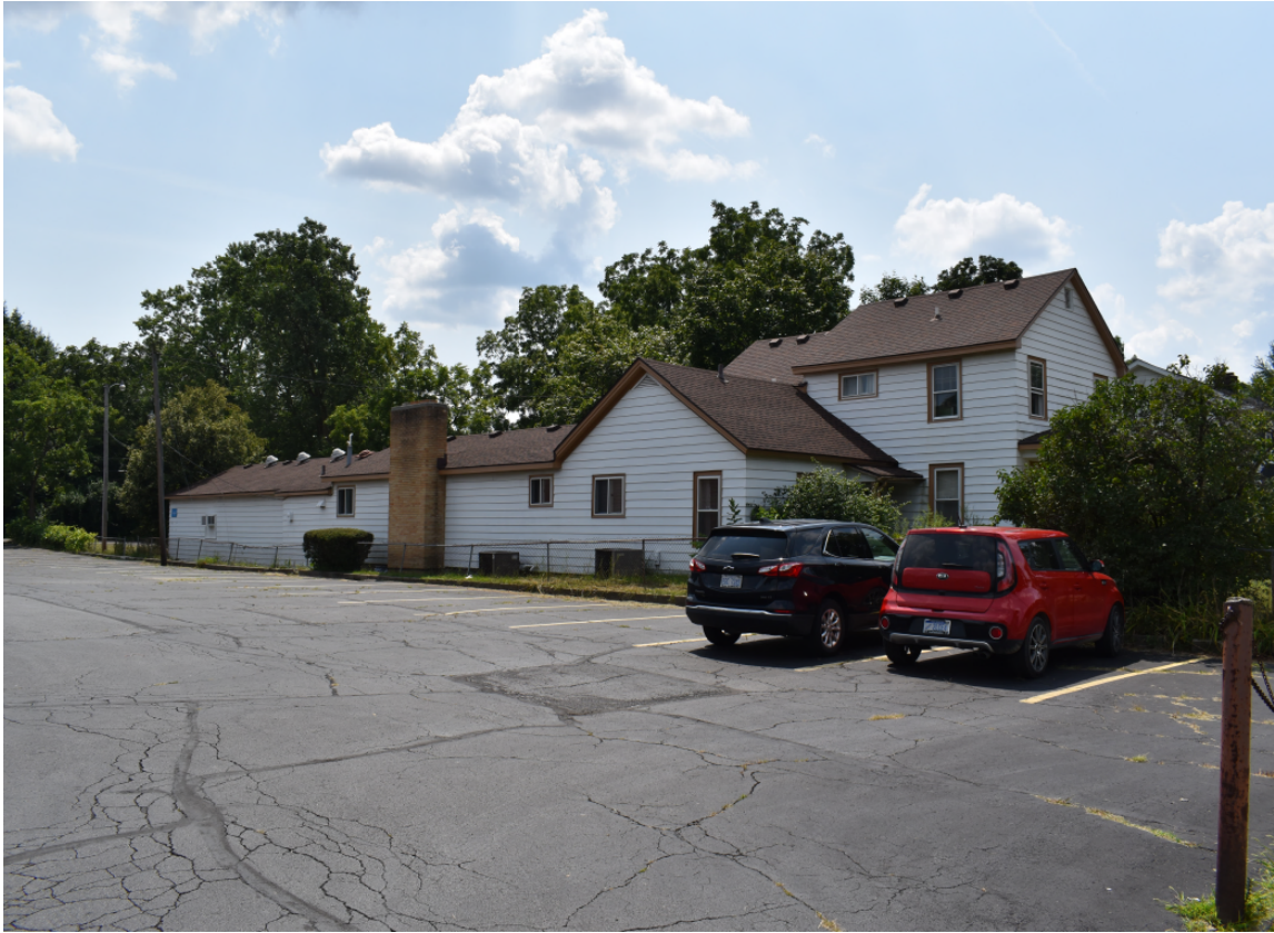
Facing southeast to east elevation. Solar arrays to be placed on the one-story addition.
