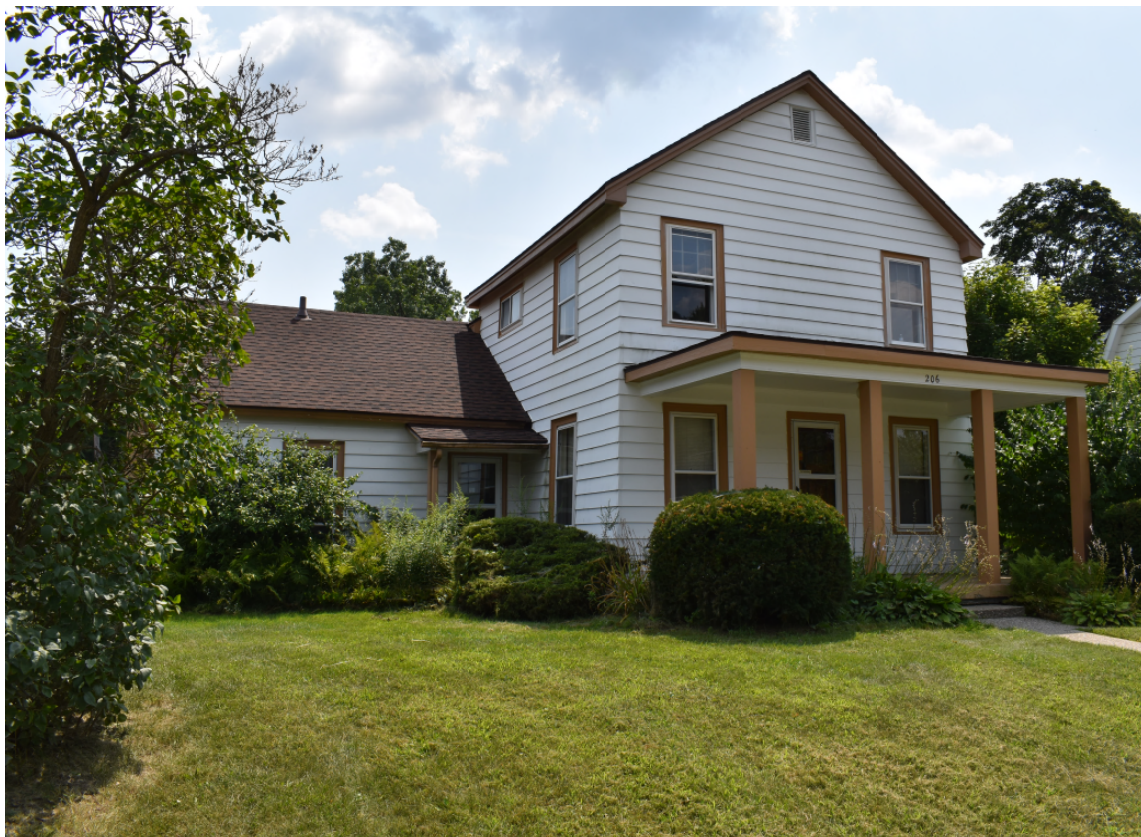
Facing southwest to facade and east elevation.
