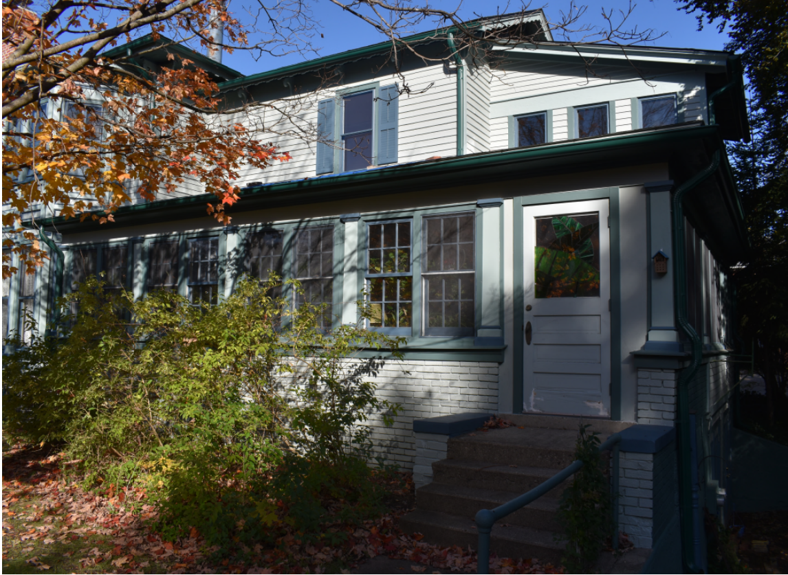
Facing northwest to south porch.
