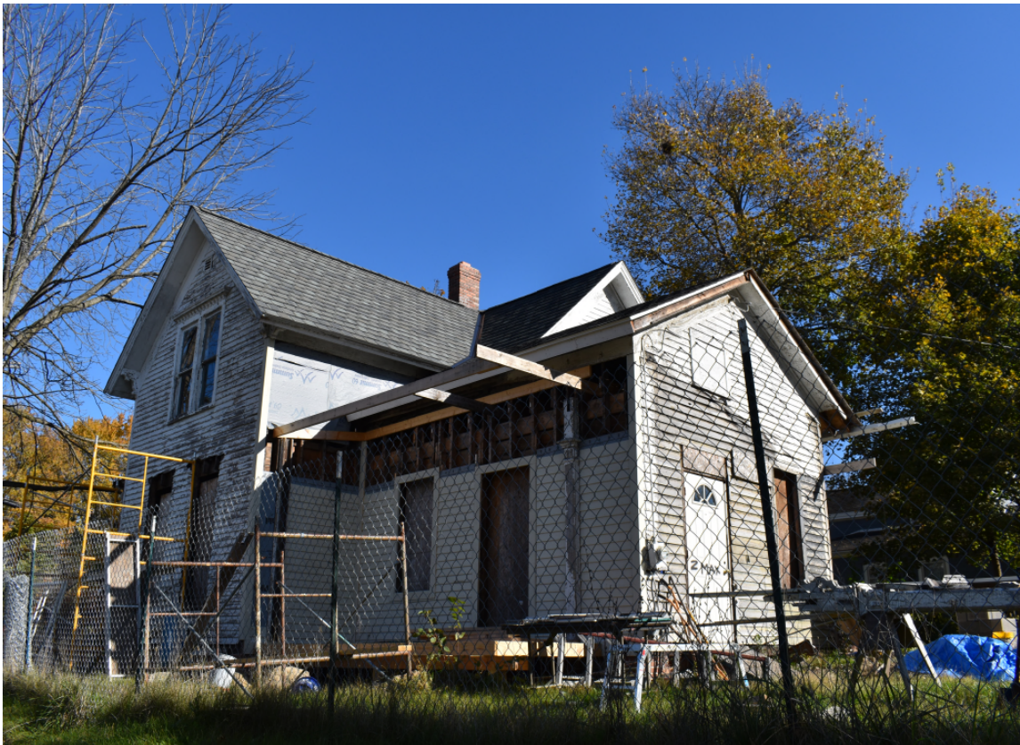
Facing northeast to south and west elevations
