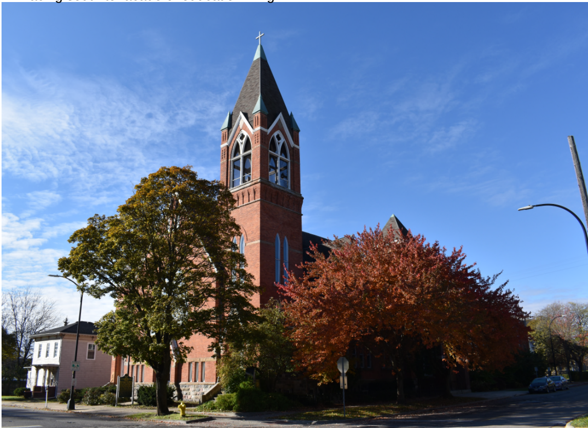
Facing southwest to Washington and Washtenaw facades
