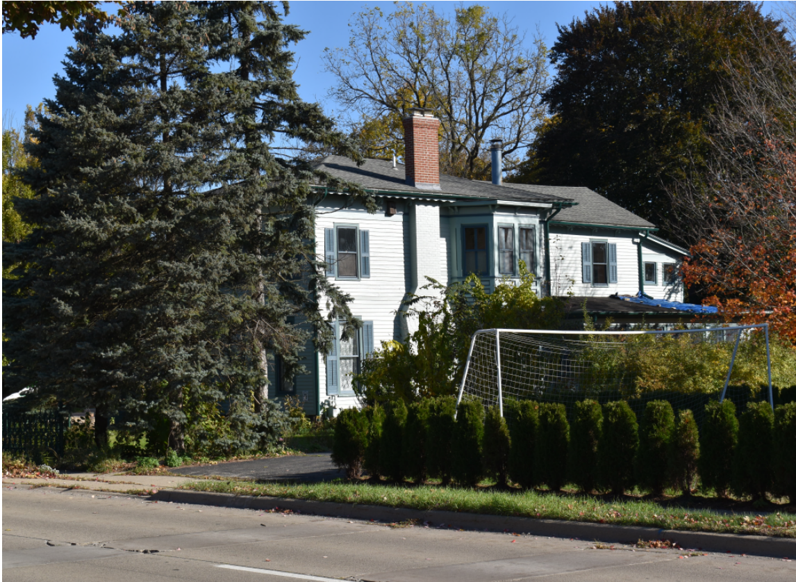
Facing northeast to facade and south elevation
