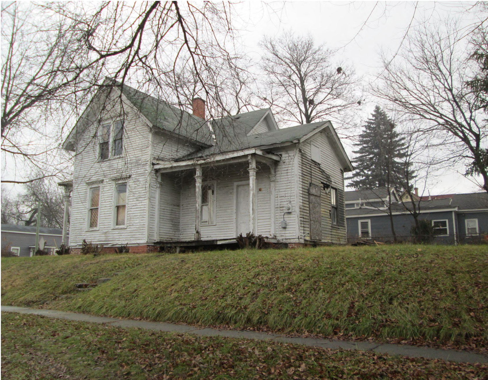
View of west porch in 2018 before removal.
