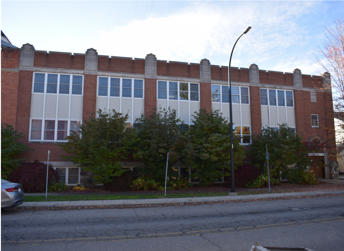
Facing south to facade of education wing
