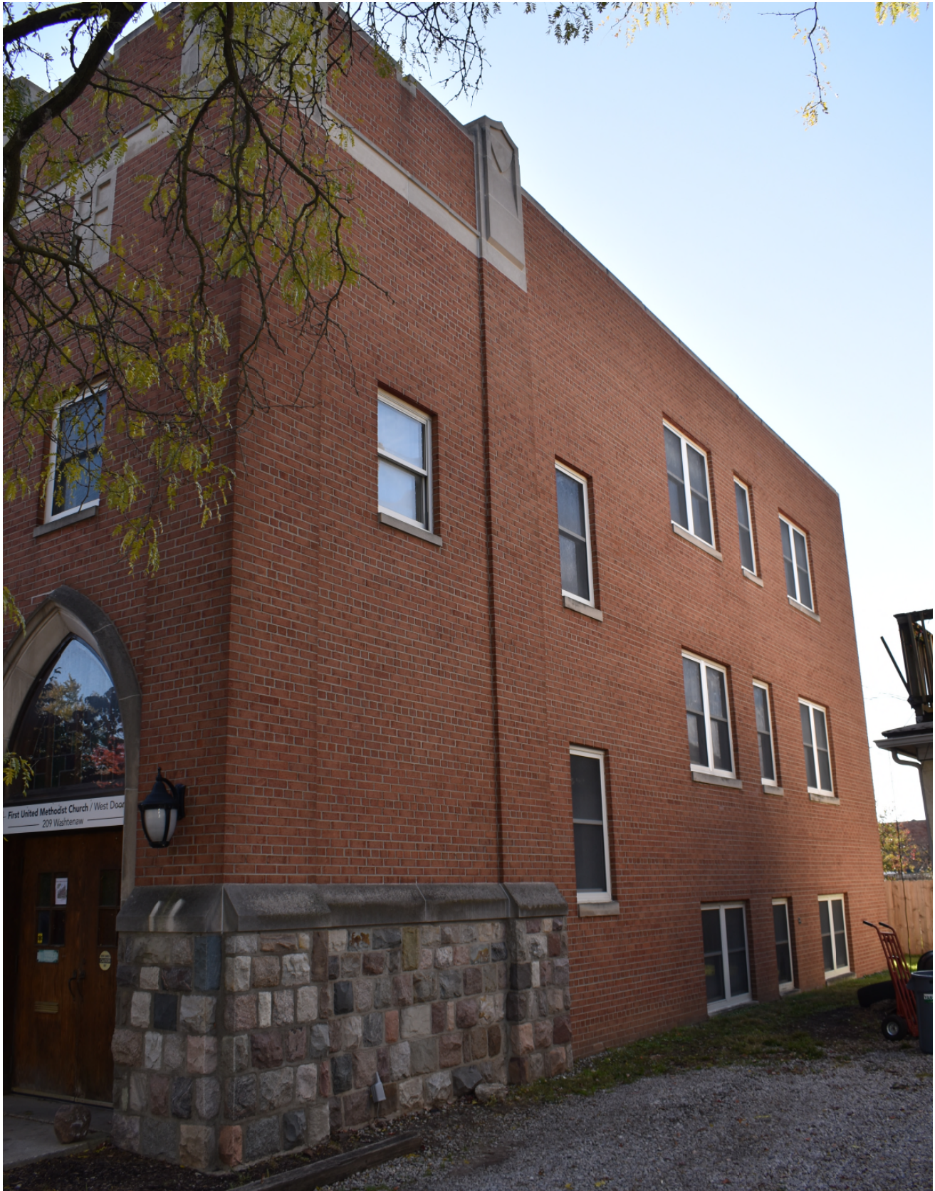
Facing southeast to west elevation
