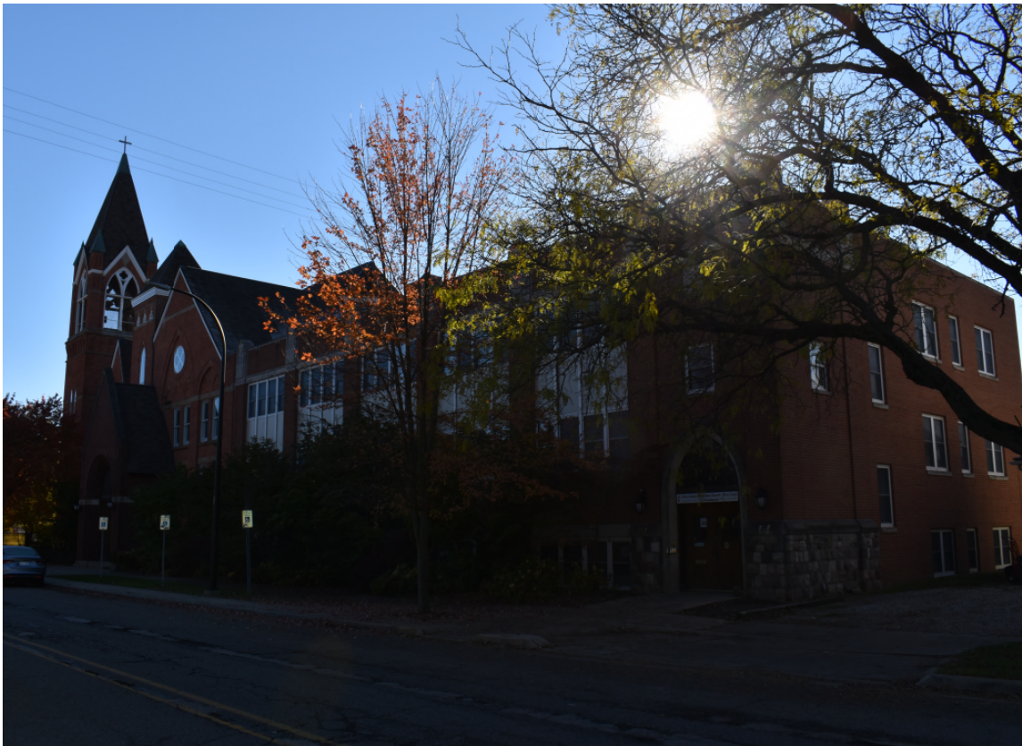
Facing southwest to facade and west elevation of education wing
