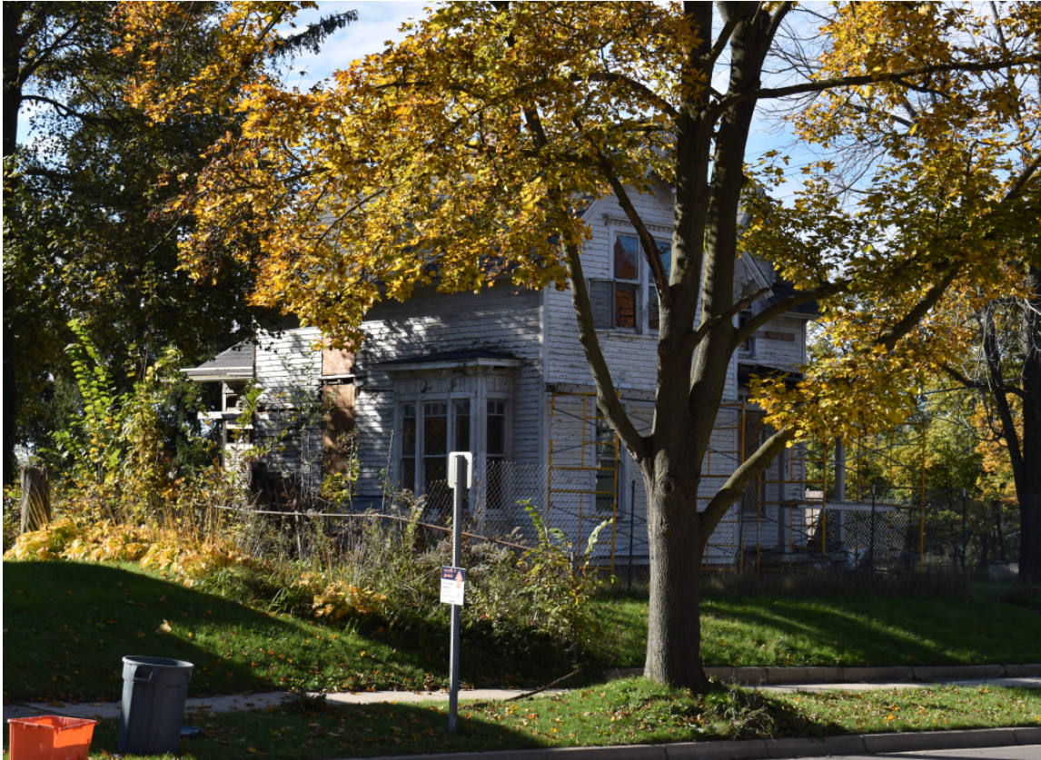
Facing southwest to facade and east elevation
