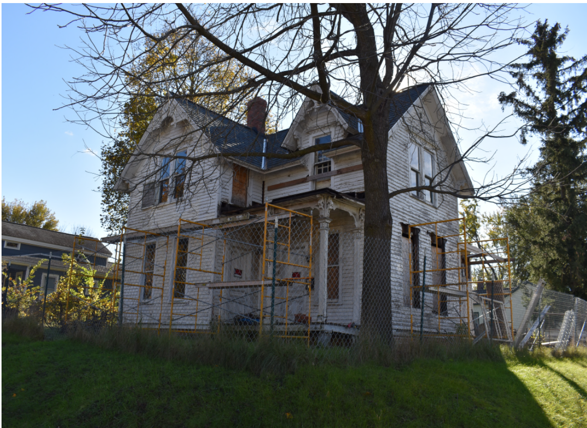
Facing southeast to facade and west elevation
