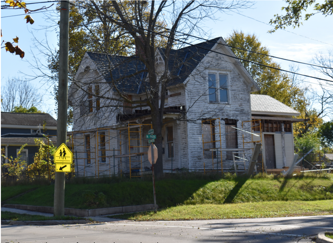
Facing southeast to facade and west elevation
