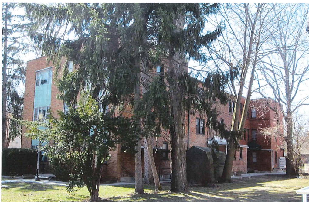
Shots showing rear additions, 2019.
