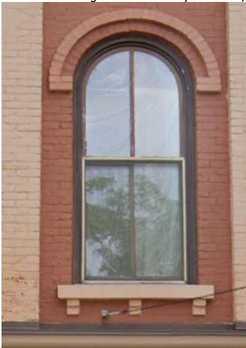
Detail of second-story window, July 2019, 18-20 N Washington (Google).
