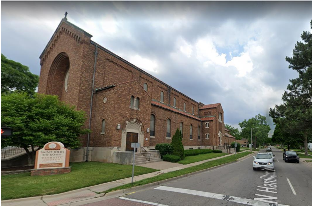
St John the Baptist at the corner of Hamilton and Cross, from Google, June 2021.
