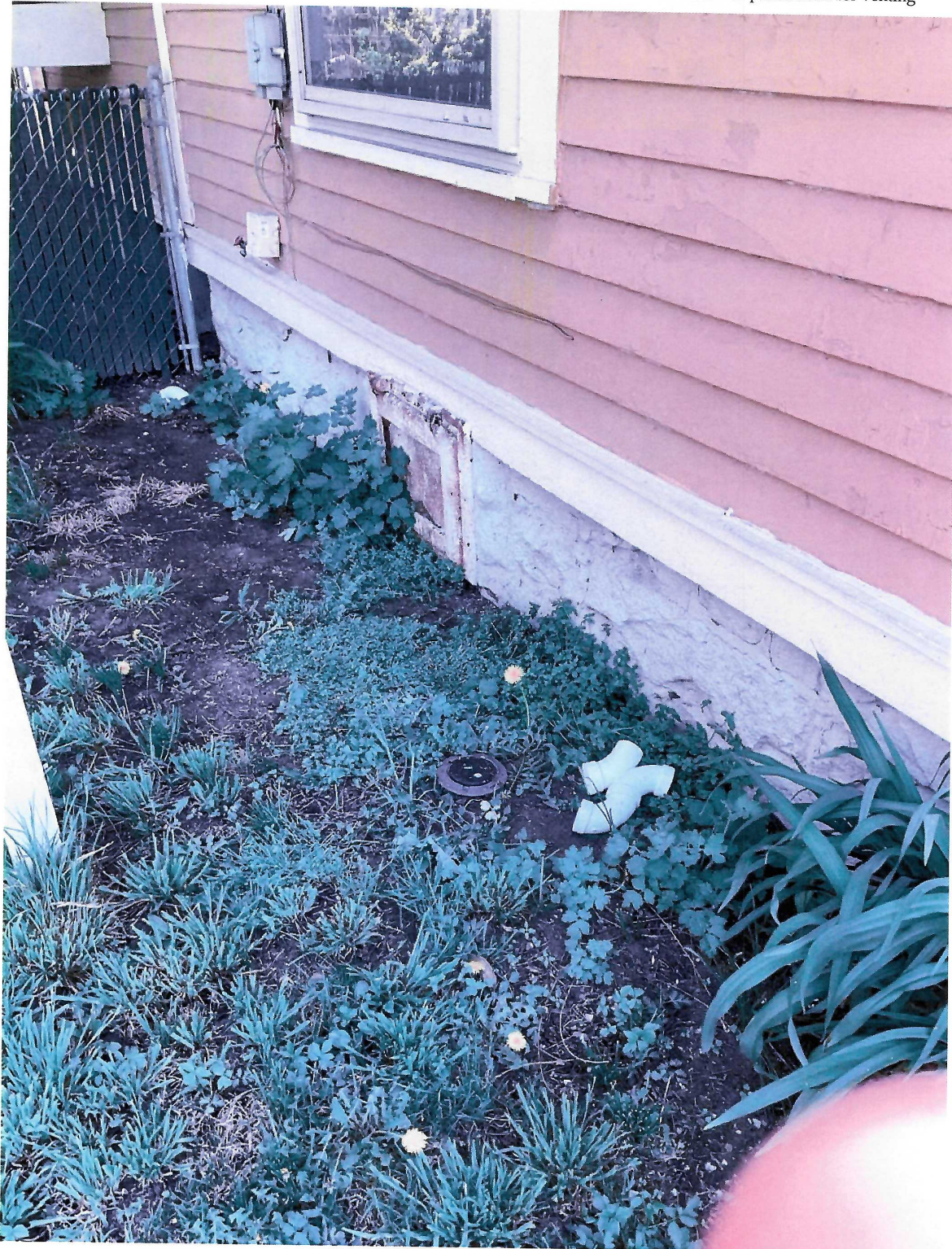
Washington, 315 S -Location of penetration for venting
