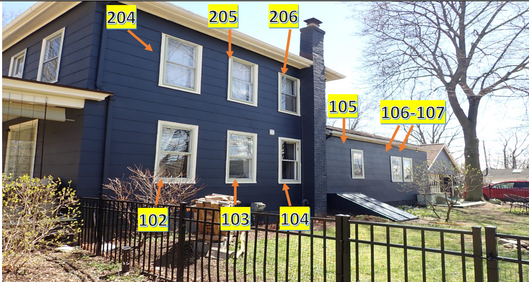
RIGHT SIDE OF HOUSE 21 windows and 1 entry door being replaced
