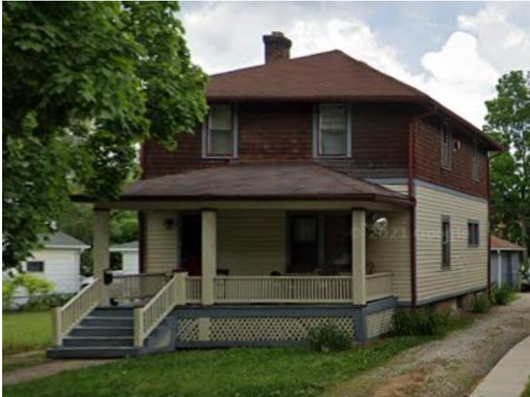
Figure 1. Photo from Google June 2021. Original porch railing and handrails.
