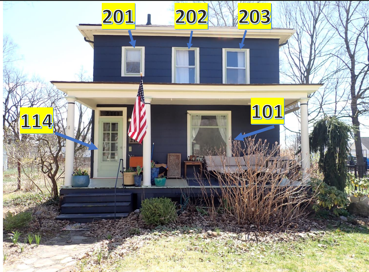
FRONT OF HOUSE 21 windows and 1 entry door being replaced
