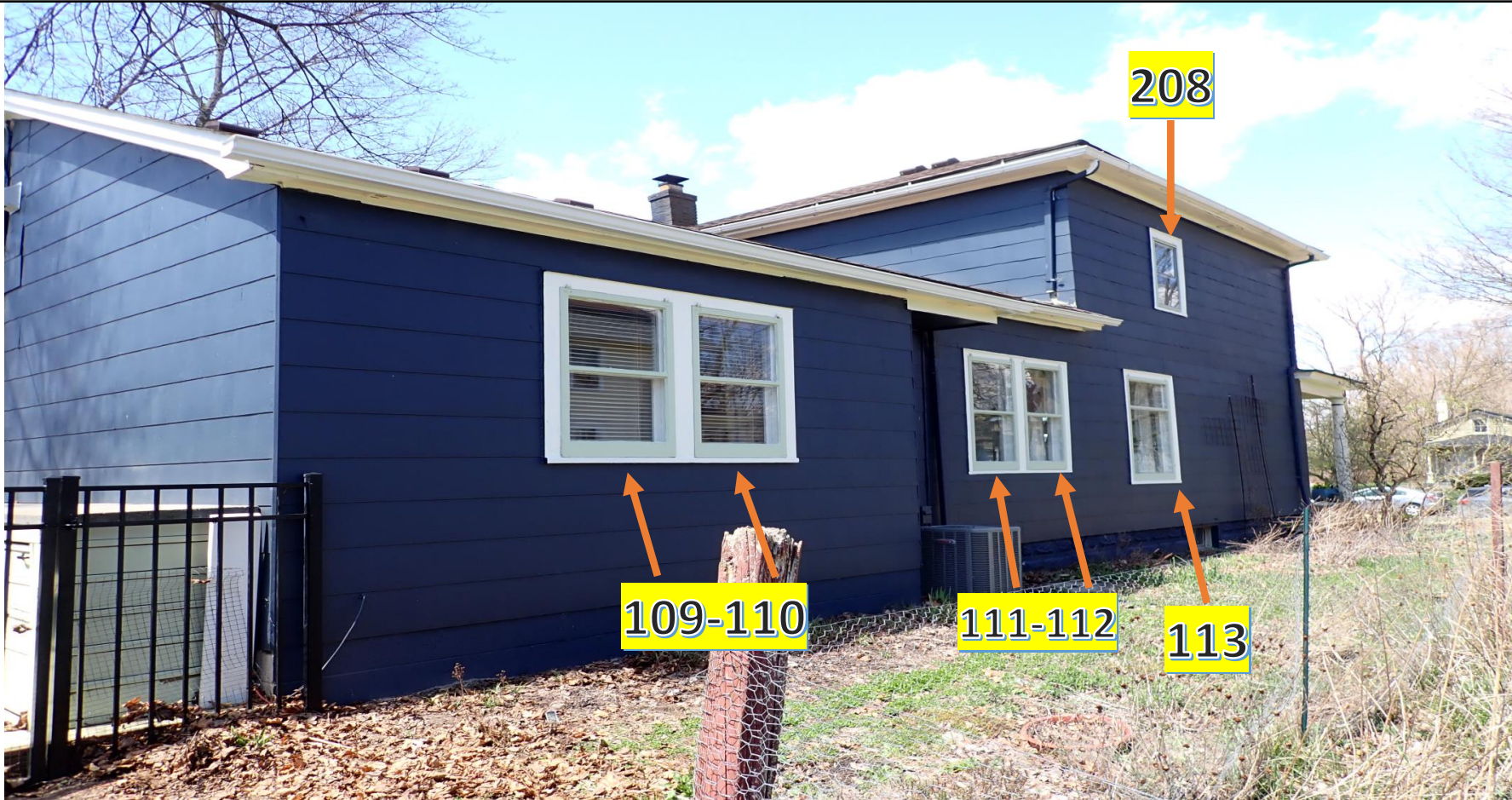
LEFT SIDE OF HOUSE 21 windows and 1 entry door being replaced
