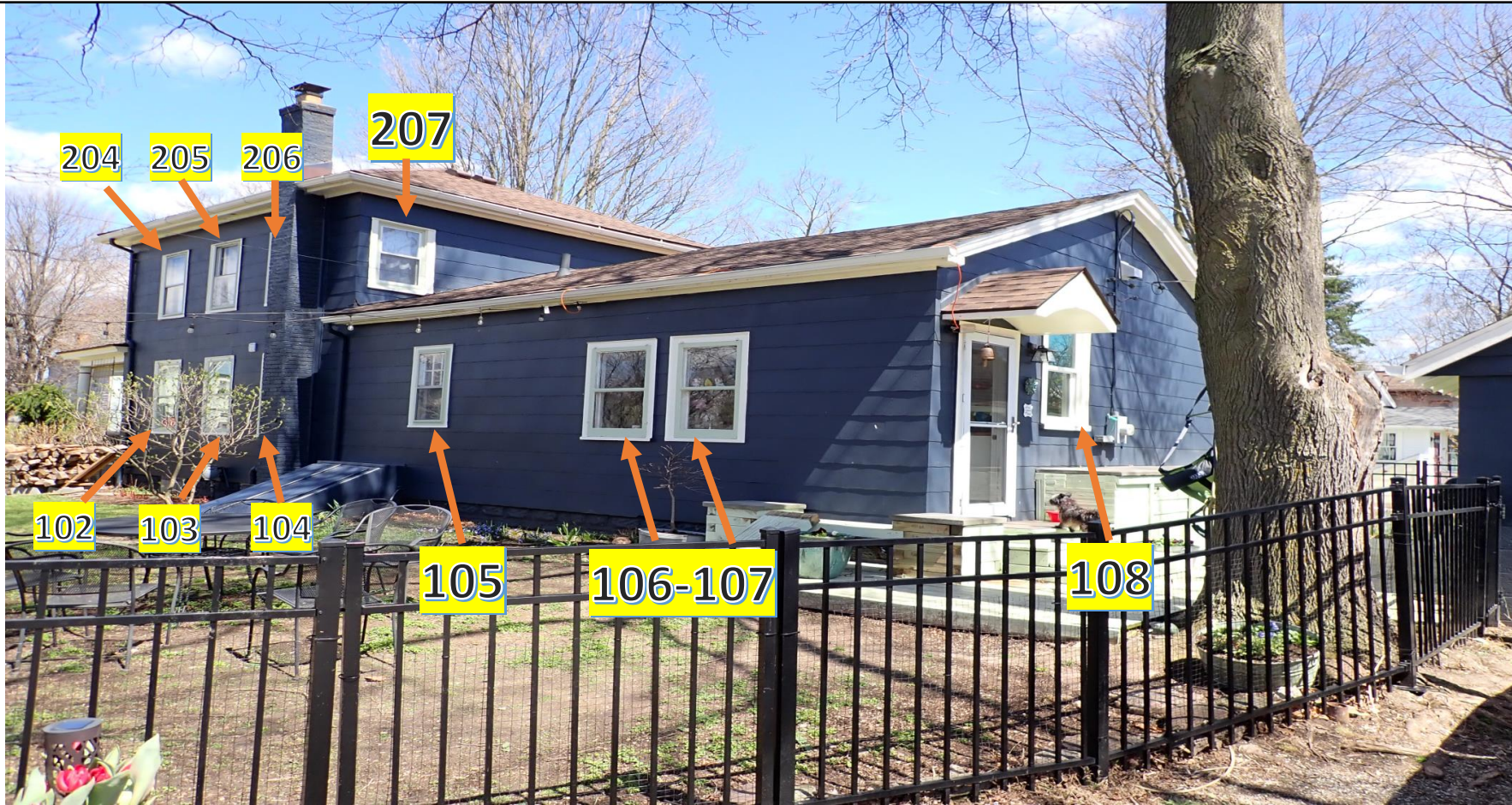
BACK / RIGHT SIDE OF HOUSE 21 windows and 1 entry door being replaced
