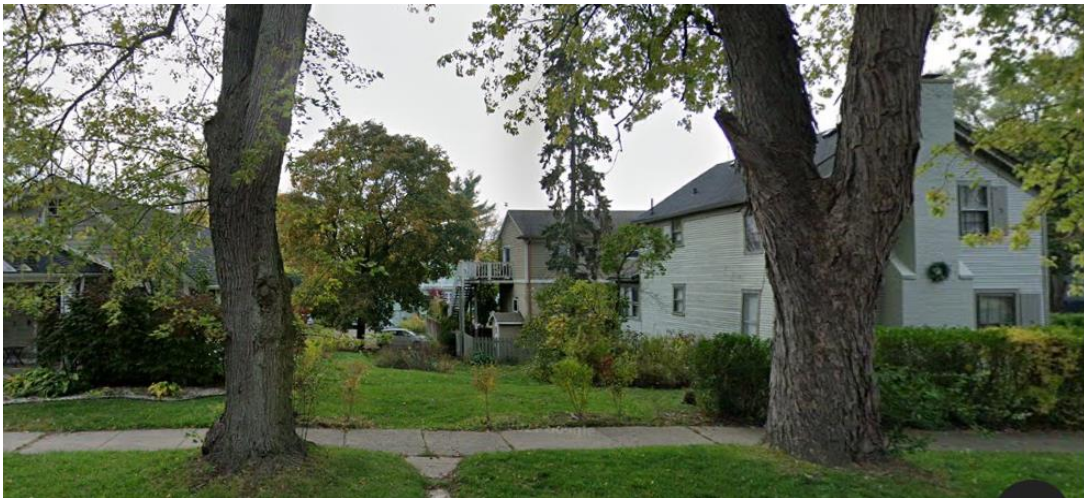
House, east end and most of the south side visible. The south side is where the solar array is being proposed. (Google, June 2021)
