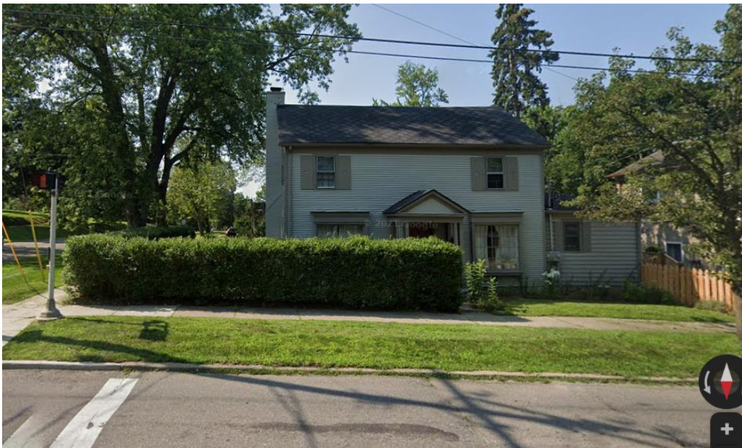
Front (north side) of house from a slightly different angle so that the one-story addition to the west is visible. (Google, June 2021)
