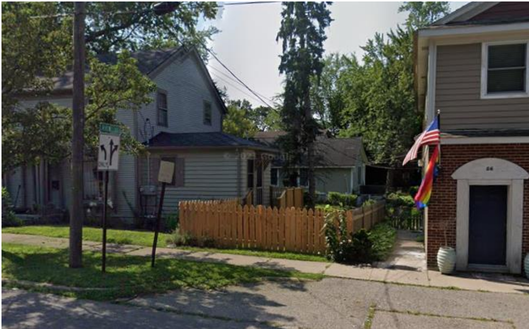
Front (north side) of house with meters and conduit visible. (Google, June 2021)
