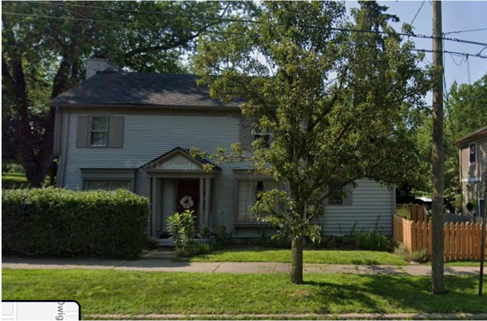
Front, north side of the house on E Forest. (Google, June 2021)
