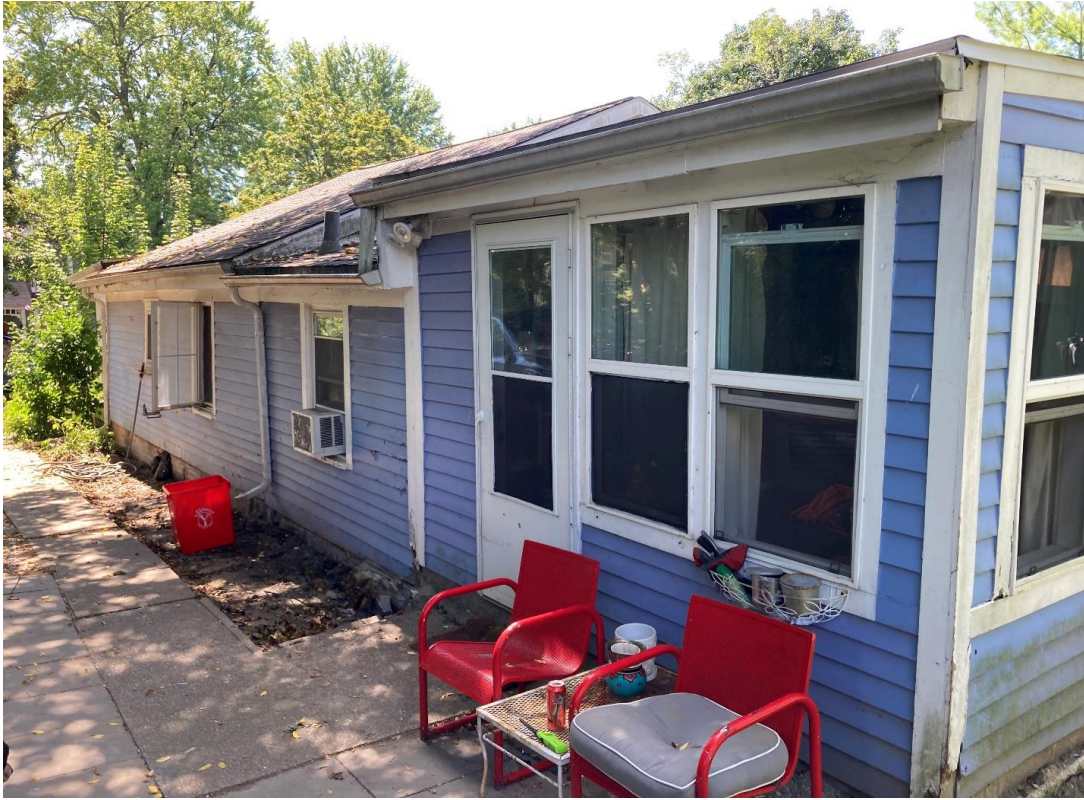
East side from the rear (north).
