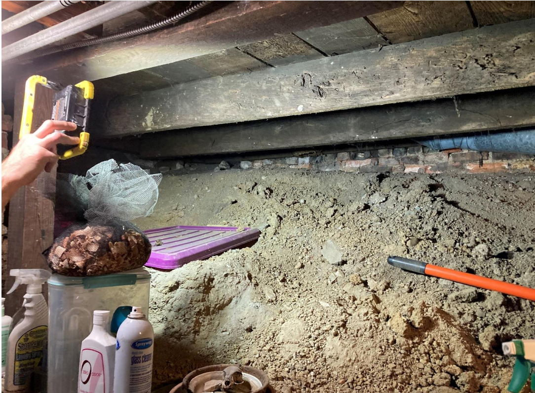
The pile of dirt, looking at the east brick wall of the foundation, along the driveway, through the opening cut in the brick shown in the previous picture.
