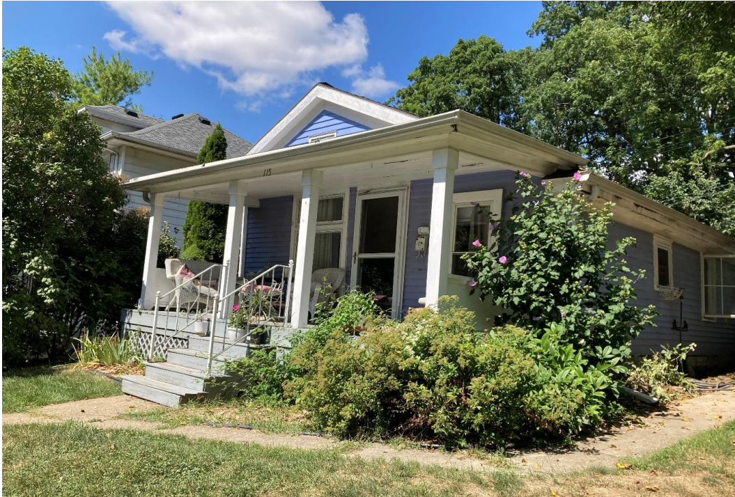
South (front) end and east side along driveway.
