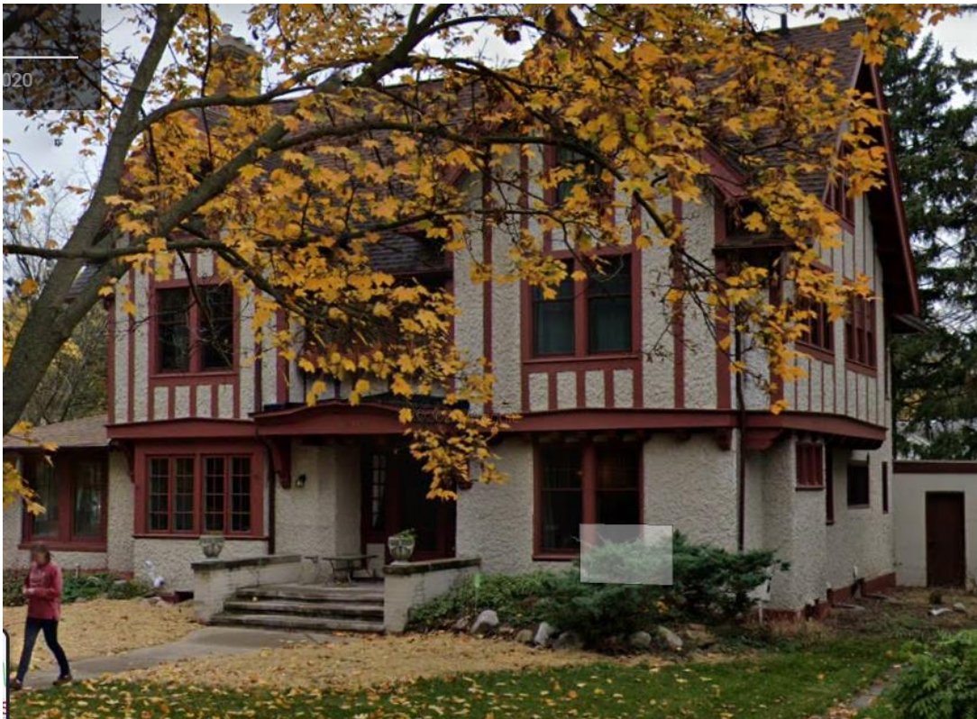
216 S Washington from Google streetview October, 2020.
