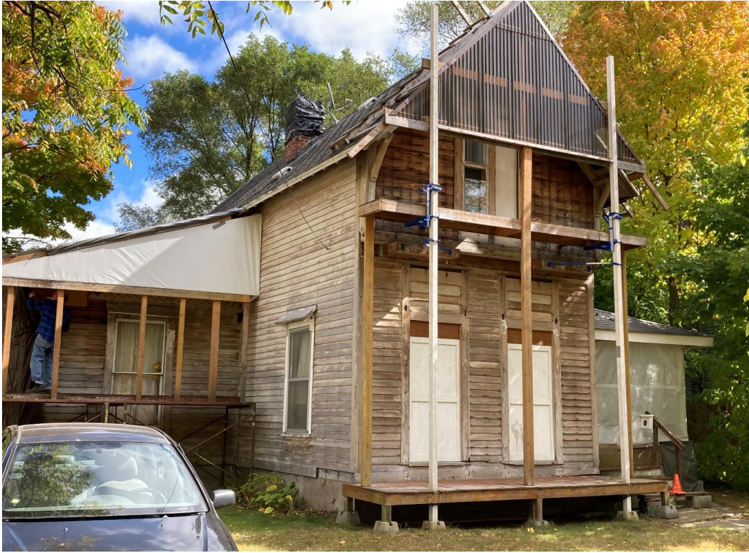
218 N River, west façade, October 7, 2022. Chimney can be seen covered here with black plastic. (staff photo)
