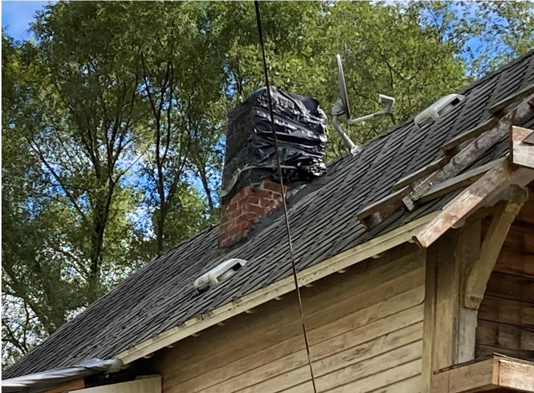
218 N River, chimney detail, October 7, 2022. (staff photo)
