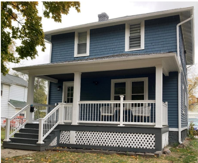
Figure 3. Photo taken by staff October 18, 2022. New porch railing and handrails, painted white.
