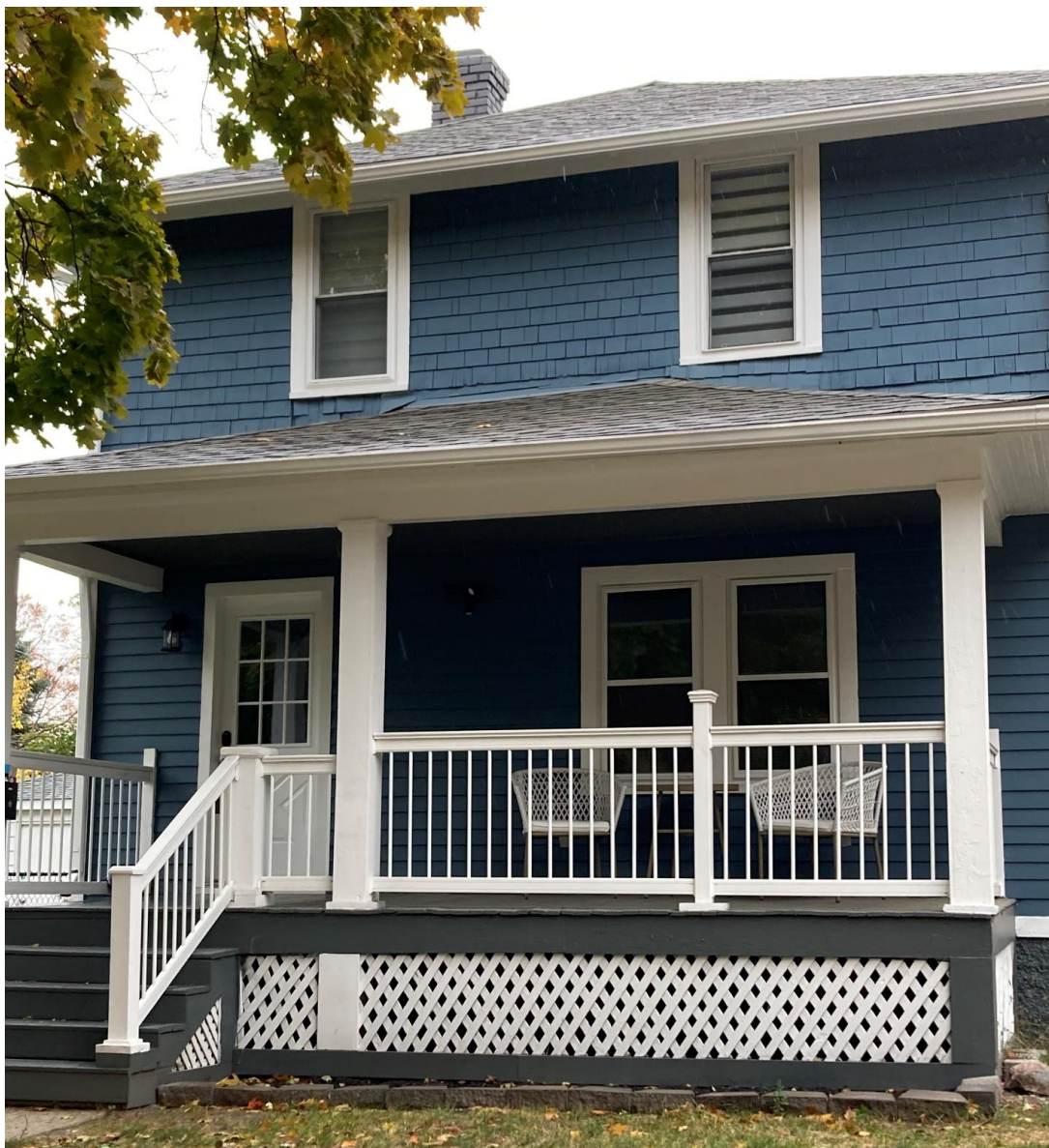
Figure 4. Closer-up photo of porch rail and handrails. (Staff, October 18, 2022)
