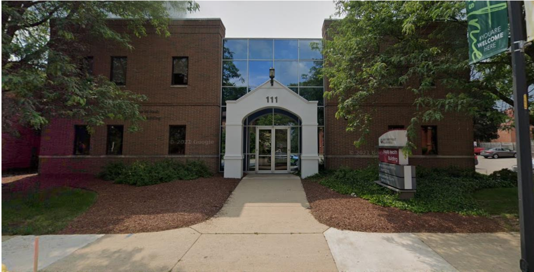
Above, east elevation, 111 N Huron, from Google streetview, 2021.
