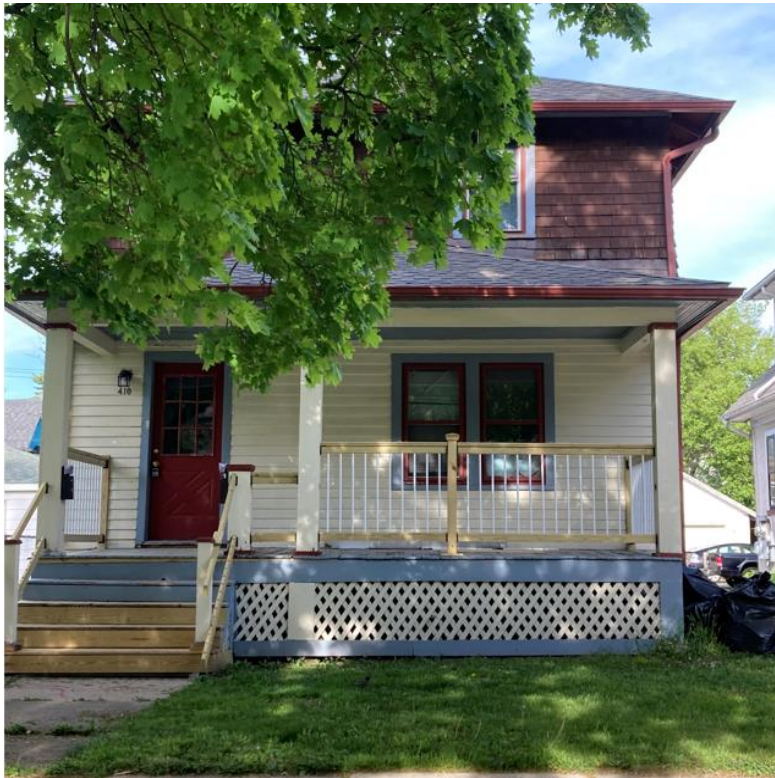
Figure 2. New porch railing and handrails, staff photo, May 2022.
