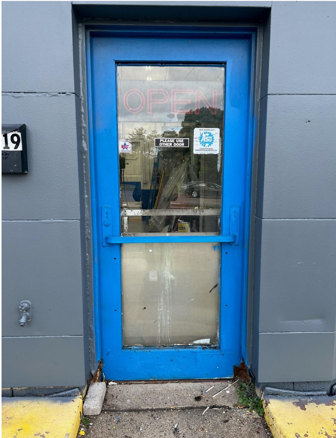
Shop Door into Garage:
