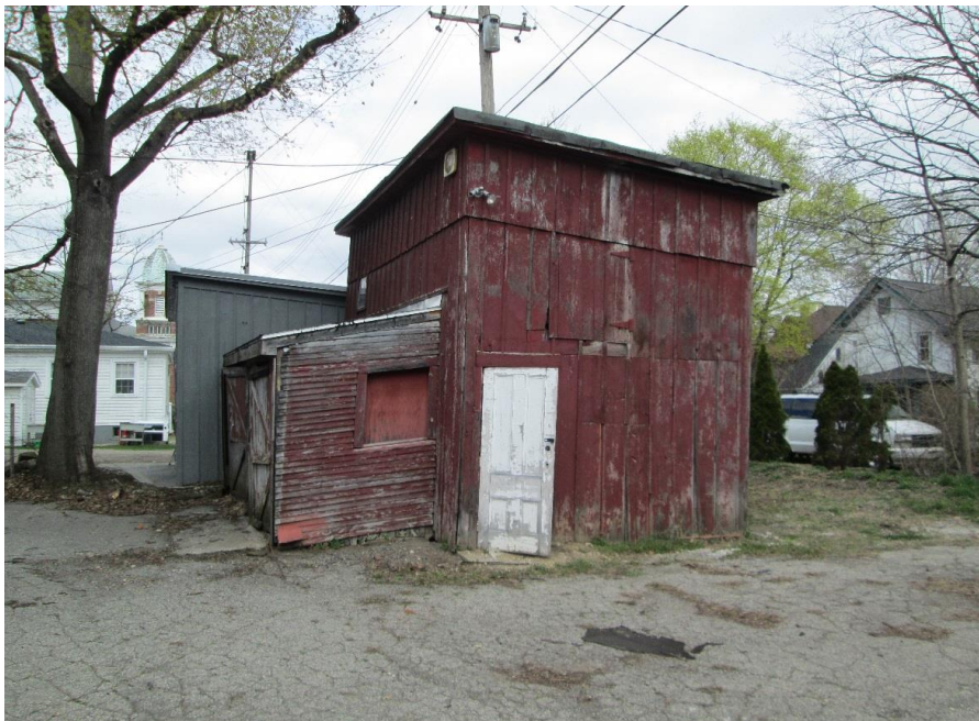
206-210 N. Washington, north carriage barn, 2019. Photo looking northeast to south and west elevations.
