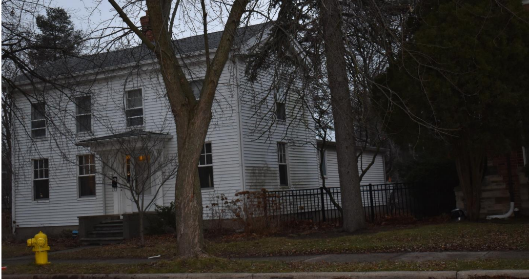
Figure 2. 307 N Washington. The front elevation is the house's east side. Here, the north end (side) of the house with the gable and Greek Revival detailing is also visible, as is the rear addition. Solar panels are proposed on the roof visible at the front of the house, and also on the roof of the addition, on the southern slope.
