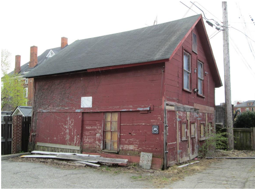
206-210 N. Washington, south carriage barn, 2019. Photo looking southeast to north and west elevations.
