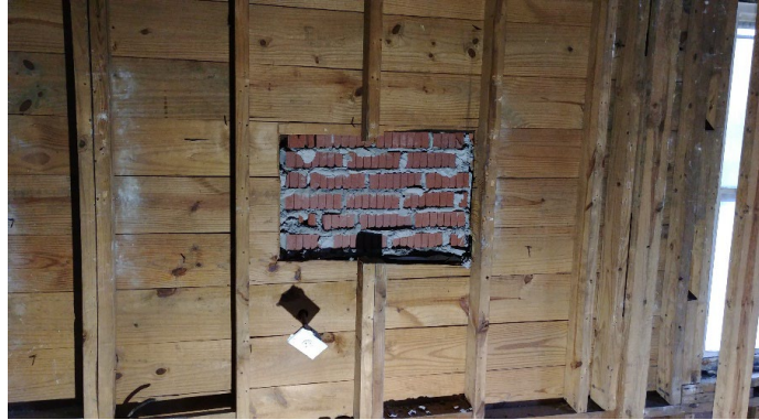
Figure 2: Example of Wall Framing Discontinuity
