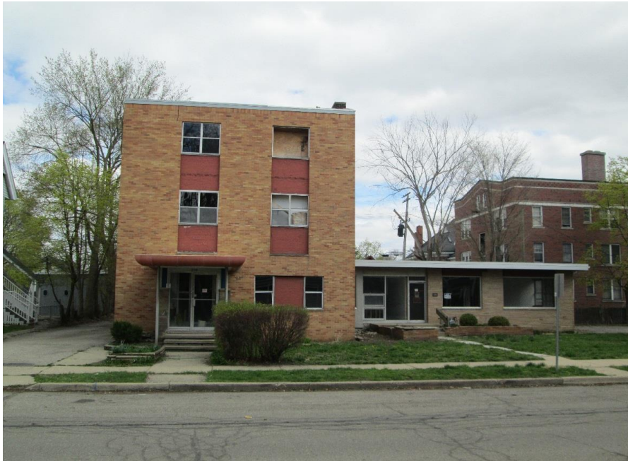
206-210 N. Washington, 2019. Photo looking east to facade.
