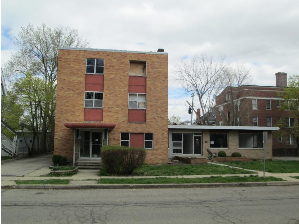
206-210 N. Washington, 2019. Photo looking east to facade.
