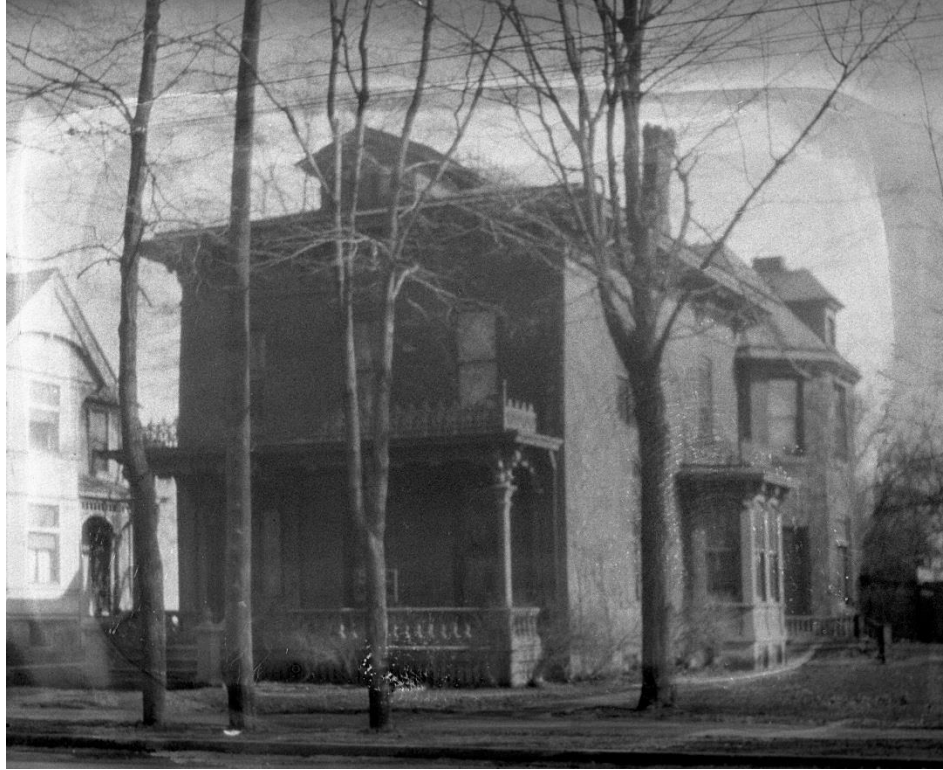
206-210 N. Washington, ca. 1900. Photo looking northeast to façade and south elevation.
