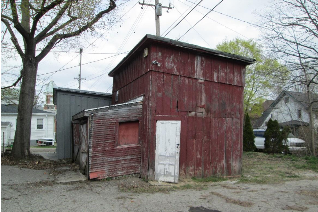
206-210 N. Washington, north carriage barn, 2019. Photo looking northeast to south and west elevations.
