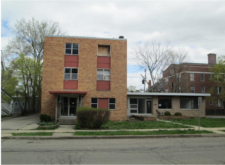
206-210 N. Washington, 2019. Photo looking east to facade.
