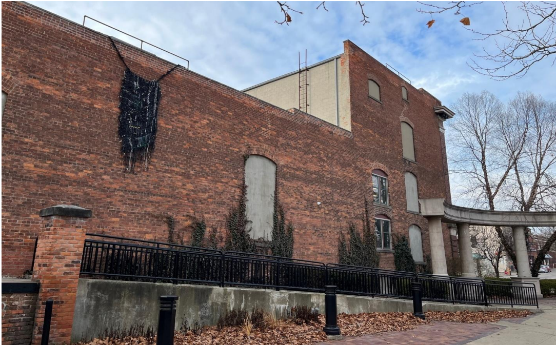
Photo 2. North side of 76 N Huron from the northeast. Again, it is clear that the third floor is smaller than the floors below. The non-original, cement block wall that forms the rear (east) wall of the third floor, where the new windows are being proposed, is just visible.
