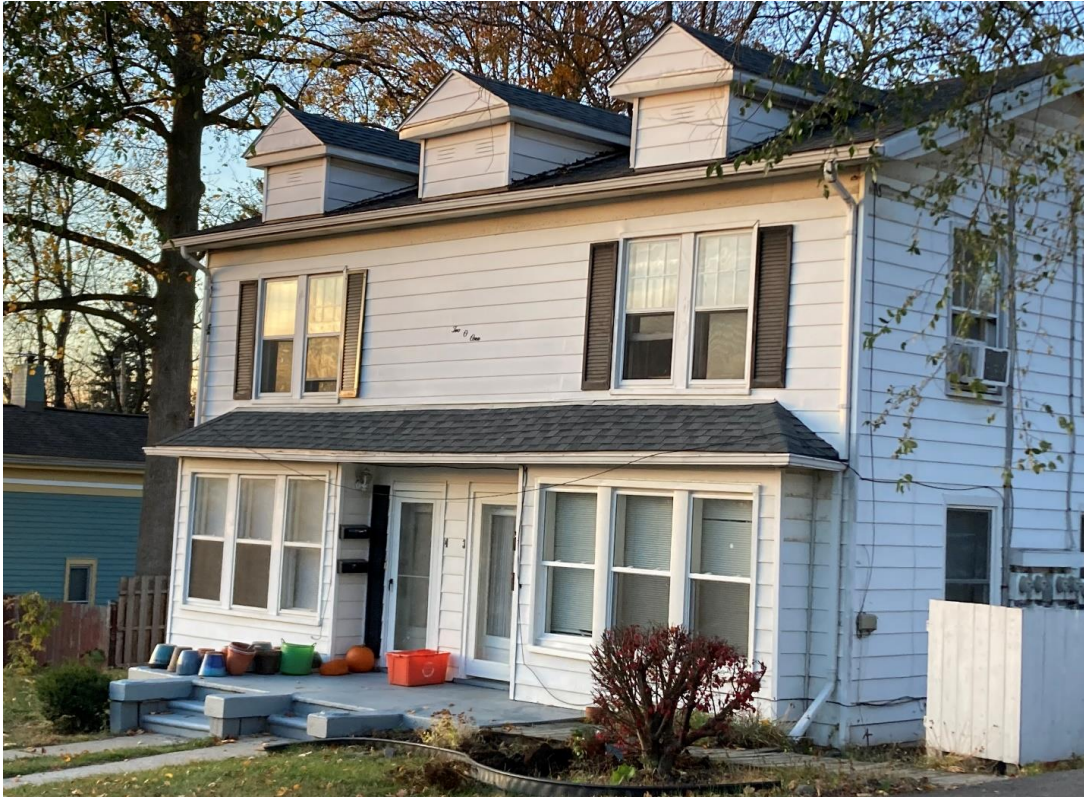
Photo taken by staff, November 8, 2022. Three windows on the lower right behind the shrub were replaced.
