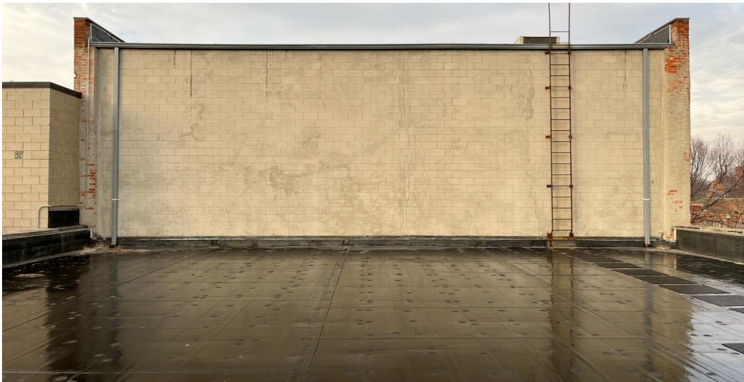
Photo 3. Standing on the roof over the second floor, looking from the building's rear (east) toward the west. This is the filled-in, cement block, rear wall for the third floor, where the windows are proposed to be installed.
