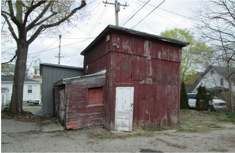
206-210 N. Washington, north carriage barn, 2019. Photo looking northeast to south and west elevations.
