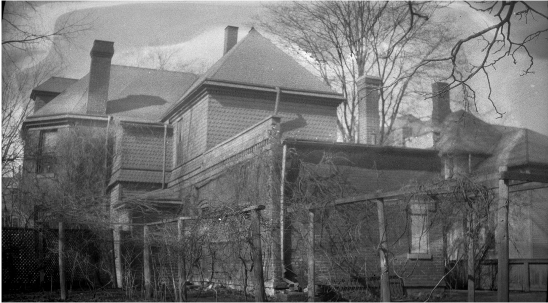
206-210 N. Washington, ca. 1900. Photo looking northwest to east and south elevations.
