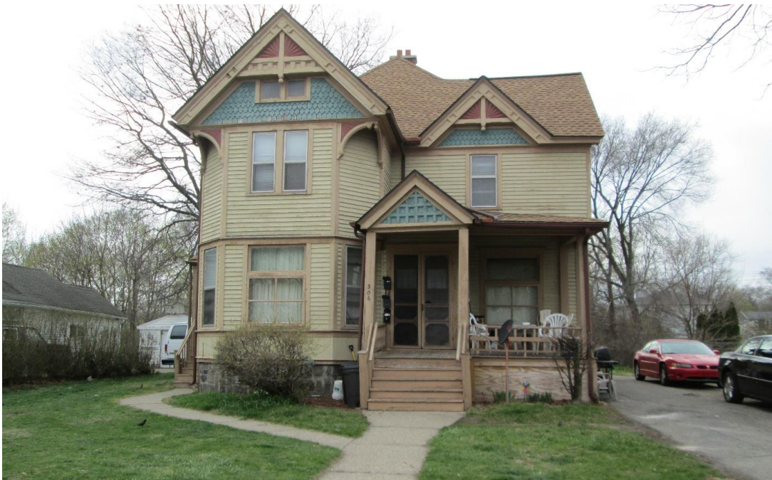
306 S Washington, 2015, picture on file. This guardrail was not historic. Thin pieces of wood were covering the historic turned porch posts to create square porch posts for the guardrails and handrails.
