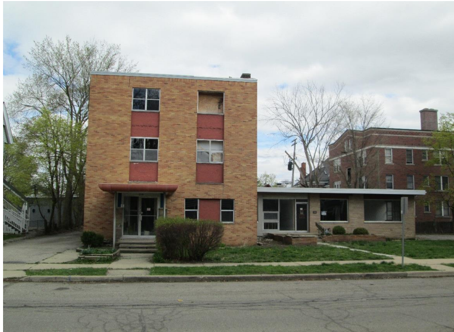
206-210 N. Washington, 2019. Photo looking east to facade.
