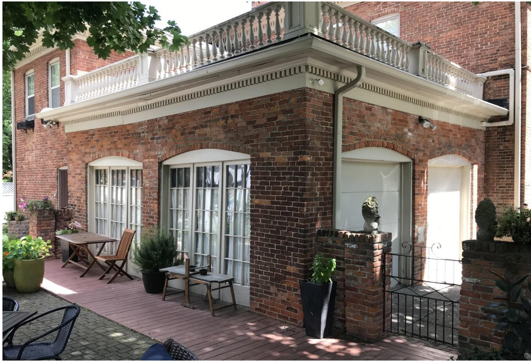
Photo provided by the applicant of project area—the garage doors on the south side are shown here, as well as the panels of windows on the rear (west side) that are proposed to be replaced. The windows to the left would be the shortened windows with infill brick below and the windows on the right would be French doors.
