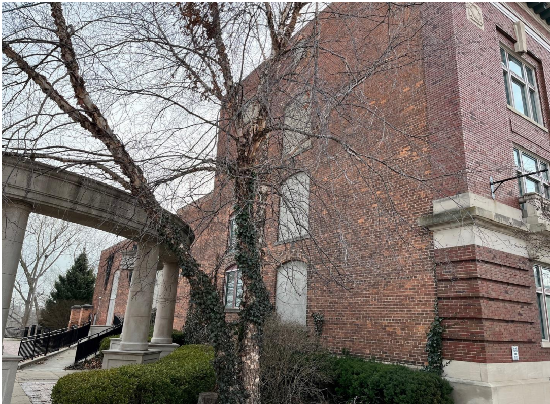
Photo 1. For context, this picture shows a little of the front (west) façade of 76 N Huron, but also the entire north side of the building. It is visible that the third floor ends abruptly and that the first and second floors go back toward the rear (east) much further than the third floor does.
