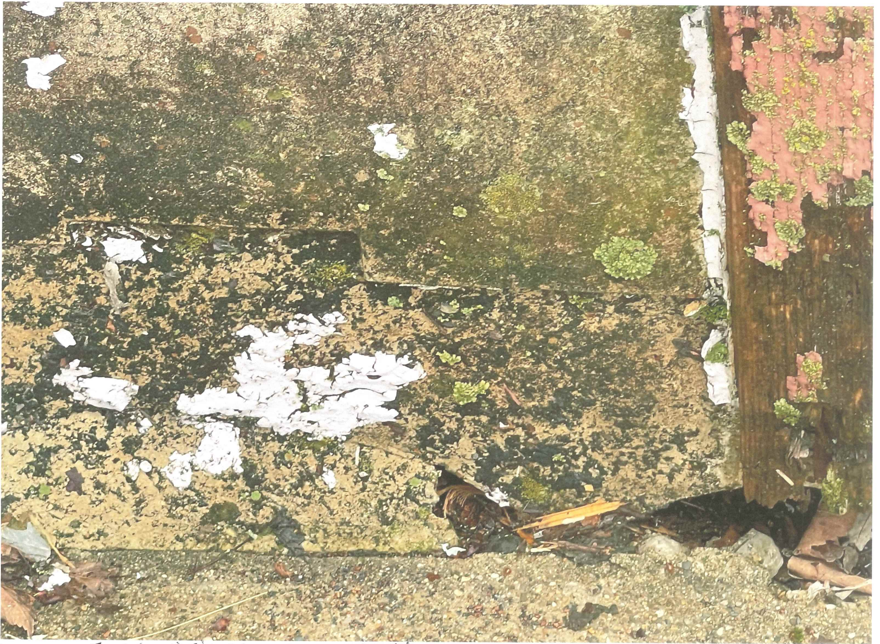
DETAIL of Front (East) Side of house where vertical trim meets concrete porch. 627 N River, April 2023
