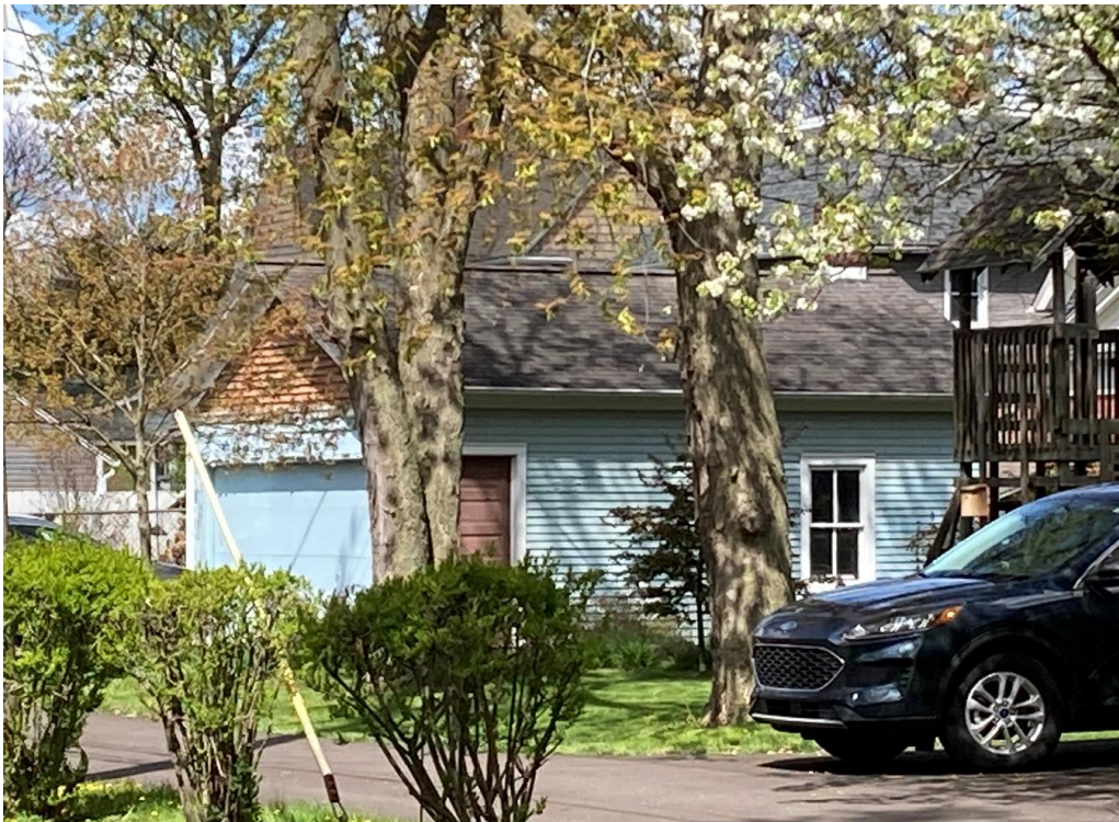
Garage. Steel garage door would replace particleboard pale blue door.
