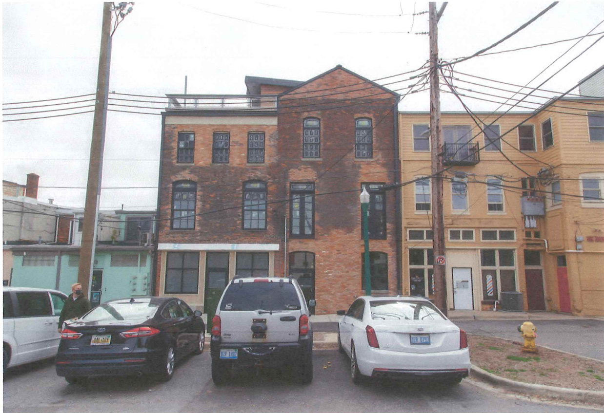
PHOTO OF EXISTING CONDITIONS
