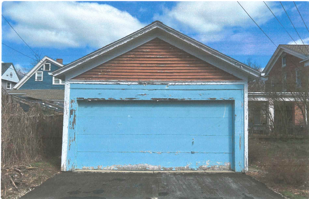
Front Elevation of Existing Door
