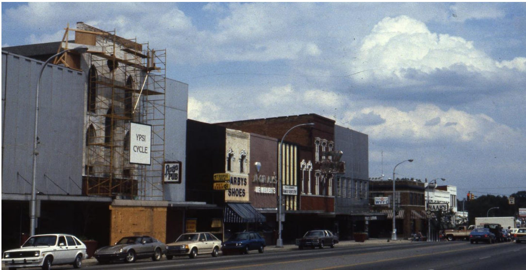
118 W Michigan Ave with its original façade exposed under scaffolding in 1984, Ypsilanti Historical Society.
