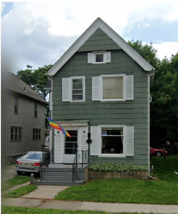
311 Washtenaw, Google streetview, June 2021.
