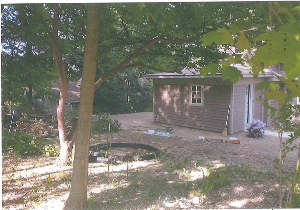
LOOKING SW FROM OAK ST. SIDEWALK
