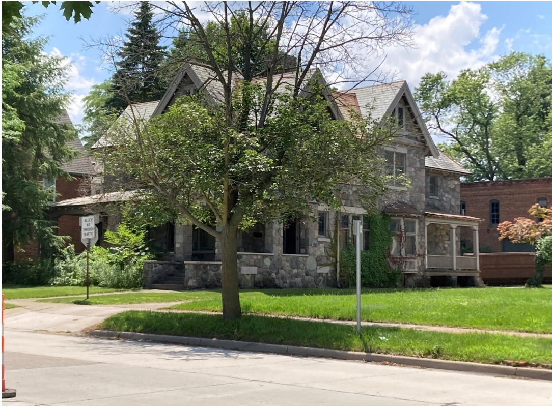
Fig. 2. 212 S Huron from across street, east end (front) and north side along alley. Front porch roof is quite visible from this angle, as are the slate roof on the rear-most portion of the house and the metal roofs on the bay window and porch on the north side of the house.
