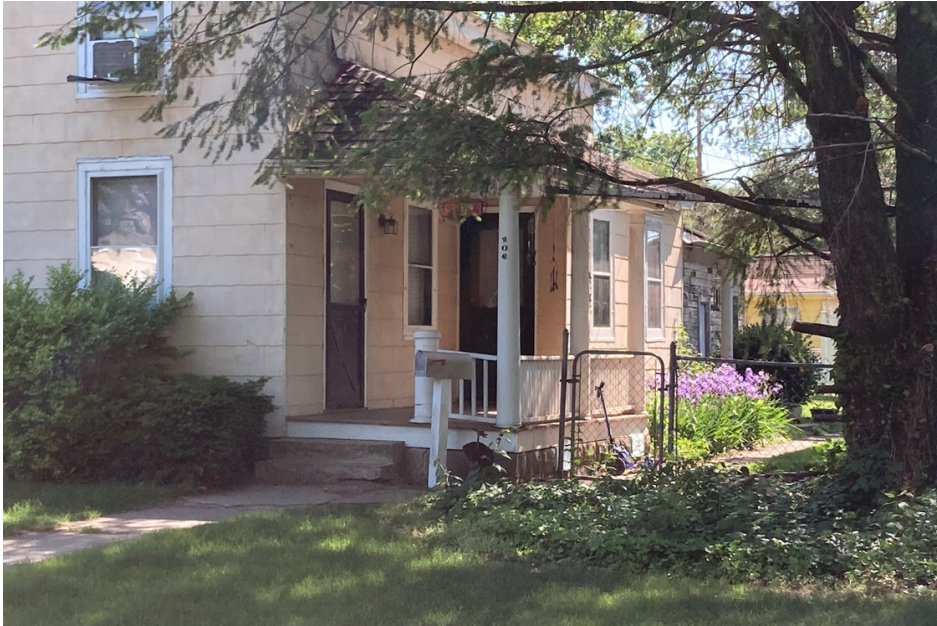
206 N River, southwest corner and southern side of house. Wood-sided portion at very rear of house barely visible here is where the replacement siding is proposed.
