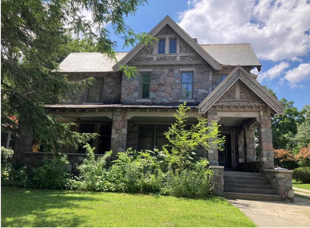
Fig. 1. 212 S Huron, east or front façade from sidewalk. July 2023. The front porch's sloping portion is not really readily visible from this perspective, in staff's view. It does appear here to have more of a shingle texture than a metal one, however.
