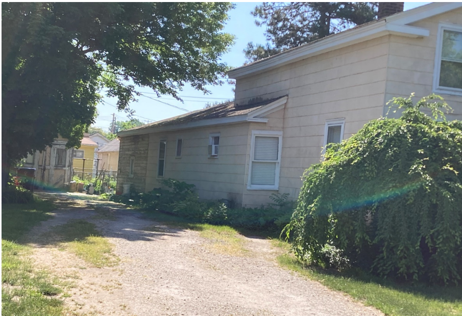
206 N River, north side and northwest corner. Wood-sided portion to rear is portion where siding is proposed to be replaced.
