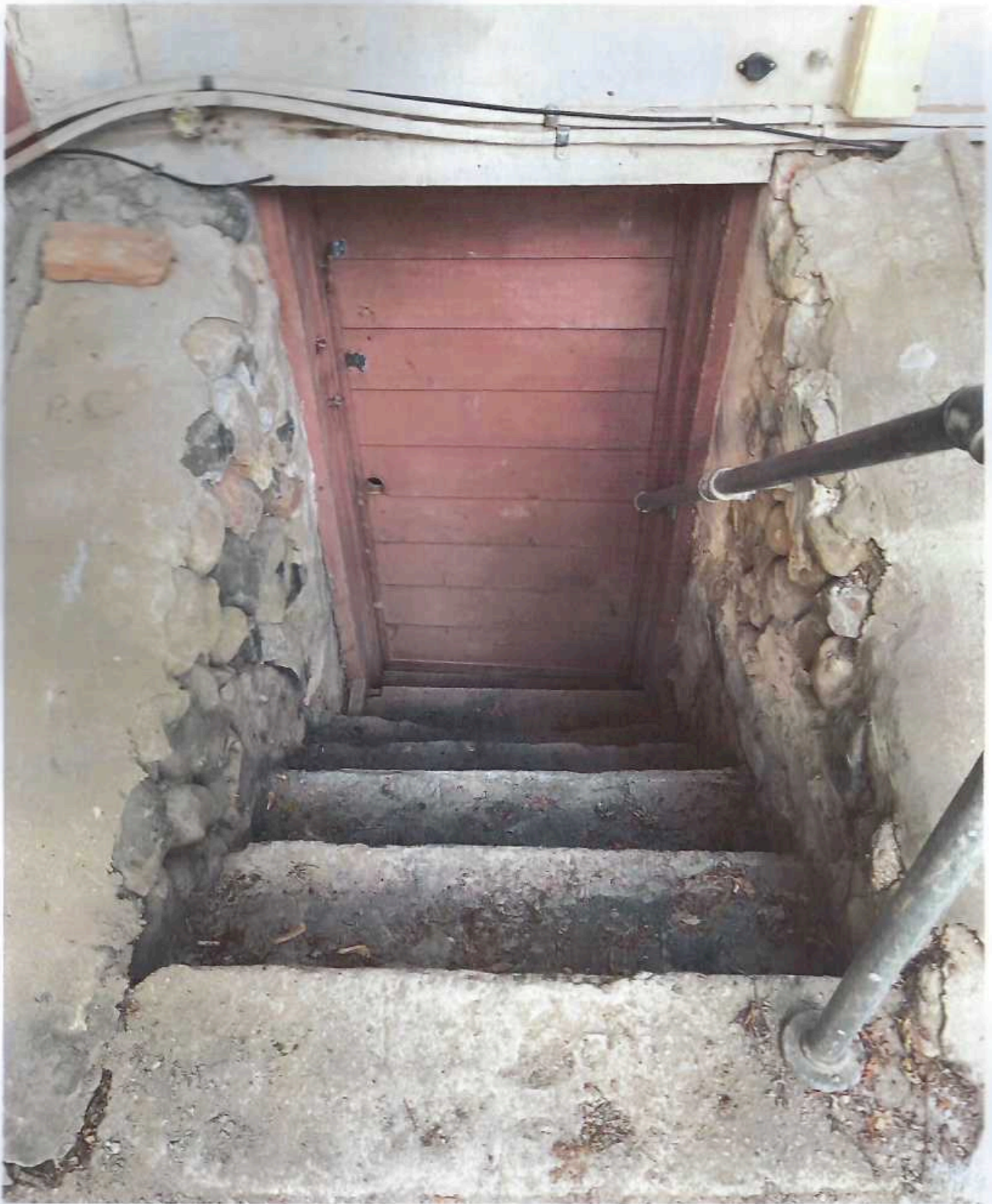
627 N RIVER, DOOR TO BASEMENT, EXISTING CONDITION. JUNE 2023
