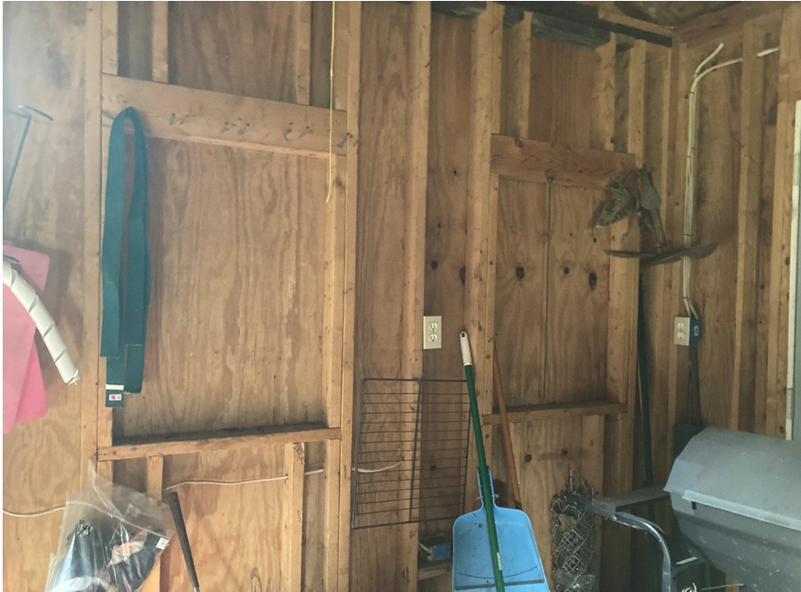
309 N Park, east wall from inside the building, existing framing for windows shown.
