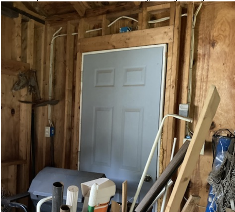
309 N Park, garage, door in south wall near the southeast corner will become a window.
