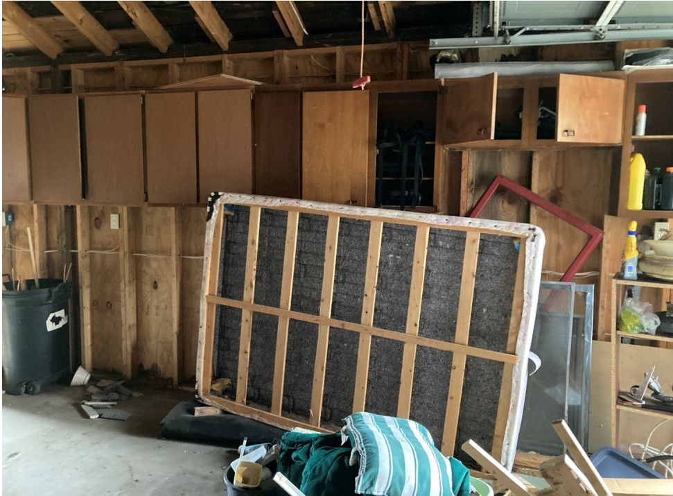
309 N Park, garage, north wall from inside. These cabinets will be removed and three windows will be installed on this wall—two will be small fixed rectangular windows and one will be a double-hung.
