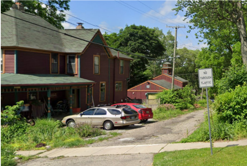
309 N Park, garage. Despite the cupola, garage is not a historic outbuilding. It was rebuilt in the 1980s or 1990s.
