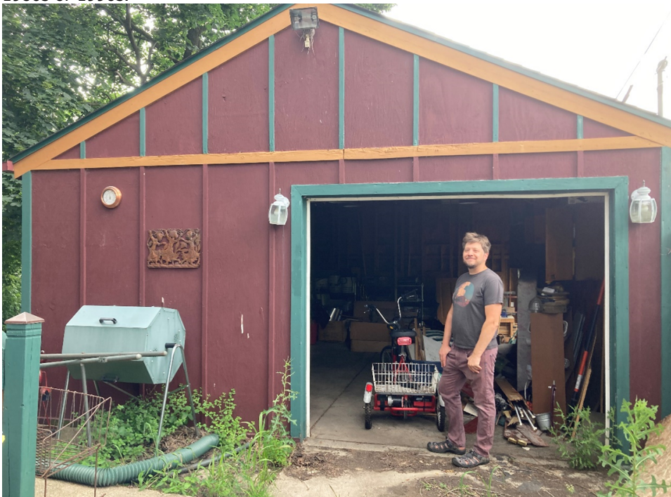
309 N Park garage, east elevation, large doorway will hold the patio doors, and to the left will be two windows installed in existing framing.
