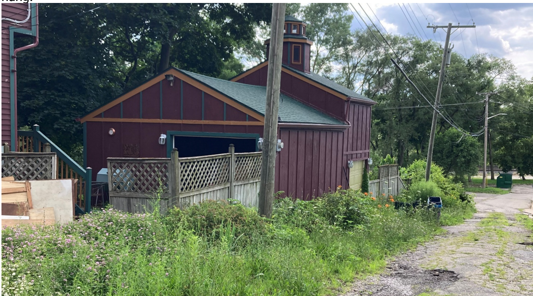
309 N Park, garage, north wall along the alley where three windows will be installed, and the east wall (front) where the patio doors and two windows will be installed.
