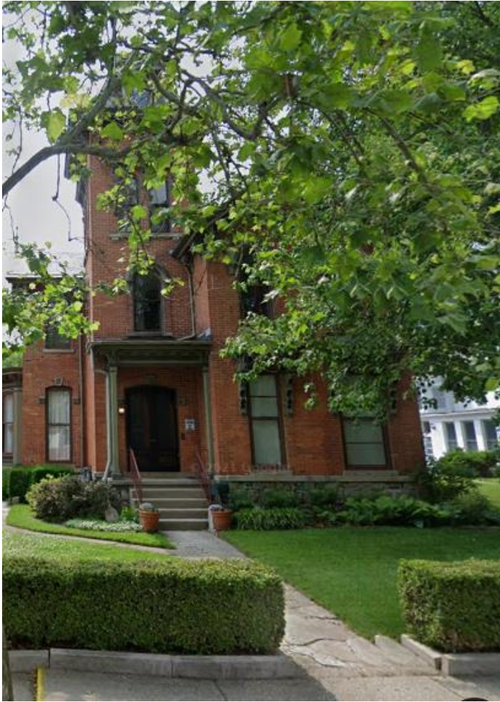
121 N Huron, June 2021. Windows being discussed are on rear of house. See attached.
