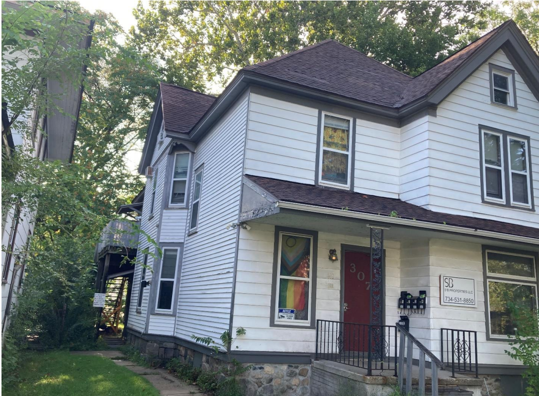
307 N Hamilton, August 2023, south side where gutter and downspout will be added.
