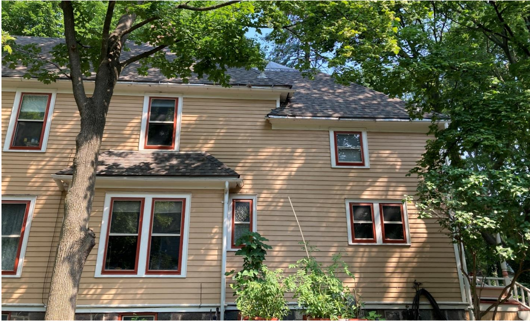
316 N Grove, August 2023, south side of house. Second-floor flat roof shown just to the right/east of the roofed first-floor windows, and the skylight installation is visible on the flat roof.
