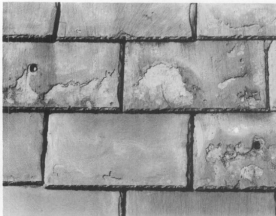
This detail shows slate delamination caused by a combination of weathering and pollution. In addition, the slates have eroded around the repair nails, incorrectly placed in the exposed surface of the slates. (Lower Pontalba Building, New Orleans, photo courtesy of Building Conservation Technology, Inc.)
