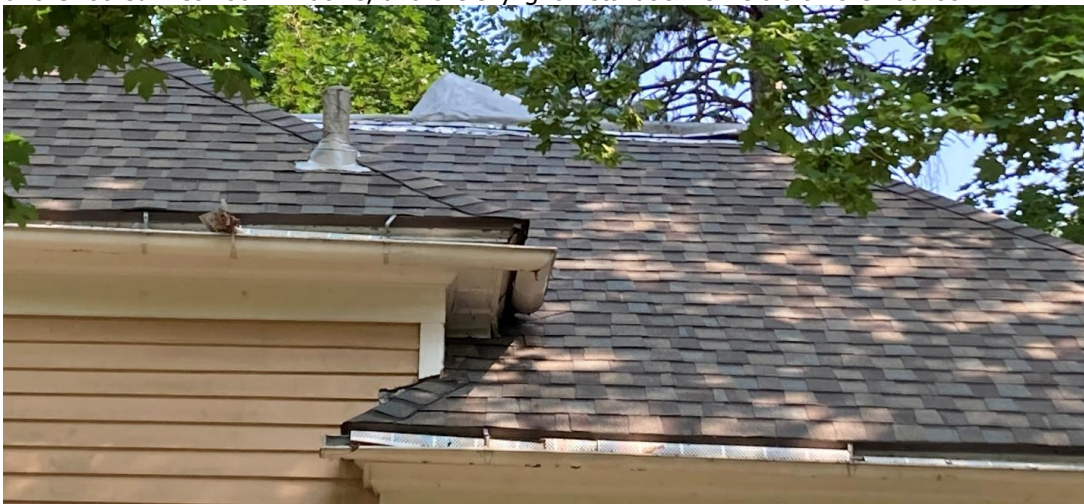
316 N Grove, August 2023, south side of house, detail of second-floor flat roof and the skylight installation.
