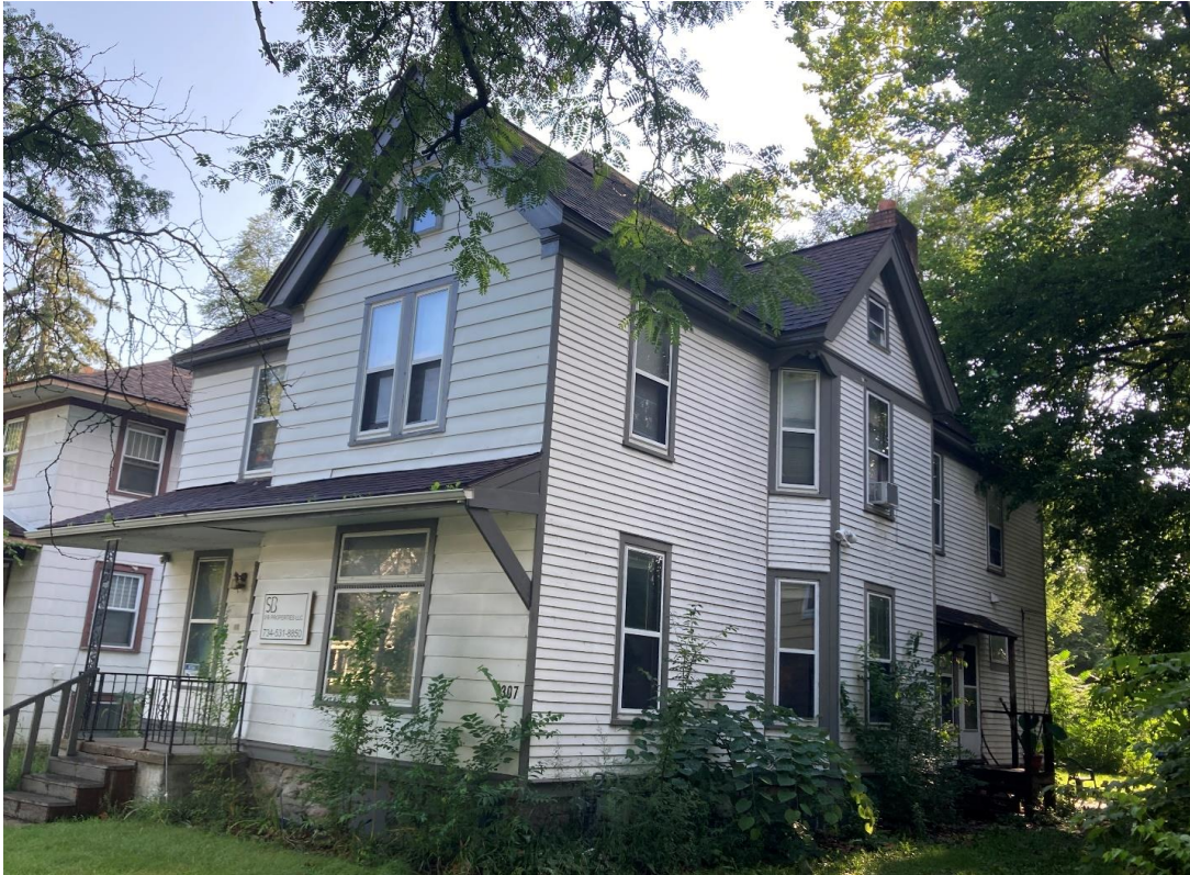
307 N Hamilton, August 2023, north side showing north chimney and the spot where the downspout near the northeast corner will be extended.
