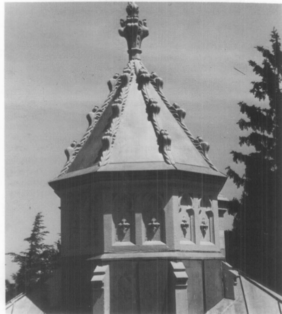
Decorative features such as cupolas require extra maintenance. The flashing is carefully detailed to promote run-off, and the wooden ribbing must be kept well-painted. This roof surface, which was originally tin plate, has been replaced with lead-coated copper for maintenance purposes. (Lyndhurst, Tarrytown, New York, photo courtesy of the National Trust for Historic Preservation)
