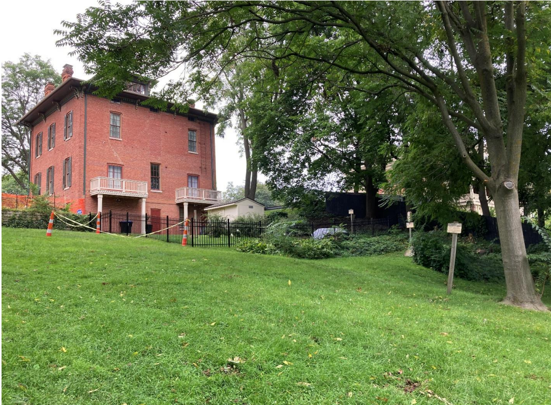
Looking northwest, privacy fence visible, erected by next door neighbor at 206 N Huron. It is this fence that the fence site plan mentions "tying into."
