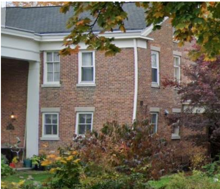
206 S Washington, northwest corner, two windows on second floor are vinyl one-over-ones. (Google Streetview, October 2020) These are the windows proposed to be replaced.
