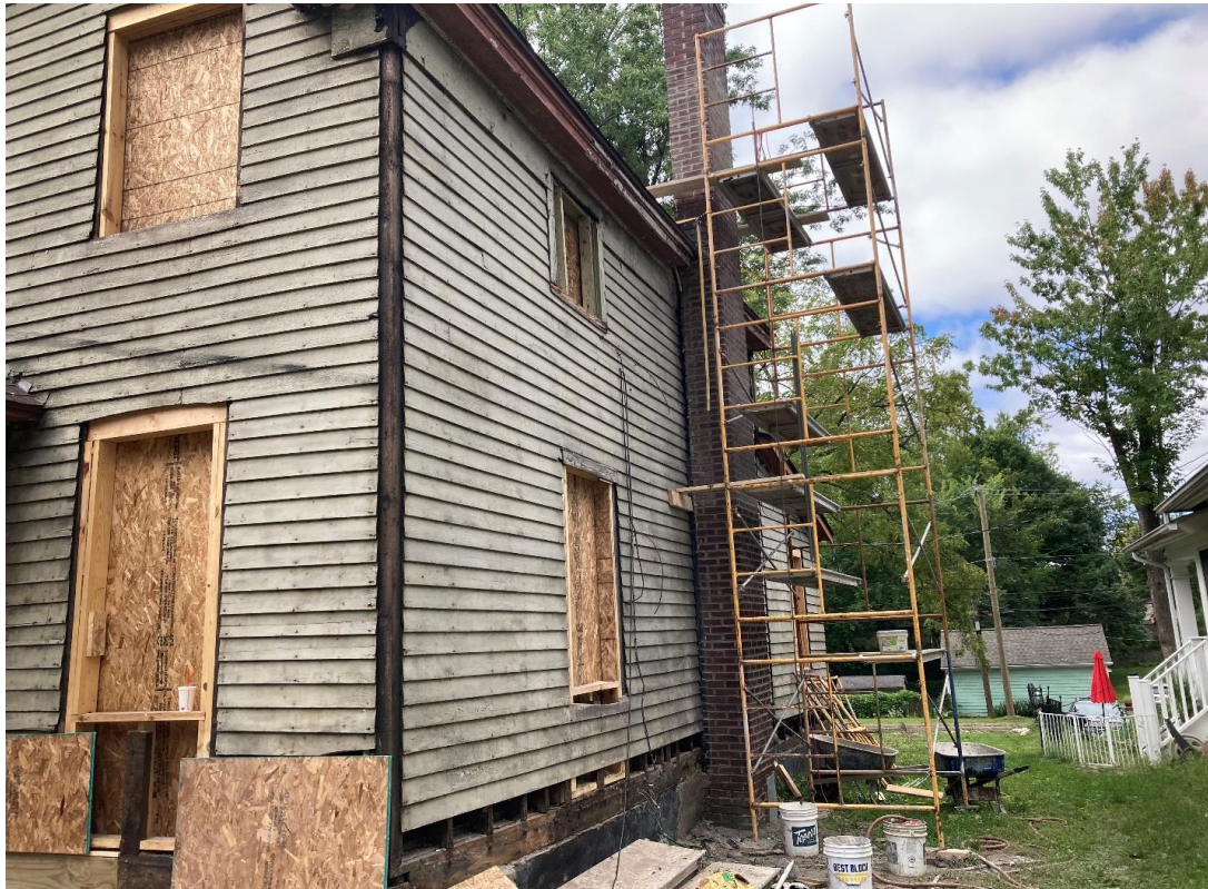
627 N River, Sept 2023. The character-defining frieze board visible here should be preserved or replicated, and the windows that are within that frieze board should be kept in that size and location as they were historically.
