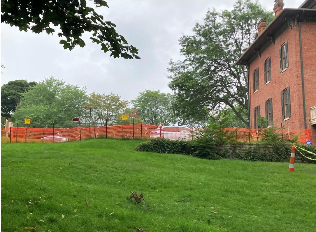
Detail of parking area next to 130 N Huron.
