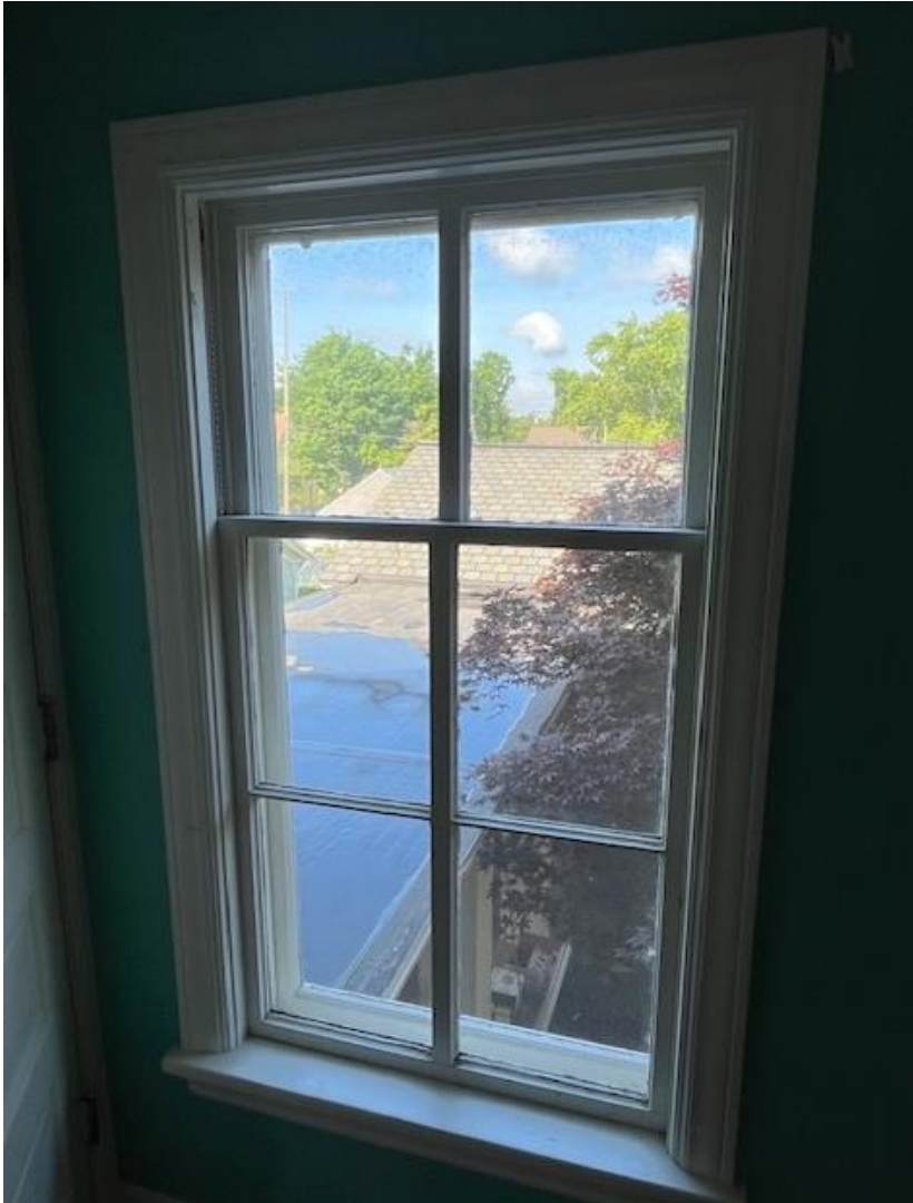
206 S Washington, historic window that will be replicated, provided by window contractor, September 2023.
