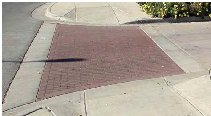
Figure 27: Driveway Apron Example
