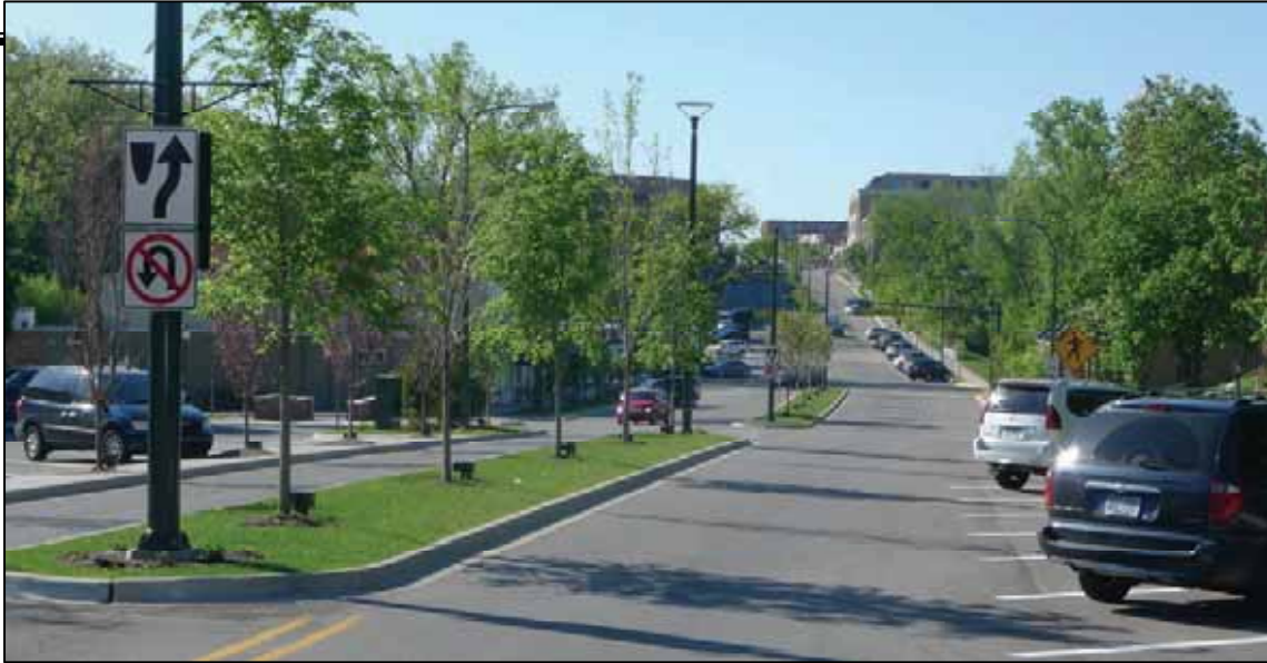
The city recently narrowed Old Woodward Avenue from a five-lane highway into a two lane street by installing a landscaped median and adding diagonal parking, as illustrated in the plan. Similar traffic-calming improvements have been installed along Ring Road downtown.
