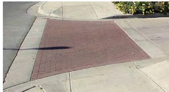
Figure 27: Driveway Apron Example
