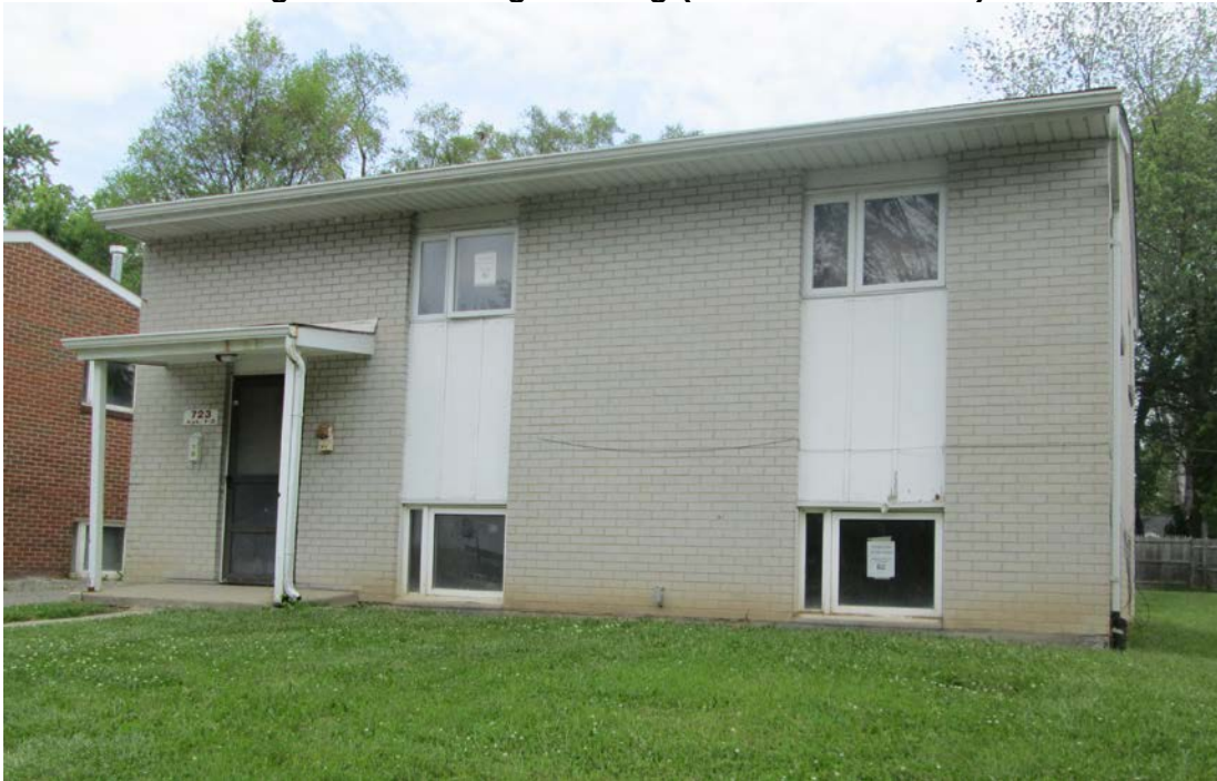
Figure 4: Existing building (to be demolished)
