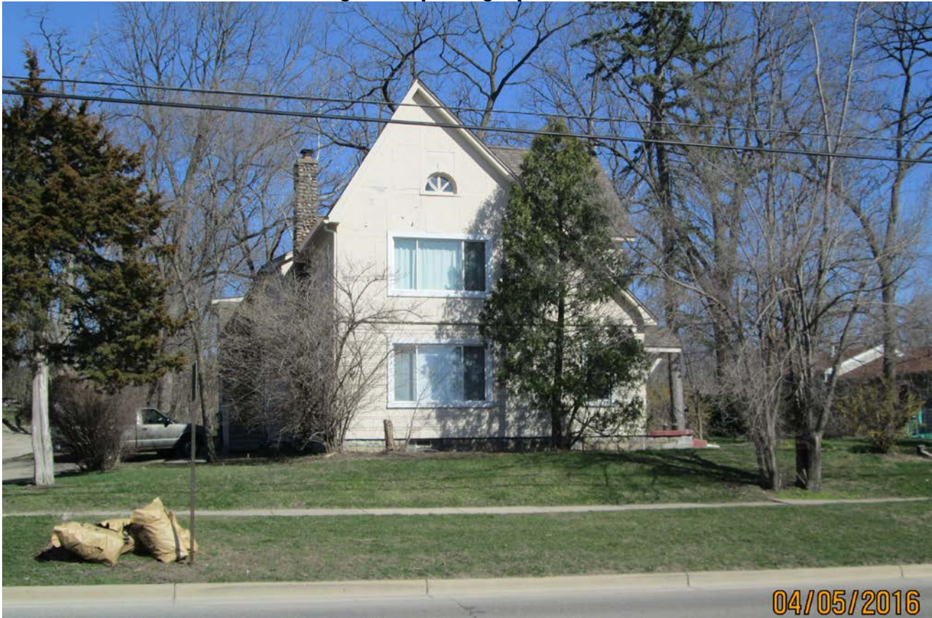
Figure 3: photograph of site
