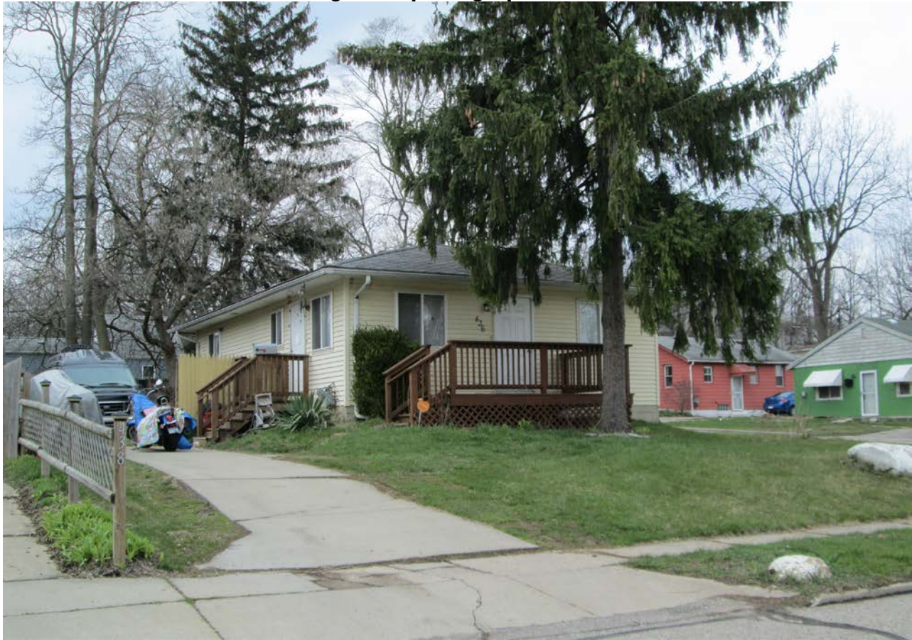
Figure 3: photograph of site
