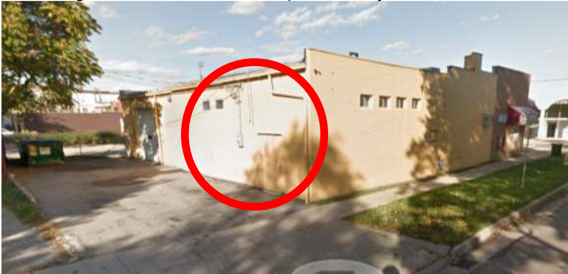
Figure 3:View from South-west; location of potential entrance
