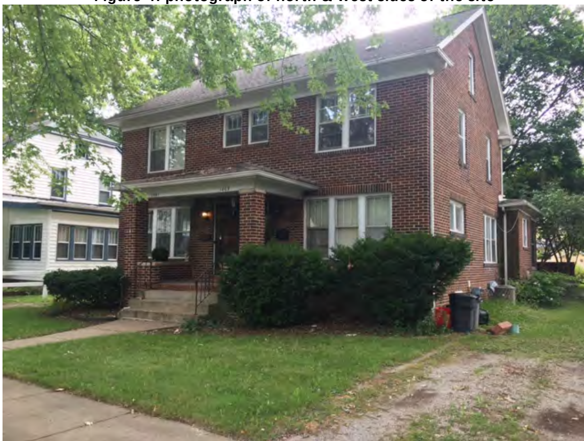
Figure 4: photograph of north & west sides of the site
