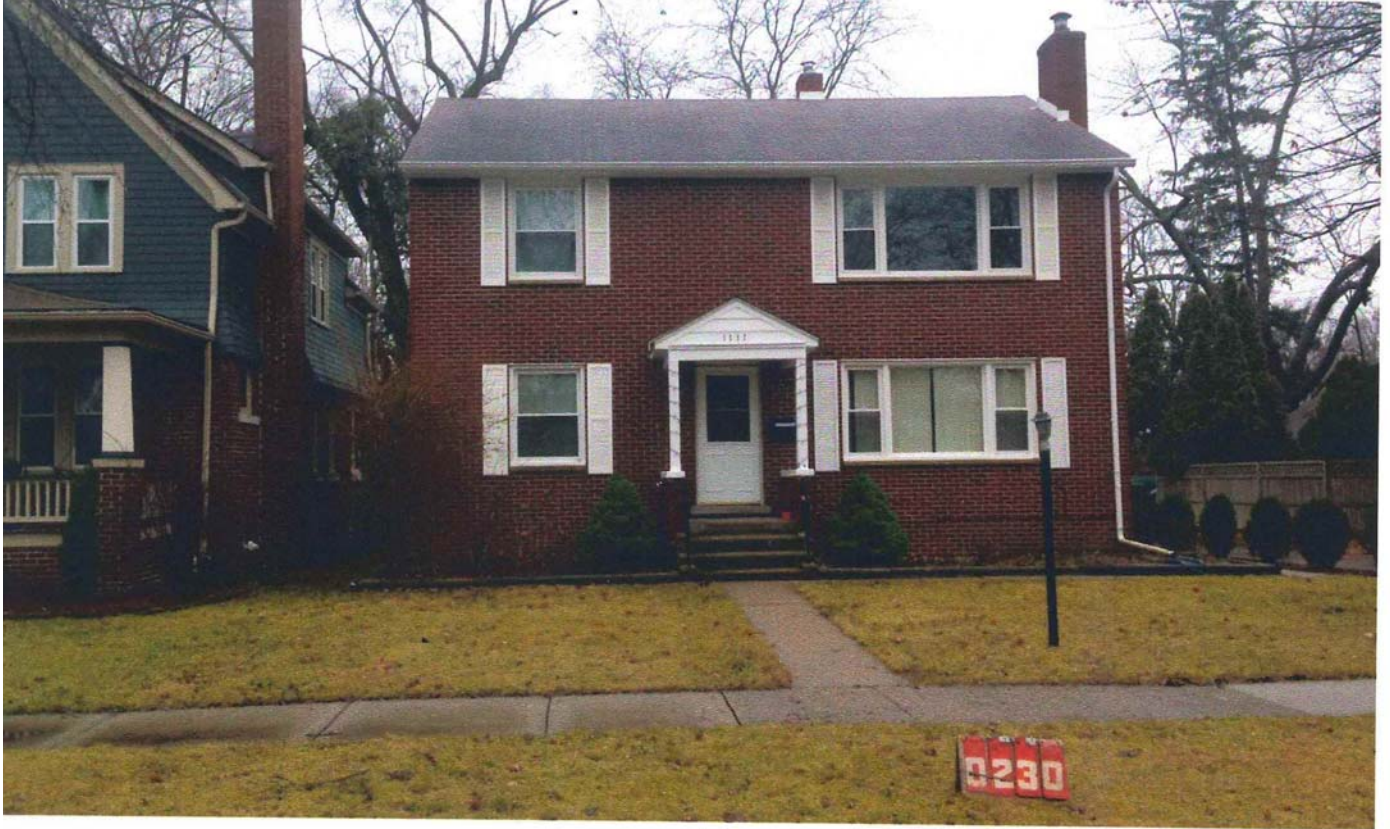
Figure 4: photograph of front/north side
