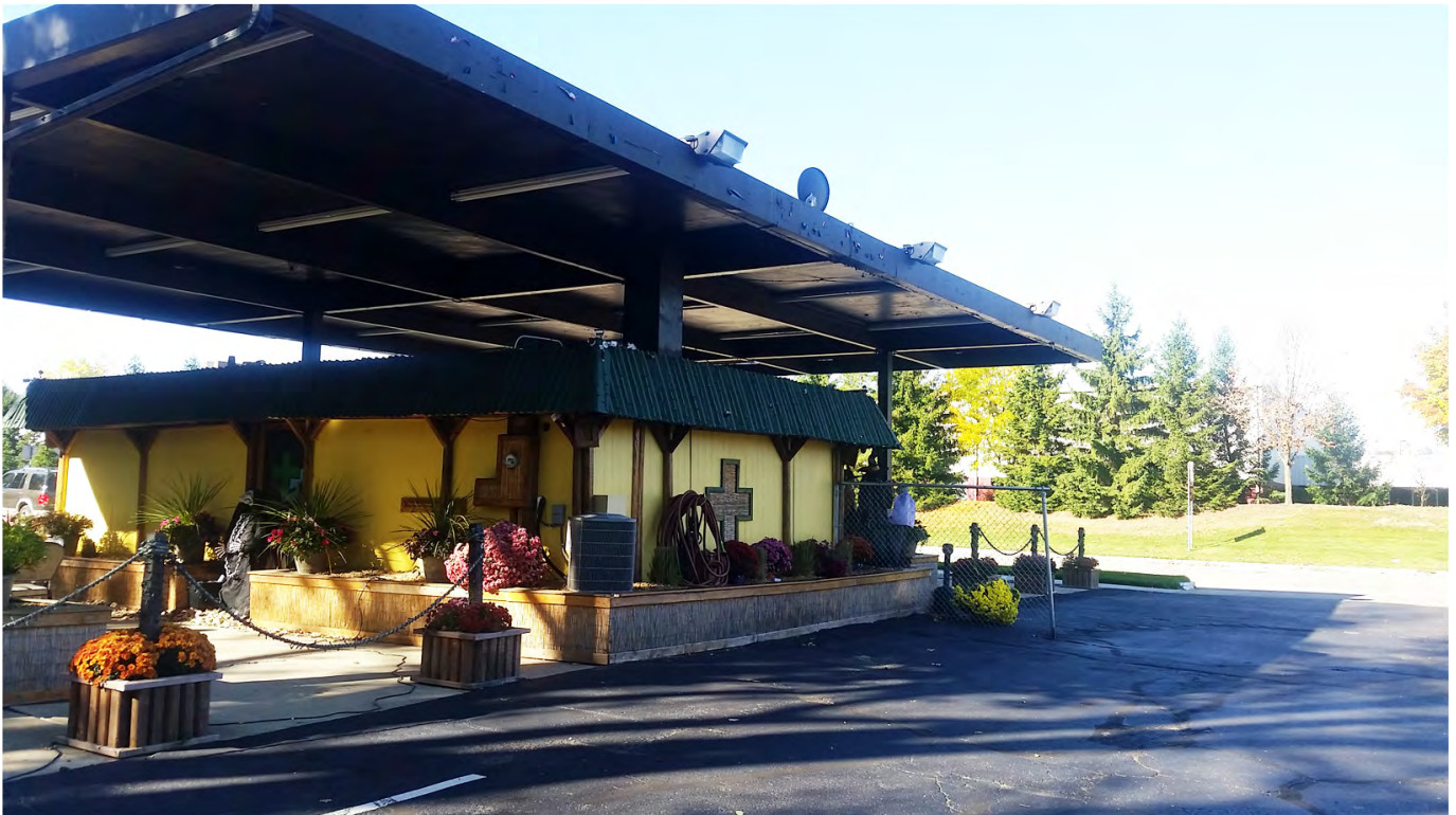
11. NORTH AND EAST SIDES OF BUILDING.
