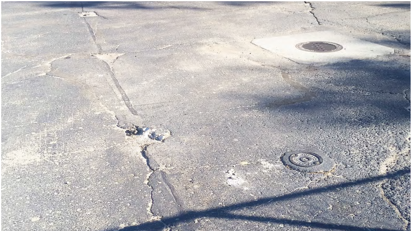
13.-14. TYPICAL "AMOCO TEST WELL" COVERS.
