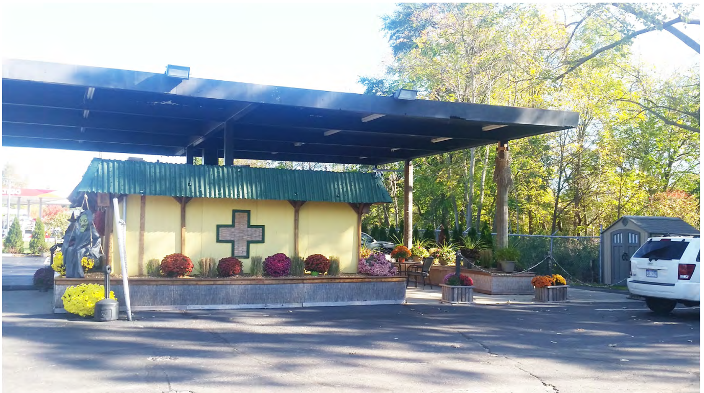
9.-10. SOUTH SIDE OF BUILDING.
