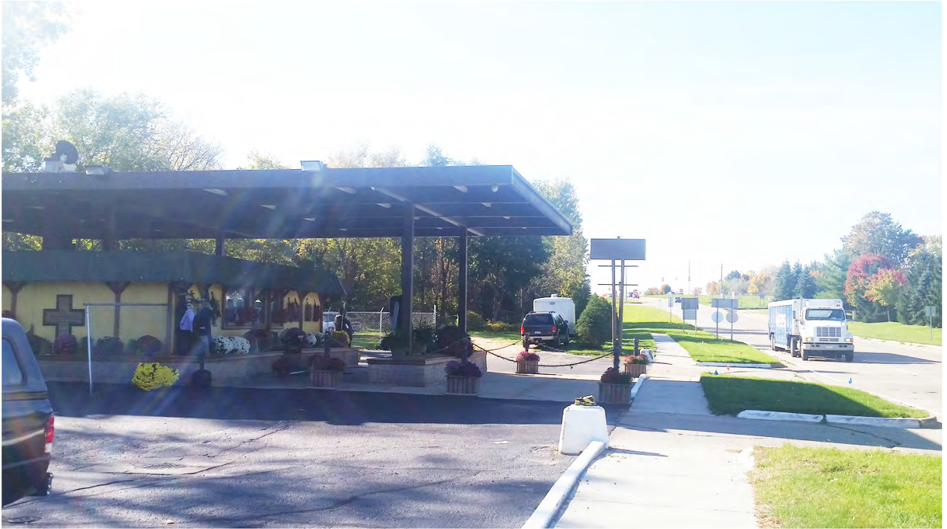
3. NEAR THE NORTHWEST CORNER, LOOKING SOUTH.
